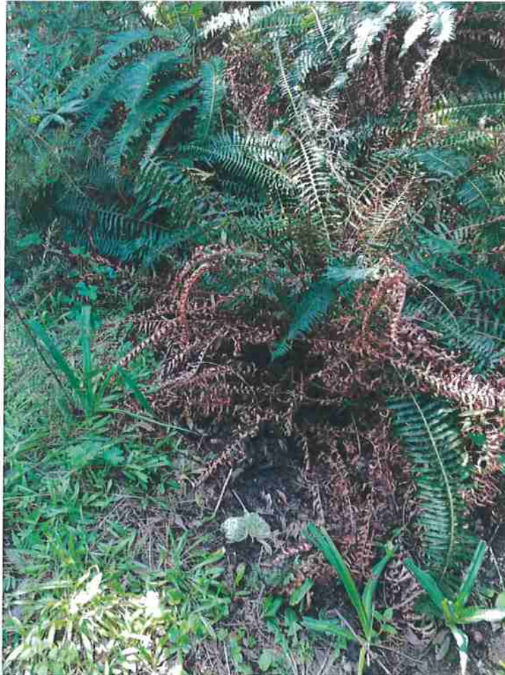
Photo 12. Stream Crossing #5, view of stream channel entering culvert inlet. Culvert is properly aligned with the natural grade of the stream channel.
