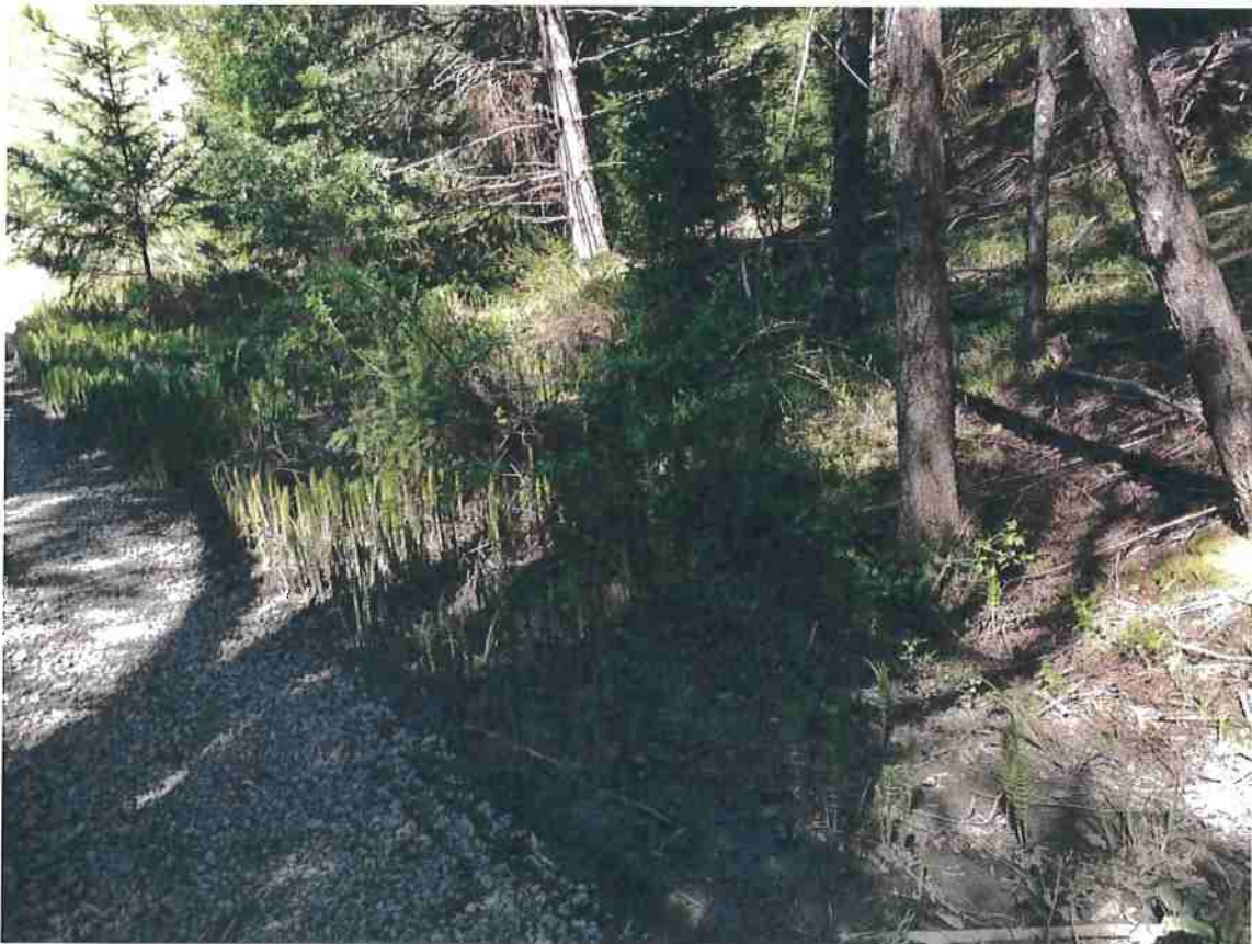
Photo 15. Stream Crossing #7, upslope view of springy area above inlet.
