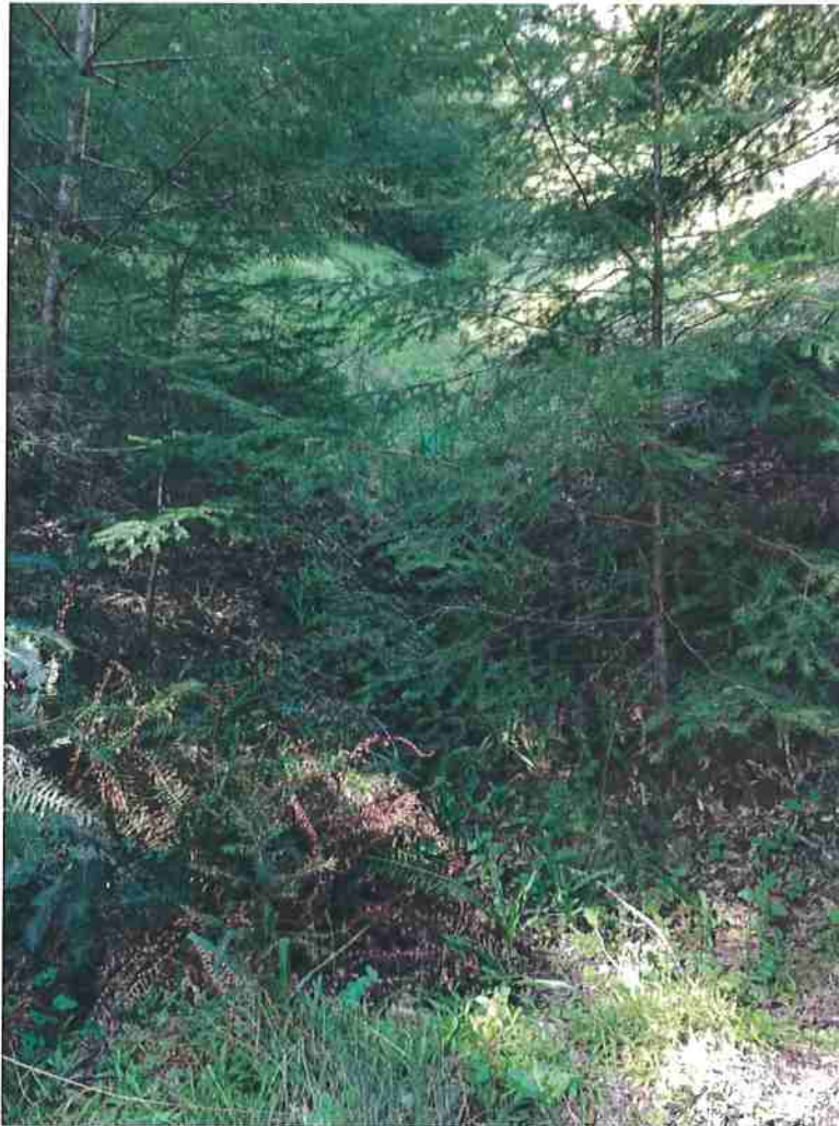
Photo 11. Stream Crossing #5, upstream view of channel of Class III watercourse leading to culvert inlet.
