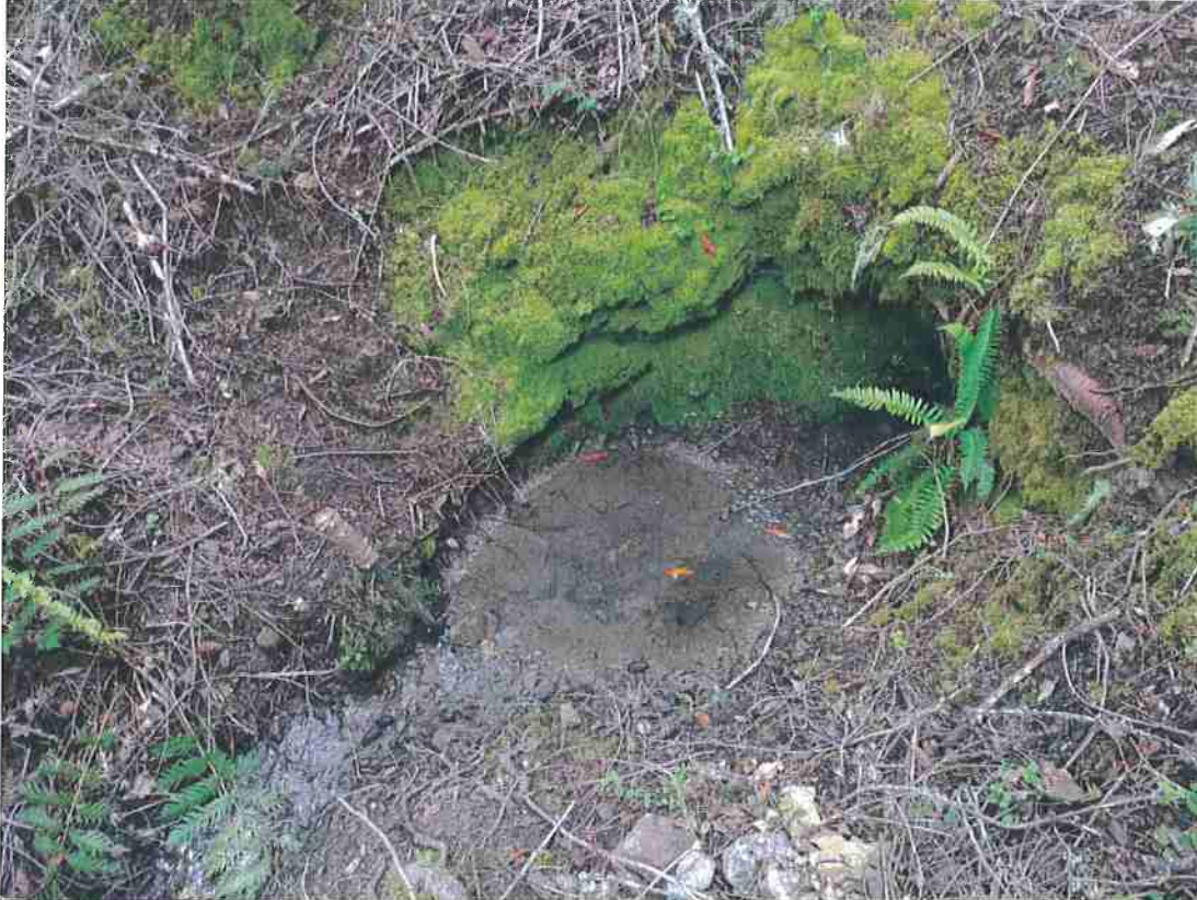
Photo 26. POD #3, photo of inlet of Point of Diversion #3, and diversion site. Diversion structure is standing out of the water for photo. Small mesh screen is zip-tied over metal screened intake, which is secured to a 3/4" diameter polyline. Water is gravity fed down to holding tanks.
