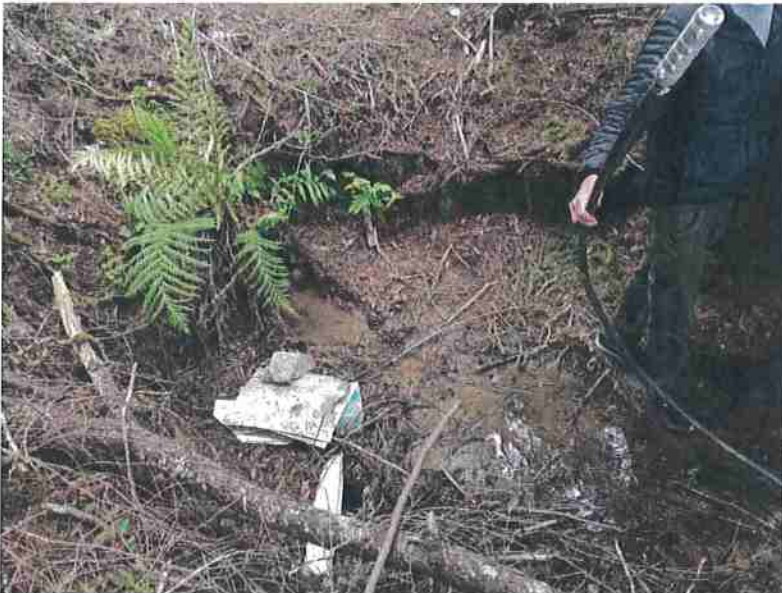
Photo 25. POD #2, photo of inlet of Point of Diversion #2. Small mesh screen is zip-tied over metal screened intake, which is secured to a 3/4" diameter polyline. Water is gravity fed down to holding tanks.
