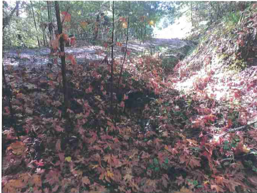
Photo 5. Stream Crossing #3, view of 24-inch diameter culvert inlet.
