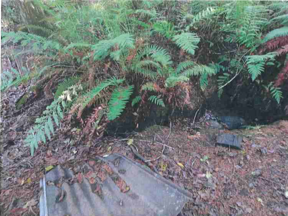
Photo 31. Pond #4 (Guerrilla Pond #2)- A previous occupant of this property excavated a small containment basin below a natural spring, lined it with a liner of unknown materials and attempted to concrete the embankments. In an attempt to camouflage the pond, it was covered it with sheet metal and vegetation. It was recently discovered by the applicants, who intend to decommission it.
