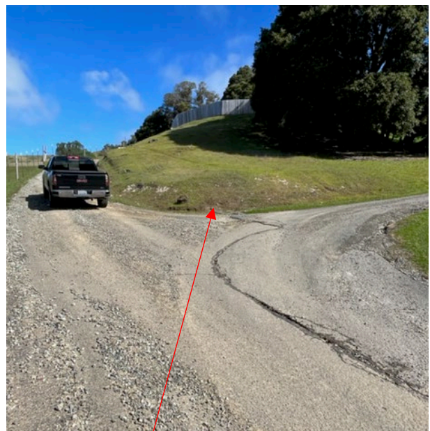
Approximate location of culvert inlet
