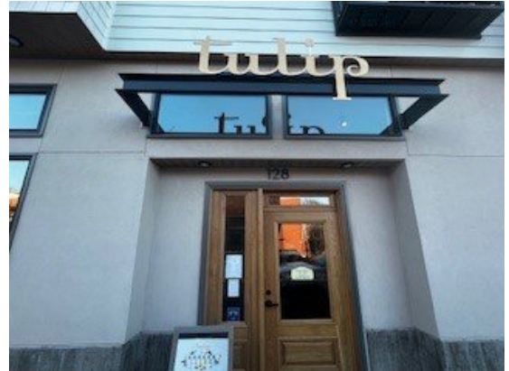
Figure 6: Street view of Tenant C canopy sign (C1) (Tulip) installed without a permit, taken March 07, 2024
