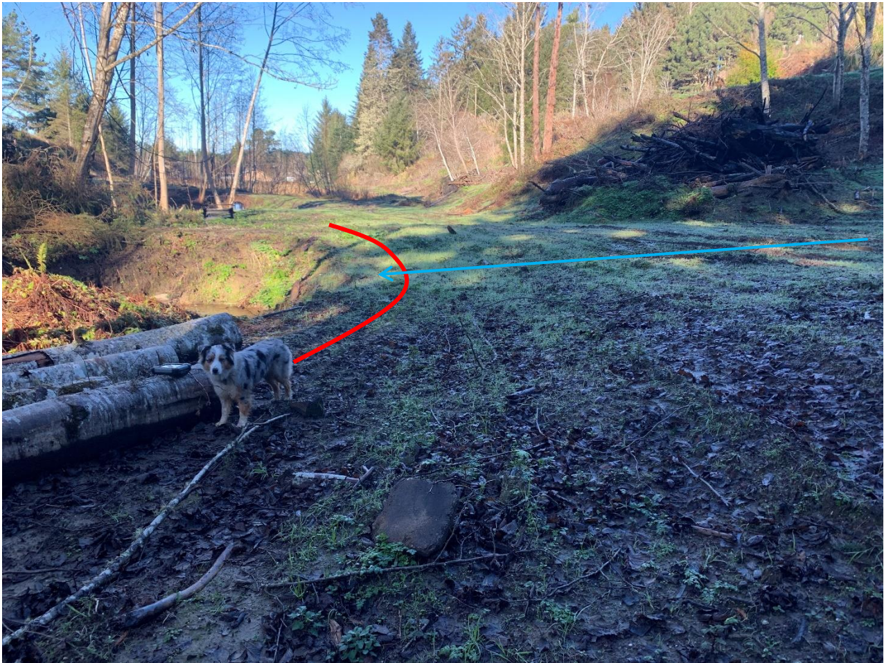
Photo #4: Concentrated surface runoff entering Willow Brook from the northside of the stream highlighted in blue. The landowner shall place straw waddles at the area highlighted in red.
