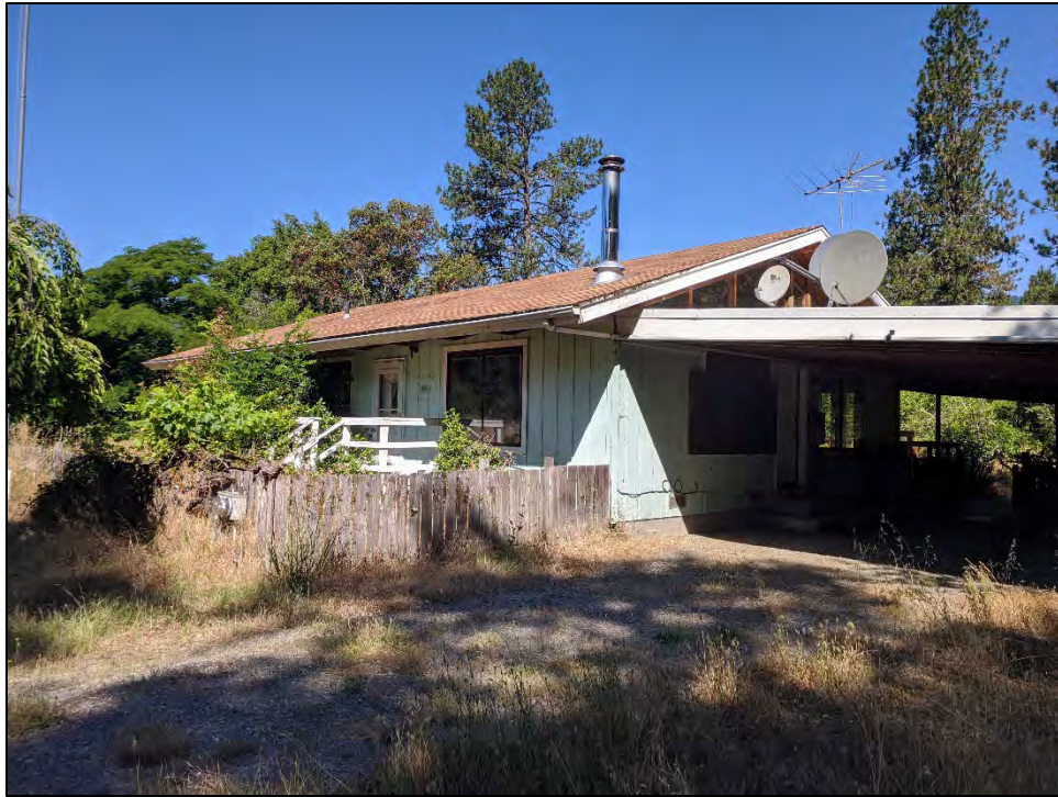
Photo 5: View of the abandoned single-family residence. June 27, 2022.
