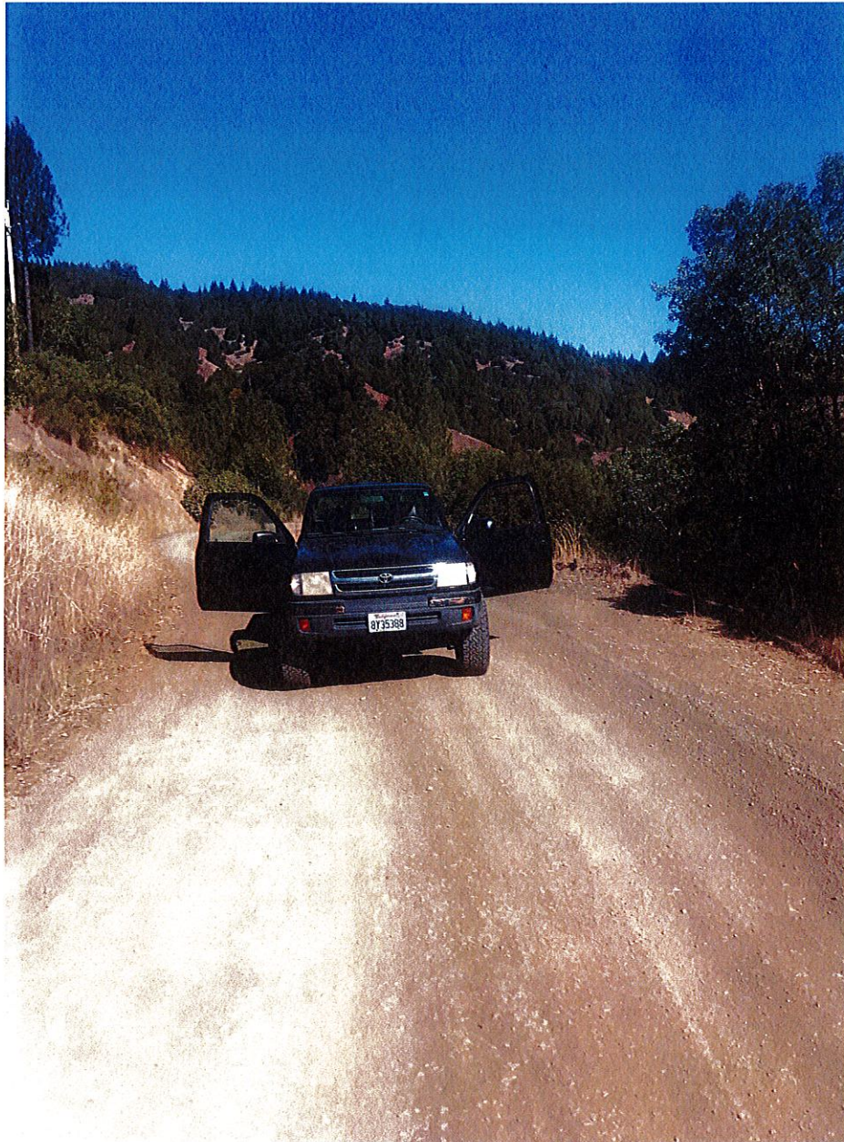
Figure 9: RP-9. Road width: 16' 14" with 7' 6" turnout.
