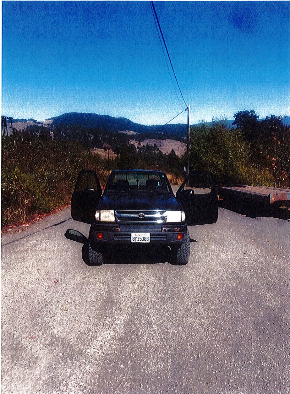
Figure 19: RP-19. Intersection of Bell Springs Rd. and Harris Rd. Harris Rd. is paved for approximately 150 feet from the intersection of Bell Springs Rd. Road width: 23' 9".
