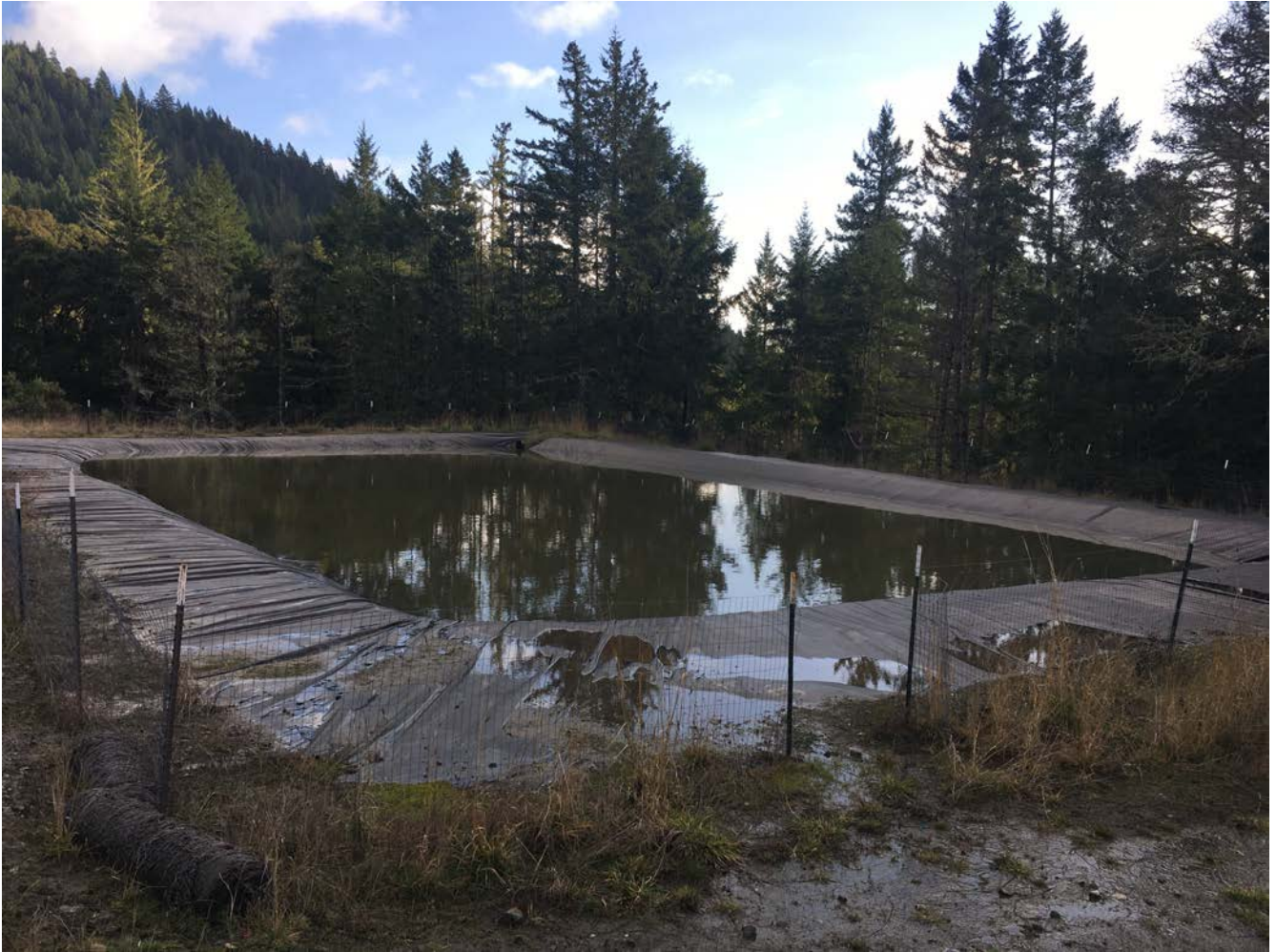
Rainwater catchment pond point of collection.
