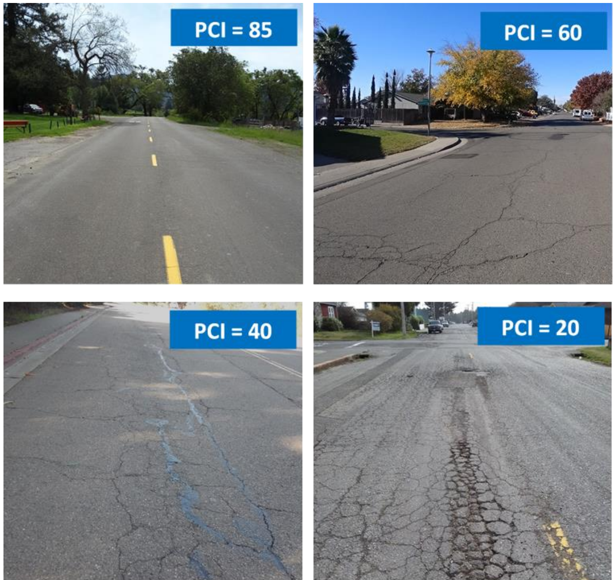
Figure 1. Examples of Roads with Different PCIs
