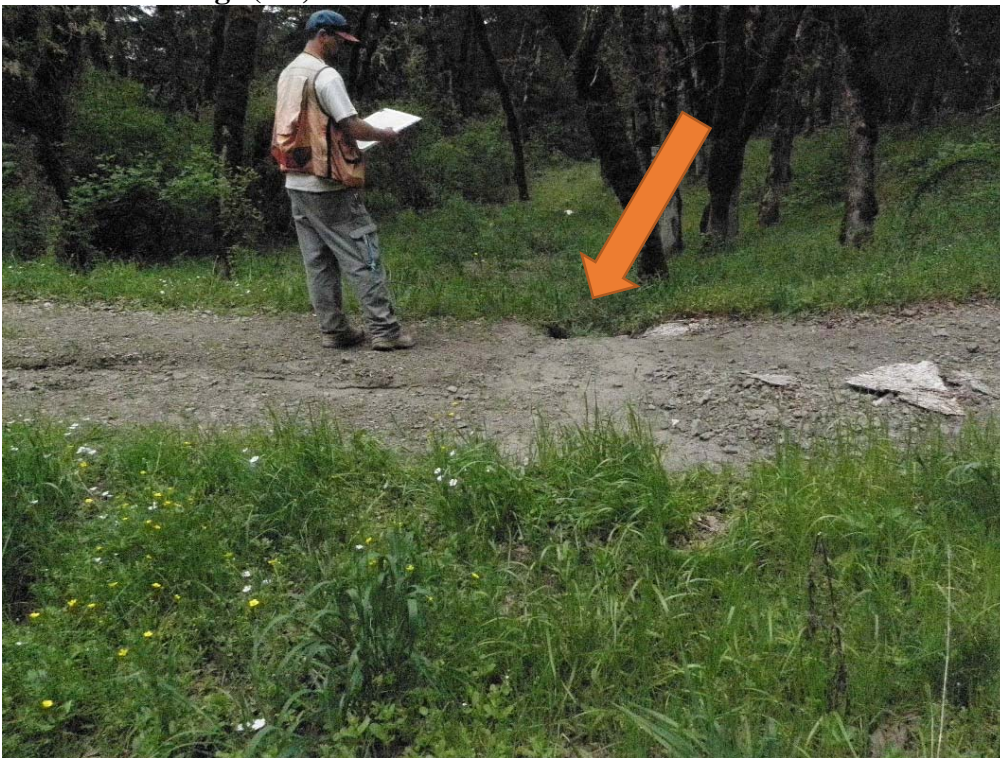
Photo 4 - Stream crossing of stream crossing in the road bed in a fill crossing on the watercourse. It is no formal drainage structure. Note the small lead pit at the offboard road. Photo April 2011
