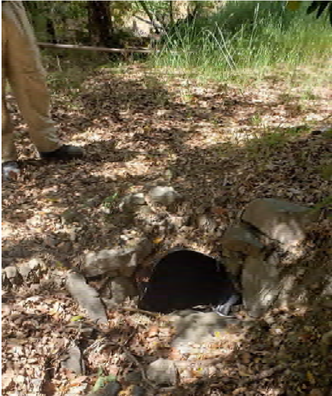
Inlet of Site 19
