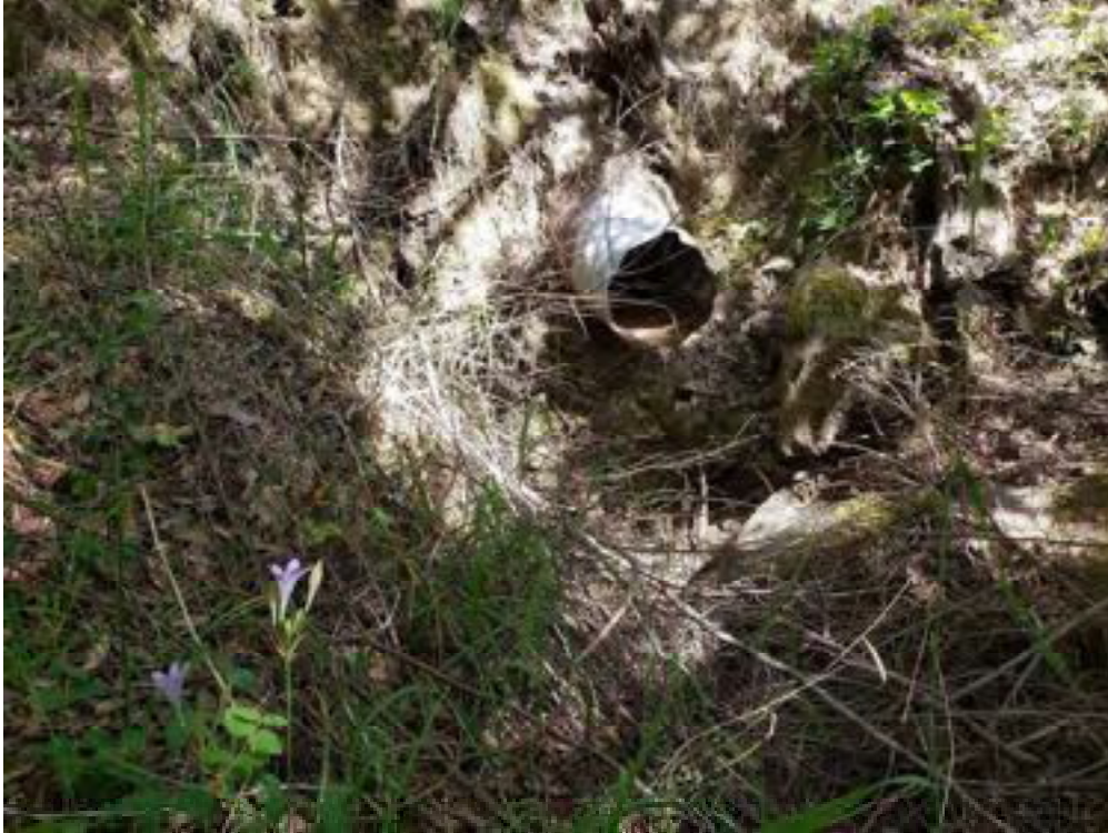
Site 05. Looking at the outlet.
