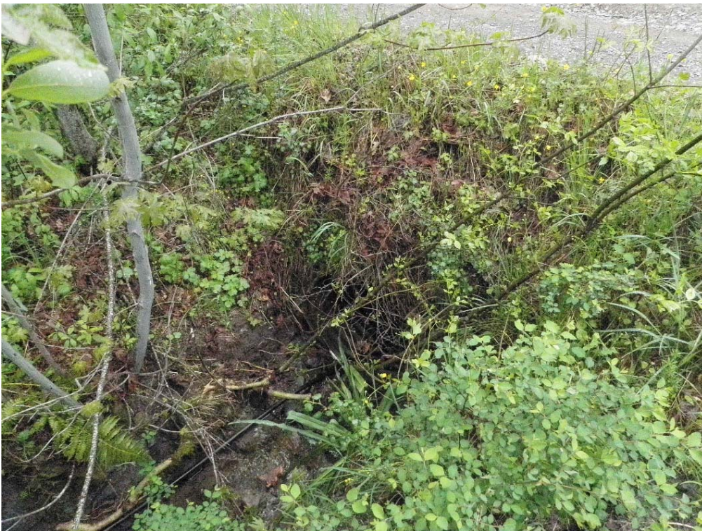
Photo 8- View of 2' long 12" diameter culvert inlet on Waterloo watercourse. Photo April 2011
