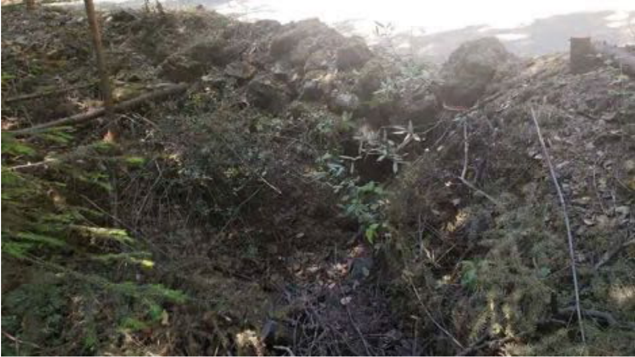
Site 26. Outlet of the watercourse crossing.
