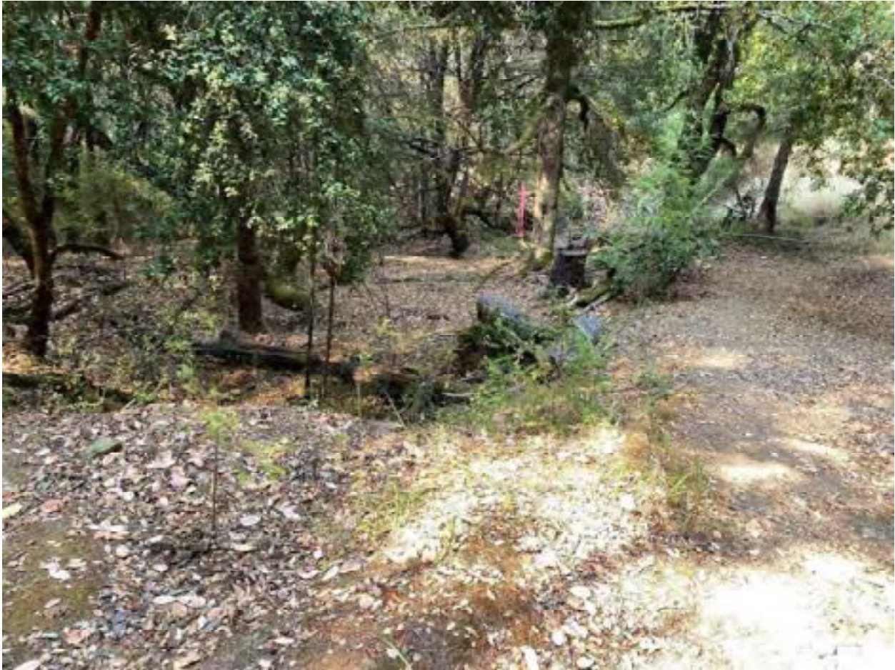
Photo 57: Stream Crossing 19. Looking downstream from the road. The pink flag indicates where the native stream channel is and where the stream will be realigned to once stream crossing 19 is decommissioned. Photo date 9-1-2021.
