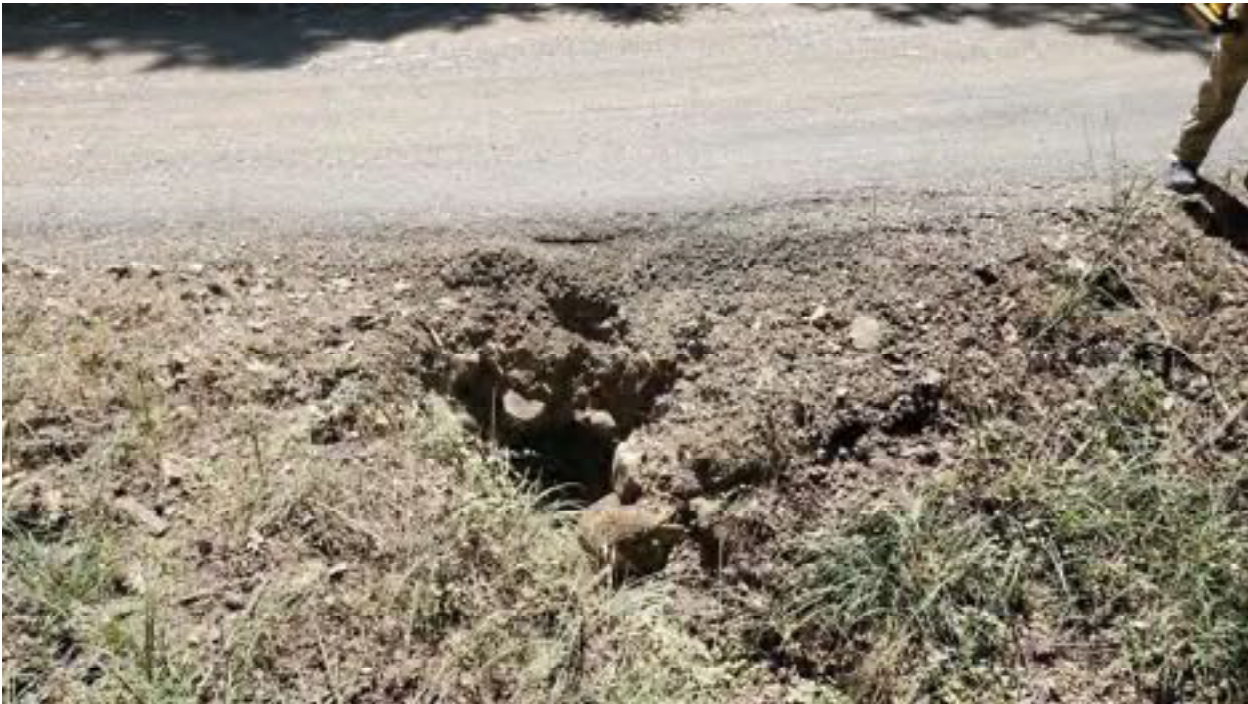
Site 26. Inlet of the watercourse crossing.
