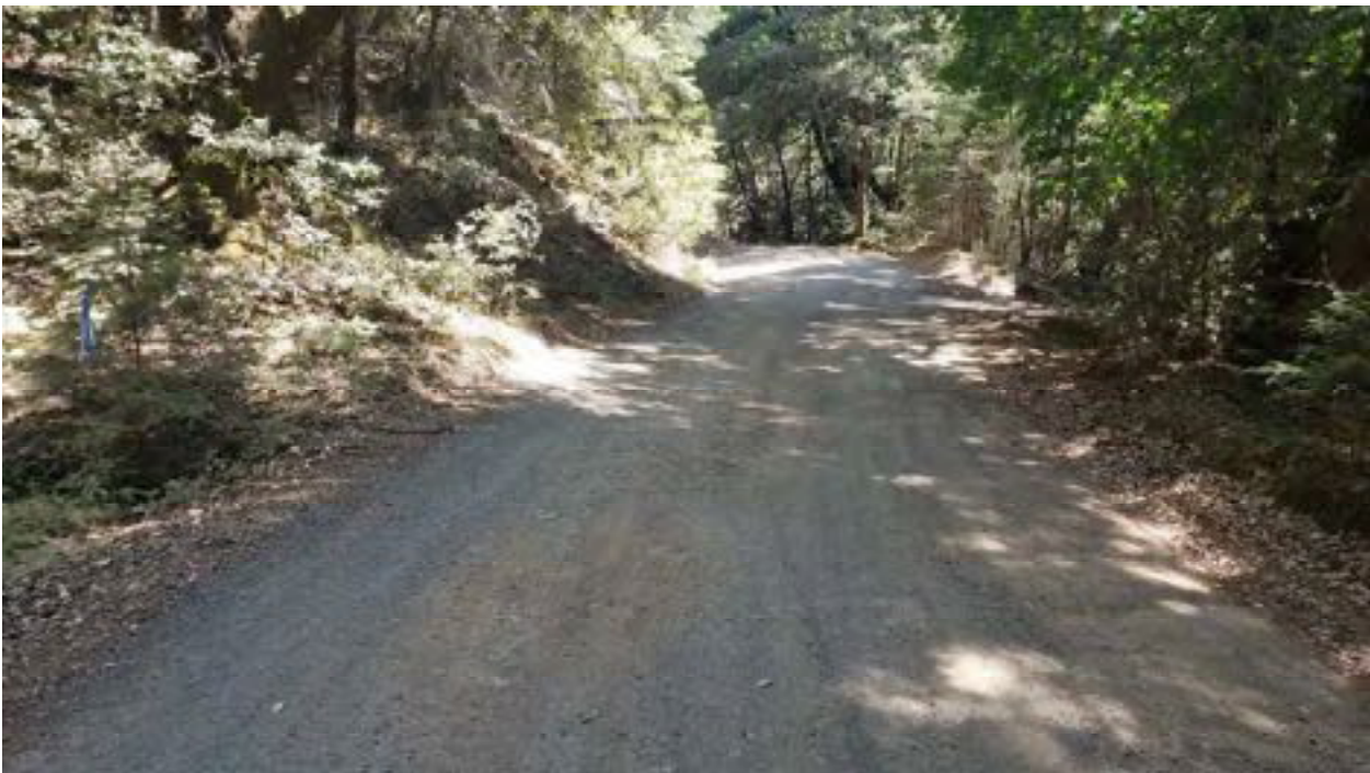
Site 24. Looking down grade.
