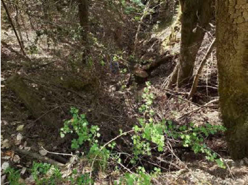
Site 06. Looking down channel from the outlet. The upgraded culvert will outlet approximately where the blue flagging is hanging.
