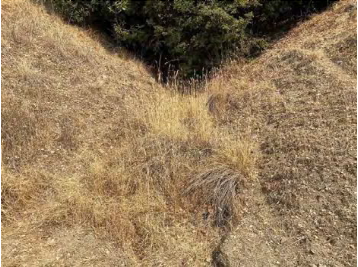
Photo 7: Stream Crossing 03. Looking upstream from the inlet of the 8-inch diameter culvert at stream crossing 03. Photo date 9-1-2021.
