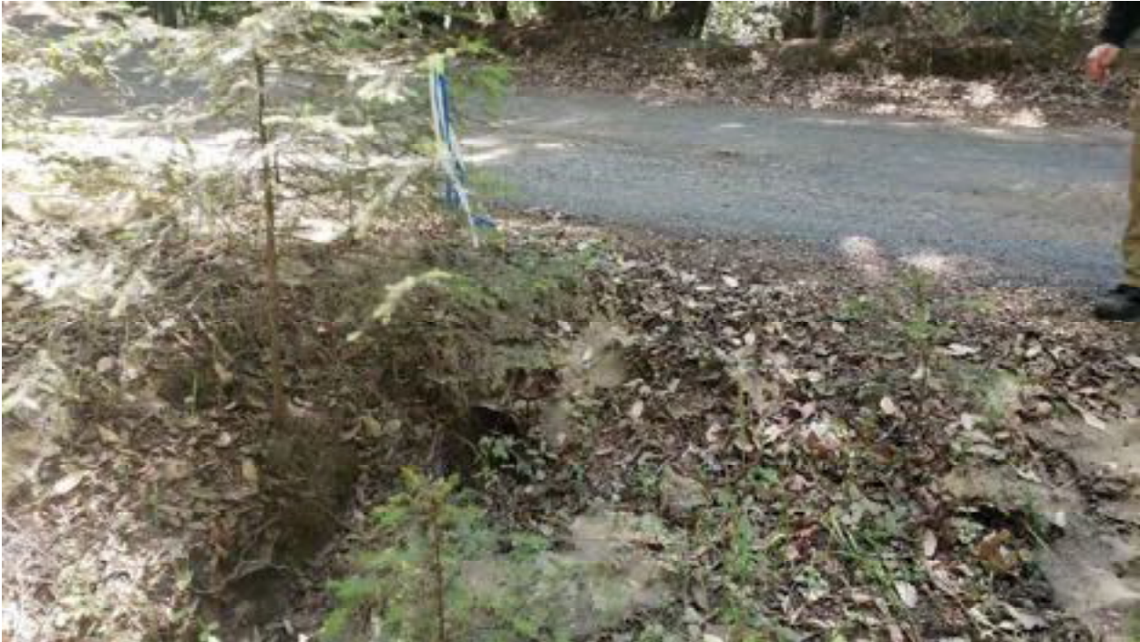
Site 24. Inlet of the watercourse crossing.
