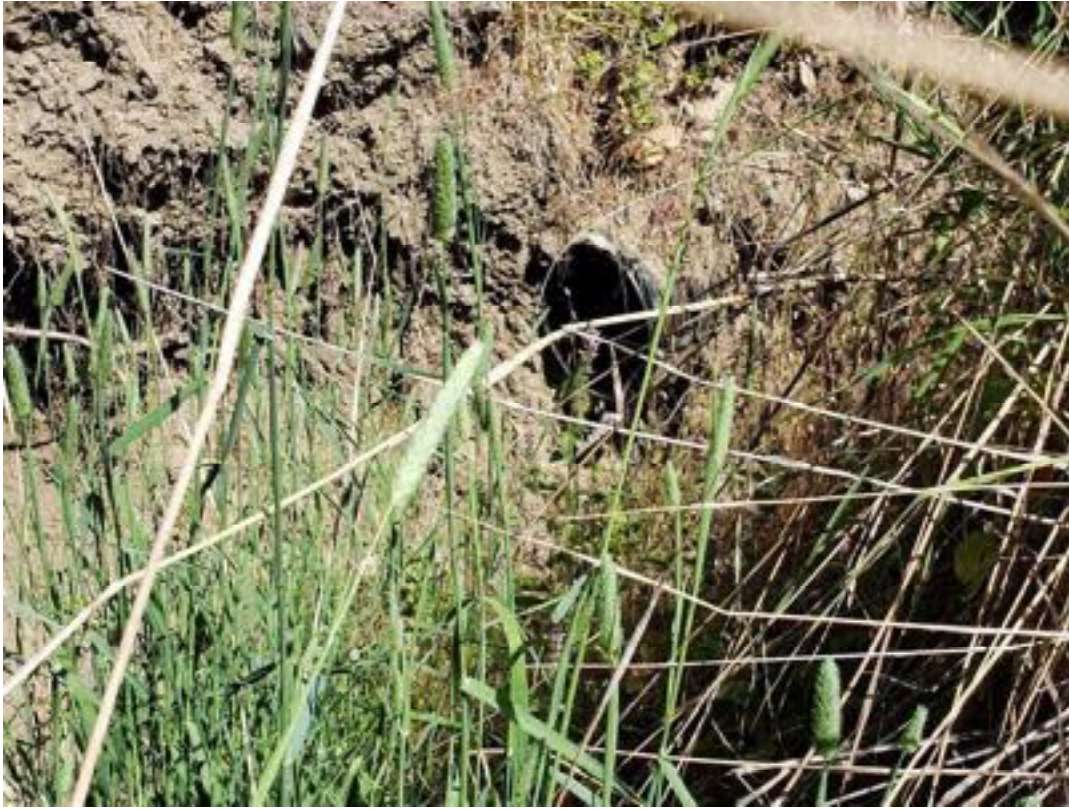
Site 04. Looking at the outlet.
