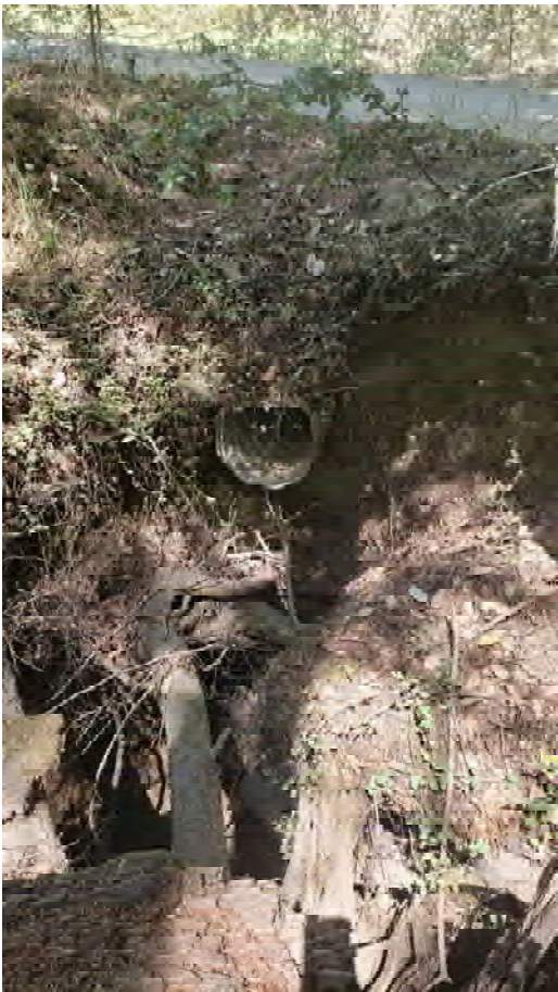
Site 24. Outlet of the watercourse crossing.
