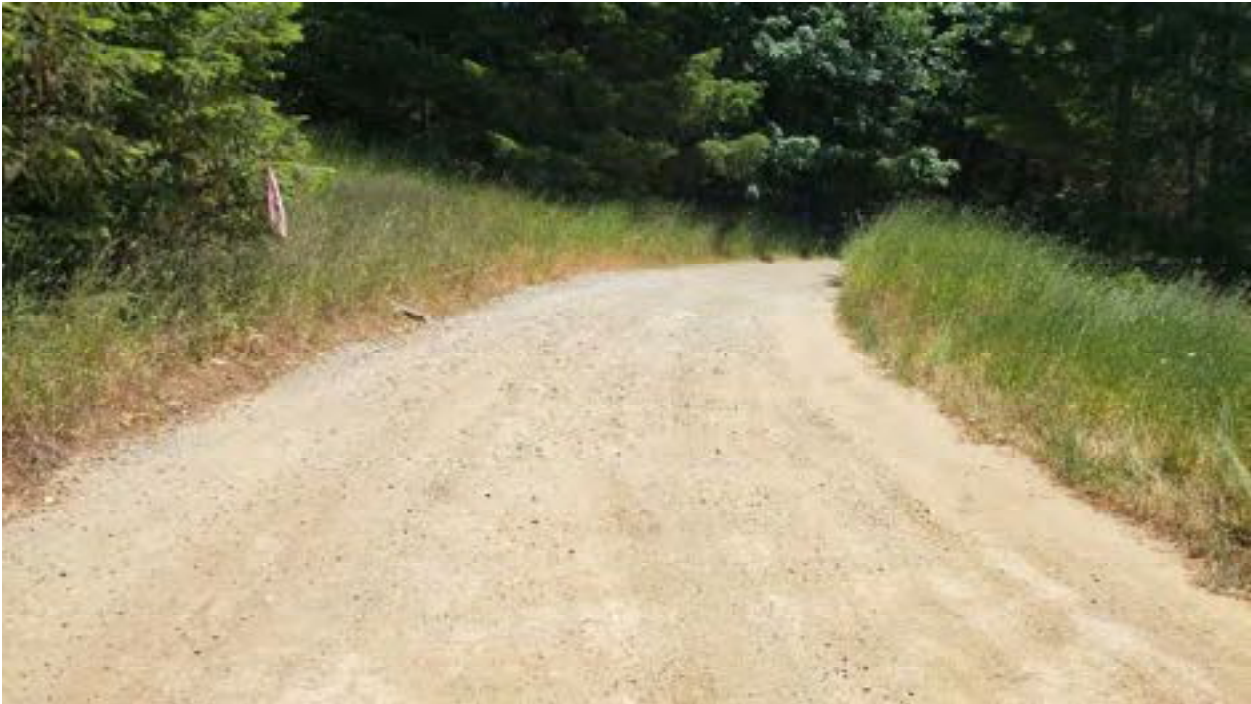
Site 12. Hydrologic disconnect for Sites 13, 14, and 23.
