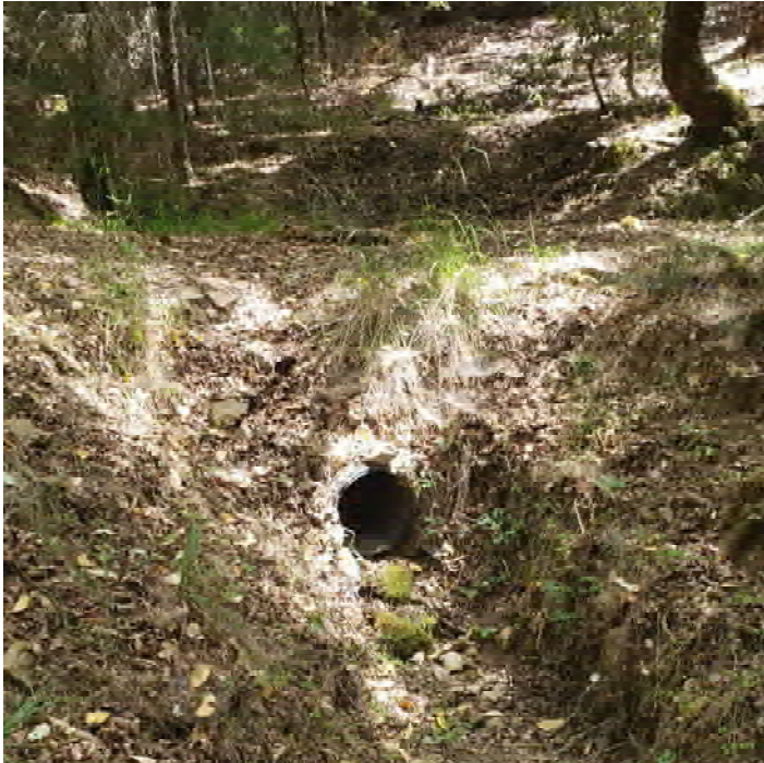
Outlet of the watercourse crossing at Site 17
