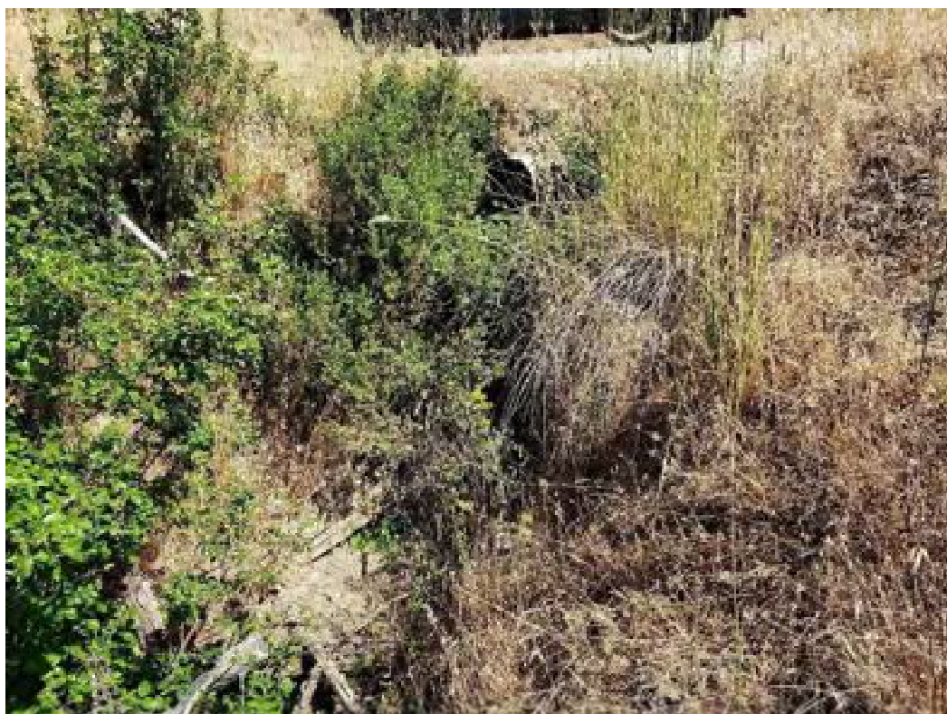
Site 03. Looking at the outlet.
