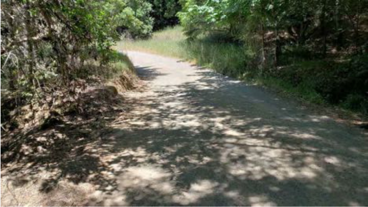
Site 13. Looking up grade at Site 13. A Class III watercourse is diverted down the inside ditch to the right. Re-alignment of this watercourse will consist of a culvert installed diagonally across the road from the grass patch in the upper center right to the lower left of the photo.
