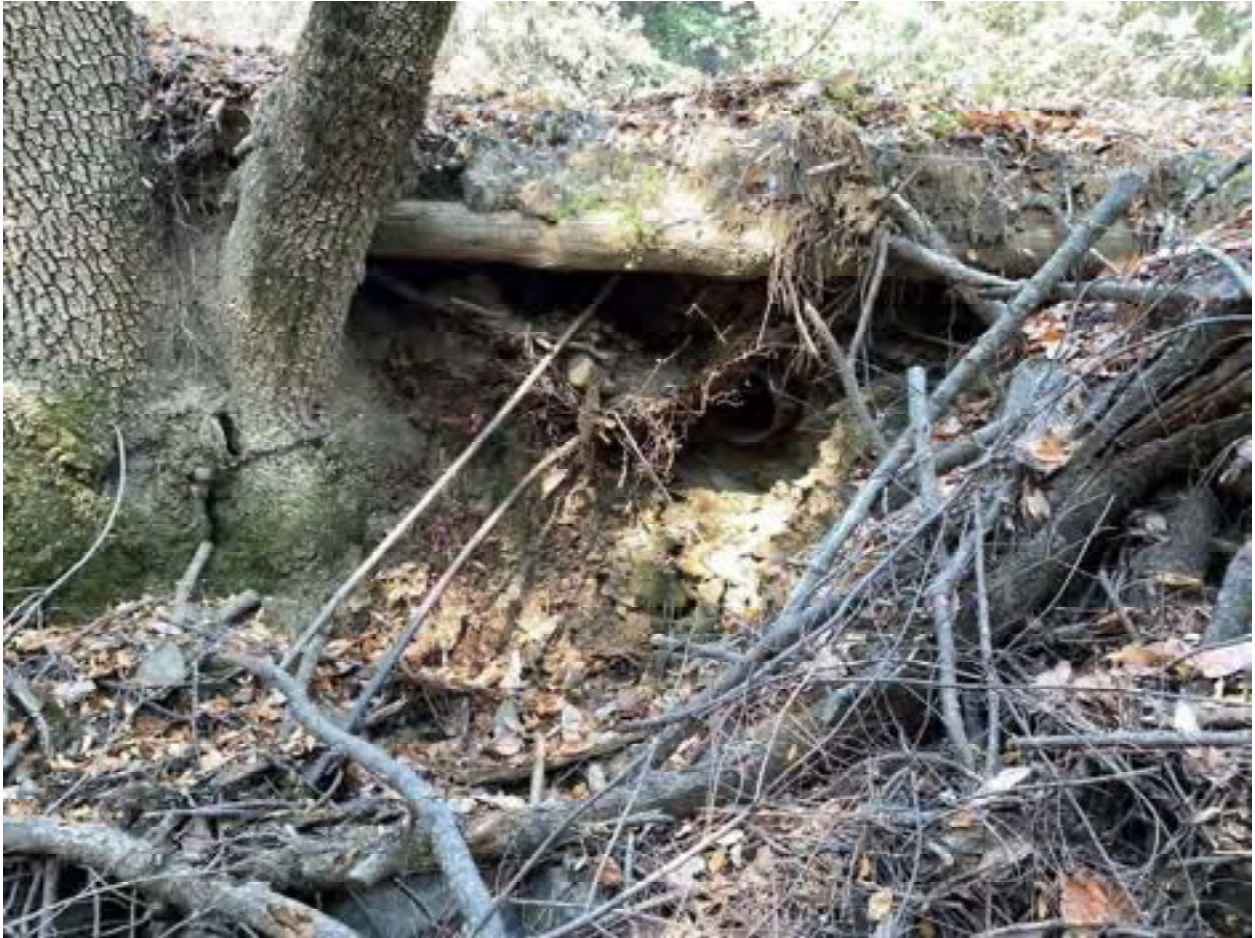
Photo 28: Stream Crossing 07. Looking upstream towards the outlet of the 12-inch diameter culvert at stream crossing 07. Photo date 9-1-2021.
