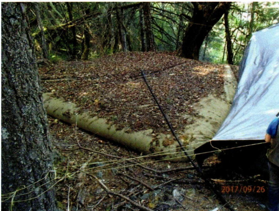
Photo 10 - View of the 20,000-gallon water bladder. Water is pumped from POD #1 upslope to this water bladder and then gravity fed for domestic and irrigation purposes.
