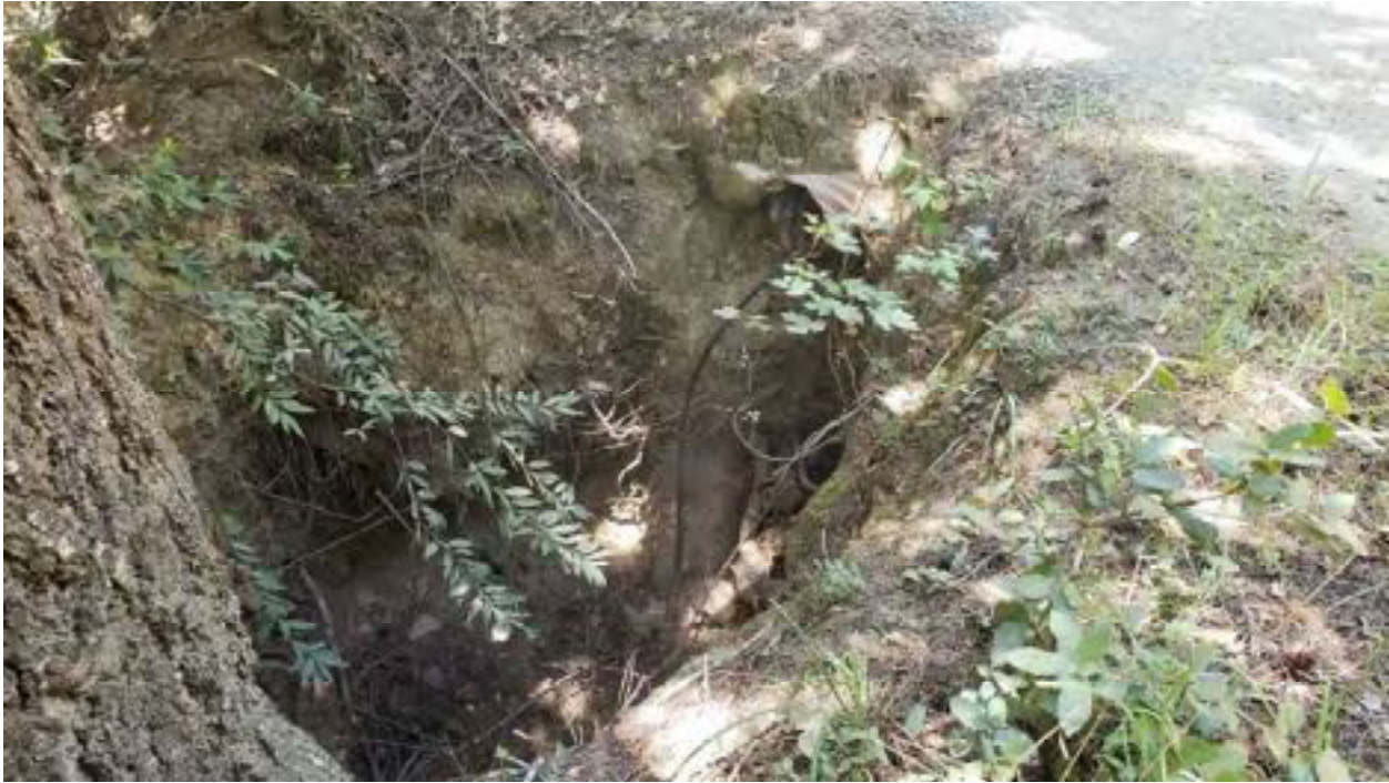
Site 14. Looking at the outlet of the ditch relief culvert.
