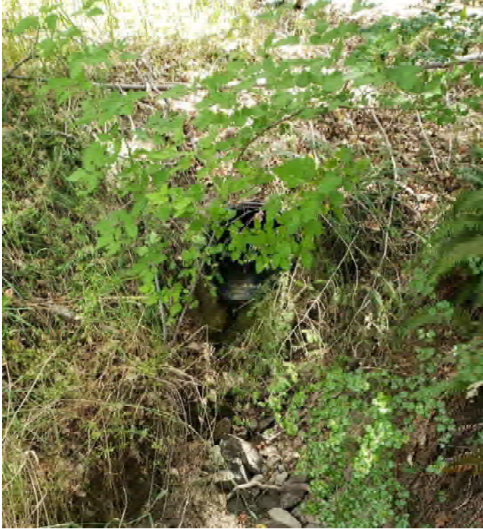
Site 19. Looking at the outlet.
