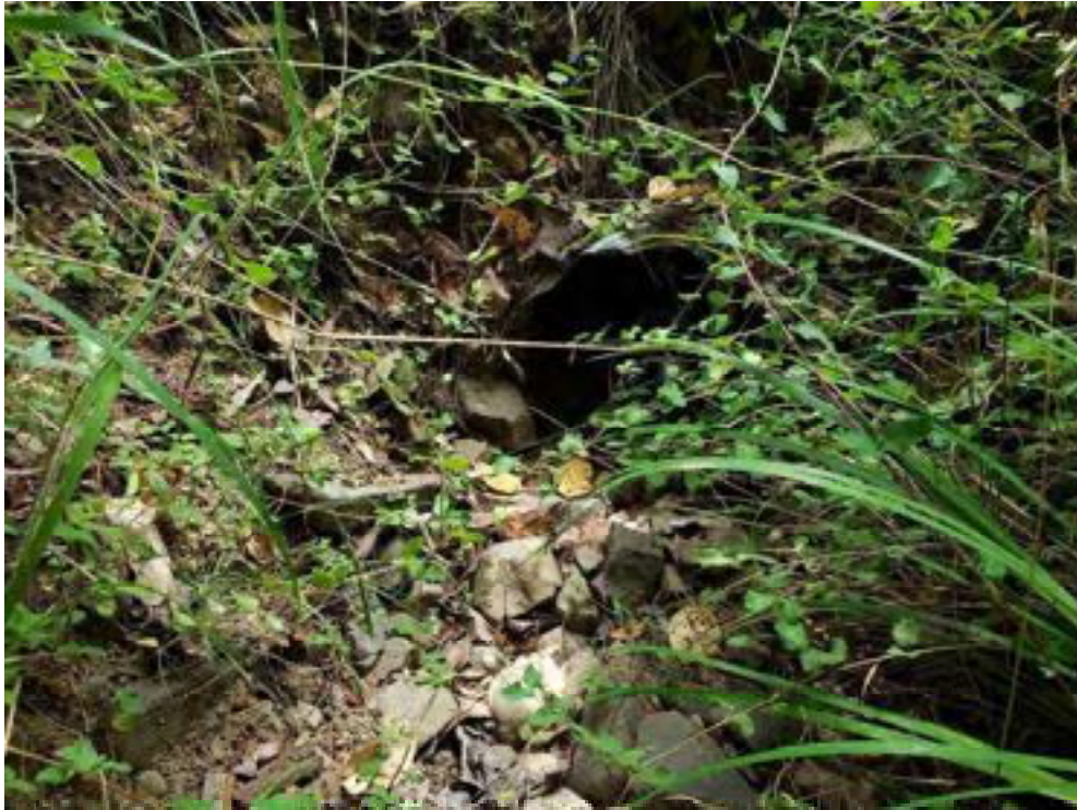
Site 06. Looking at the inlet.
