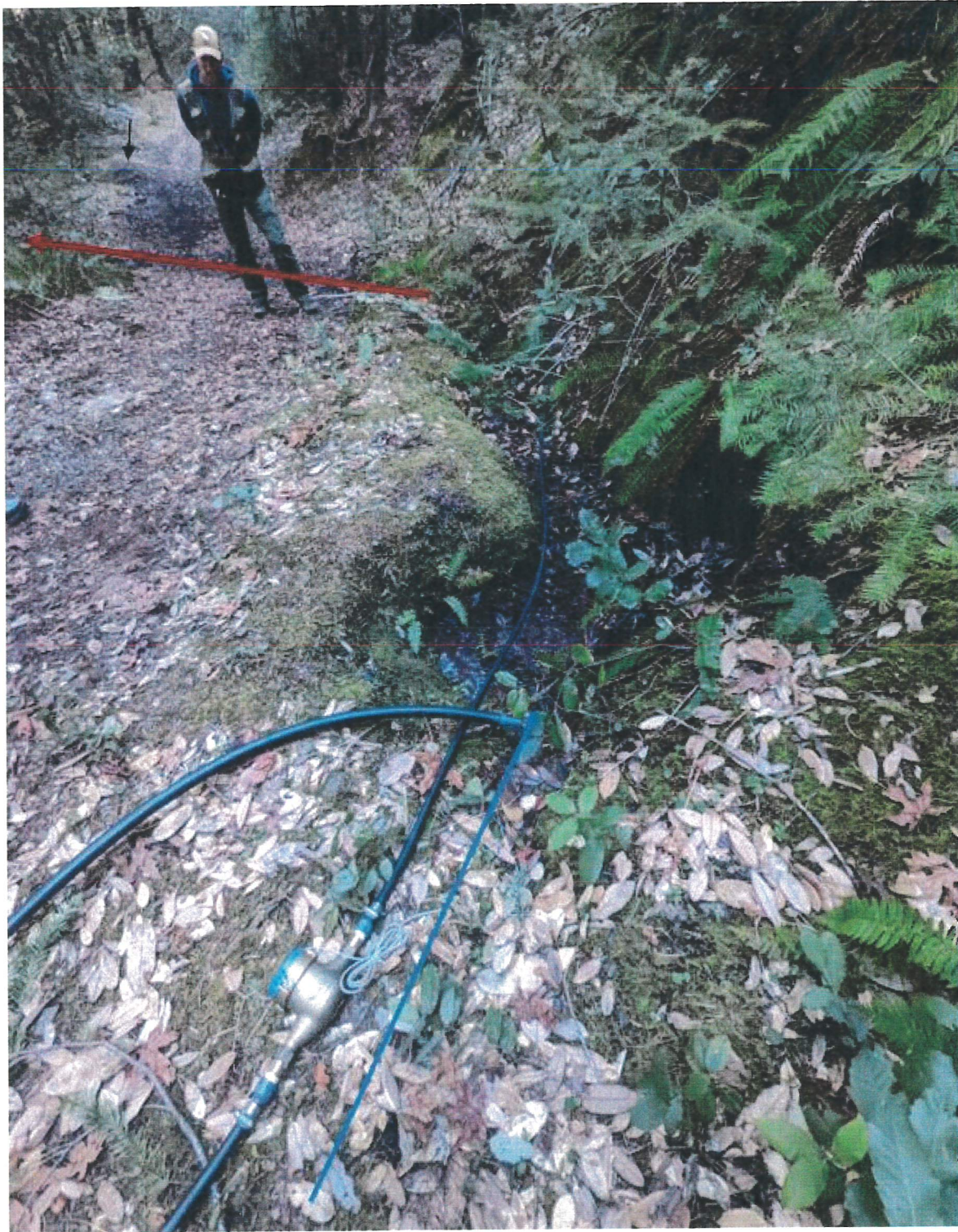
Picture 38: Location where water resurfaces before crossing the road at Crossing 10. The red arrow indicates the location of Crossing 10, rocky ford installation. The black arrow indicated the location of the rolling dip downgrade. Photo date: 2/2/22.
