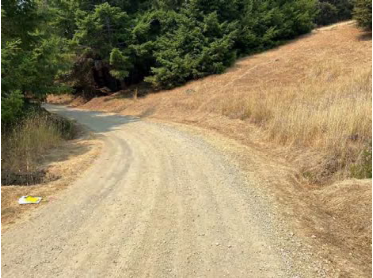
Photo 18: Stream Crossing 05. The roadside approach to stream crossing 05 facing West. Photo date 9-1-2021.
