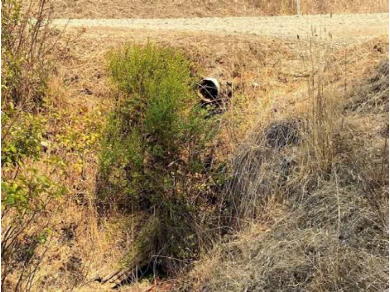
Photo 9: Stream Crossing 03. Looking upstream towards the outlet of the 8-inch diameter culvert at stream crossing 03. Photo date 9-1-2021.
