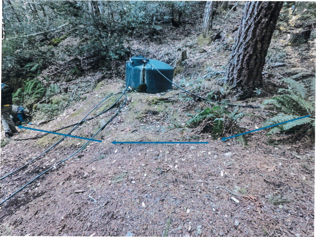
Picture 37: The blue arrows indicate approximate location where channel shall be created to reconnect surface water flow. Photo date: 2/2/22.
