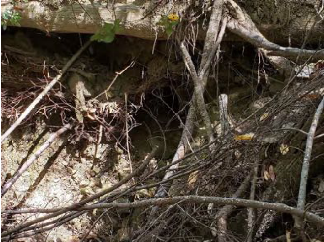
Site 06. Looking at the outlet.
