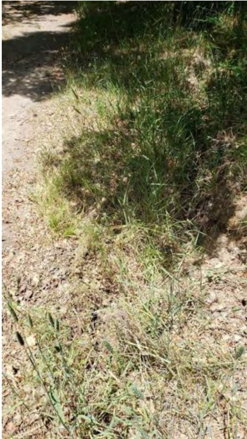
Photo 73: Stream Crossing 35. Looking towards the inlet of the 8-inch diameter culvert at stream crossing 35. Photo date 6-8-2021.
