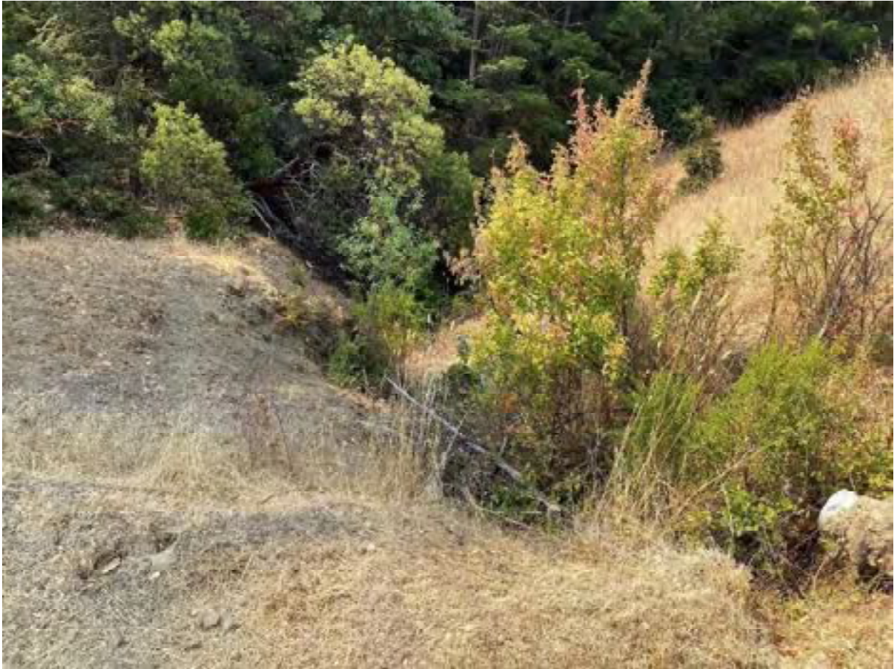
Photo 10: Stream Crossing 03. Looking downstream from the outlet of the 8-inch diameter culvert at stream crossing 03. Photo date 9-1-2021.
