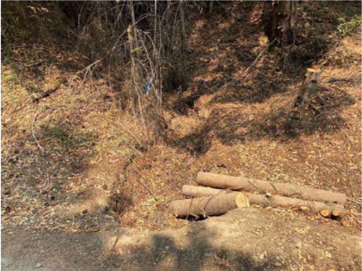
Photo 22: Stream Crossing 06. Looking upstream from the inlet of the 12-inch diameter culvert at stream crossing 06. Photo date 9-1-2021.
