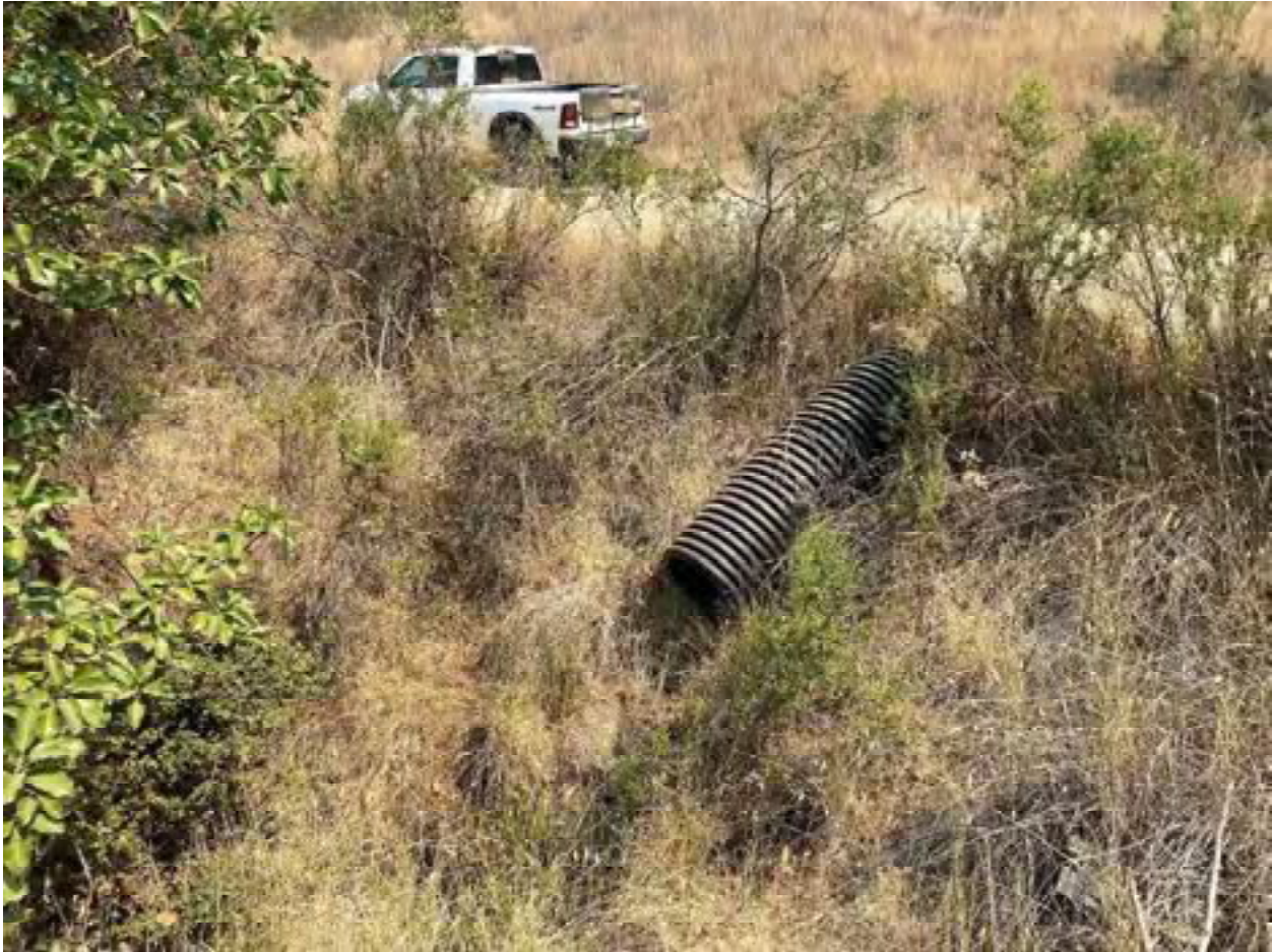
Photo 38: Stream Crossing 11. Looking towards the outlet of the 24-inch diameter culvert at stream crossing 11. Photo date 9-1-2021.
