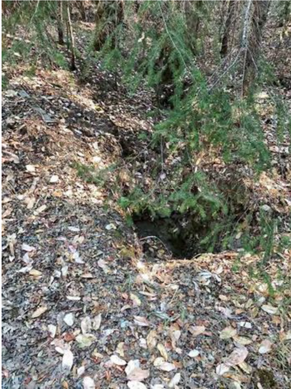
Photo 51: Stream Crossing 17. Looking downstream from the outlet of the 18-inch diameter culvert at stream crossing 17 that is proposed for removal. Photo date 9-1-2021.
