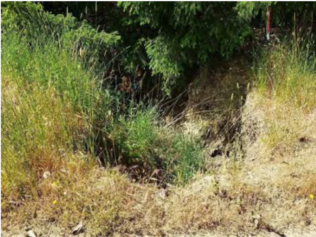
Site 04. Looking down channel from the outlet. The upgraded culvert will extend to where the man is hanging the blue flagging.
