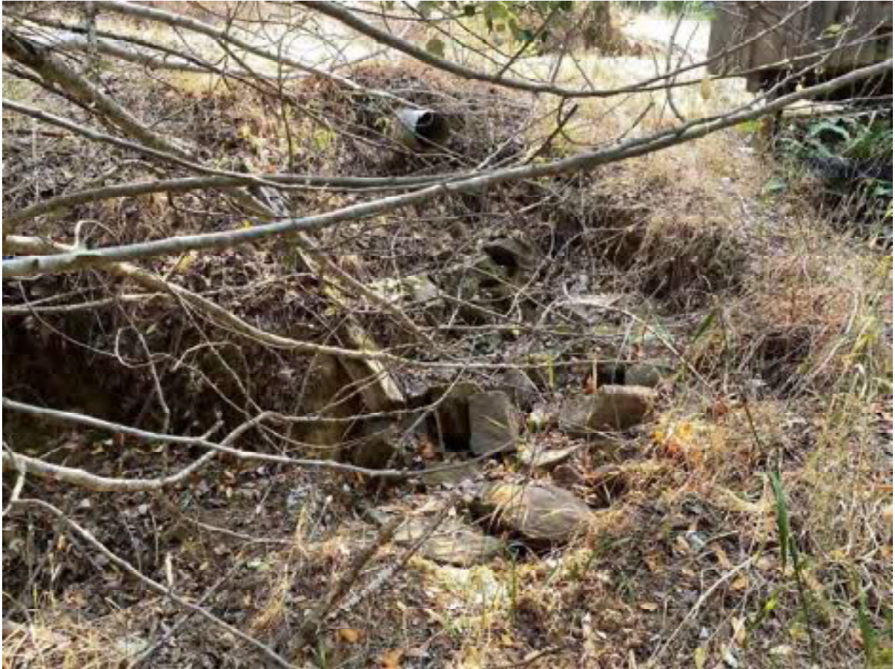
Photo 76: Stream Crossing 35. Looking upstream towards the outlet of the 8-inch diameter culvert at stream crossing 35. Photo date 9-1-2021.
