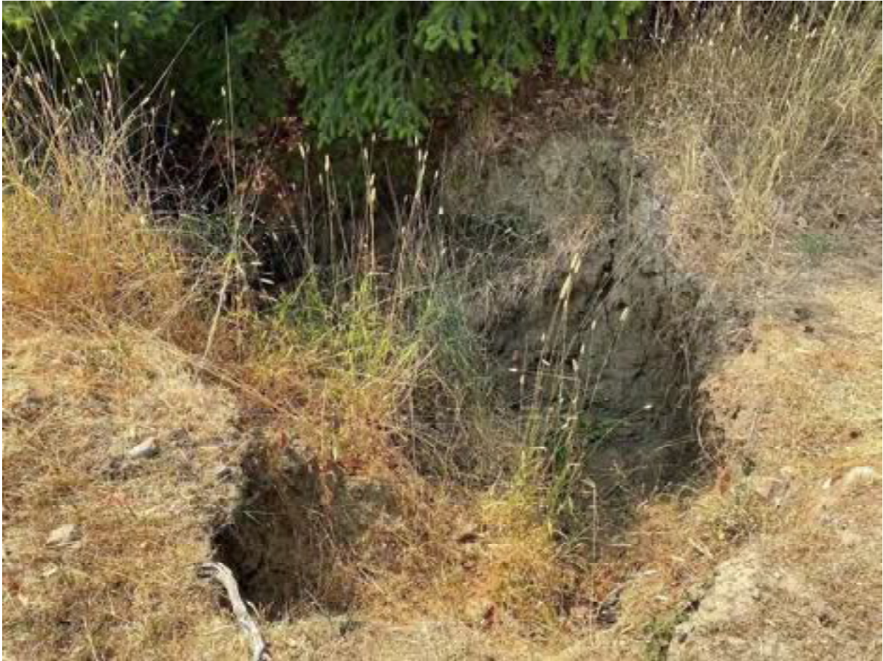
Photo 20: Stream Crossing 05. Looking downstream from the outlet of the 12-inch diameter culvert at stream crossing 05. Photo date 9-1-2021.
