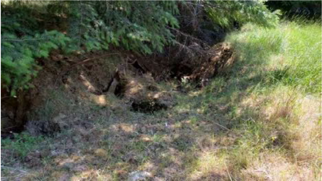
Photo 78: DRC 38: Looking at legacy Refuse downstream from the DRC. Photo date 6-10-2021
