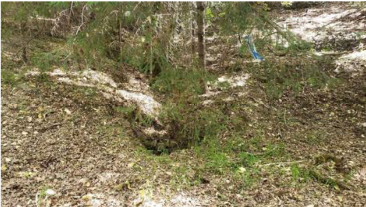
Inlet of the watercourse crossing at Site 17.
