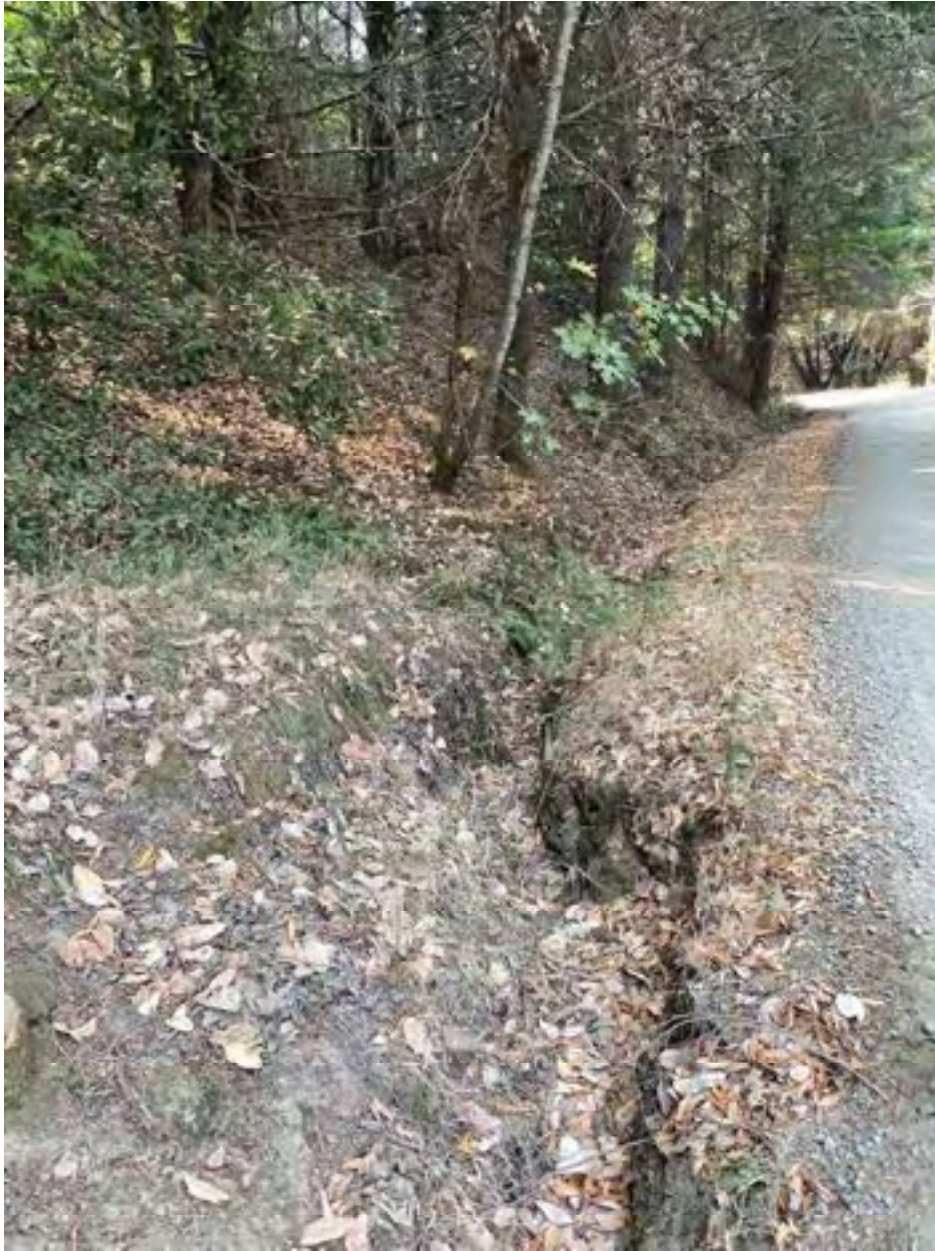
Photo 43: Stream Crossing 13. Looking downslope along the inside ditch that is currently diverting the flow away from the native stream channel at stream crossing 13. Photo date 9-1-2021.
