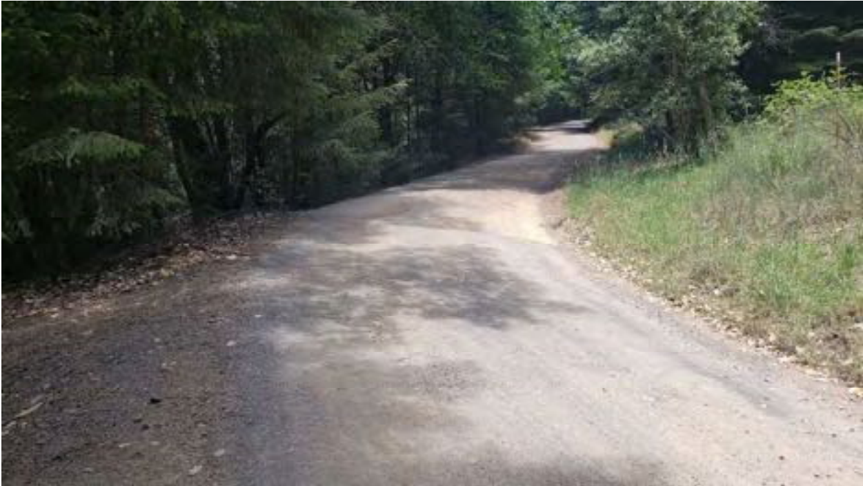
Looking up grade from Site 23 towards Site 14 and 15.
