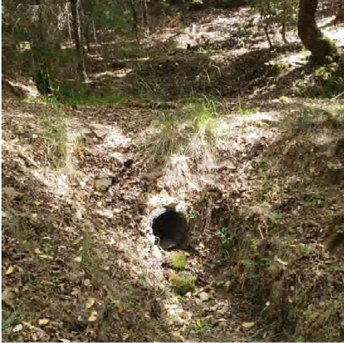
Outlet of the watercourse crossing at Site 17
