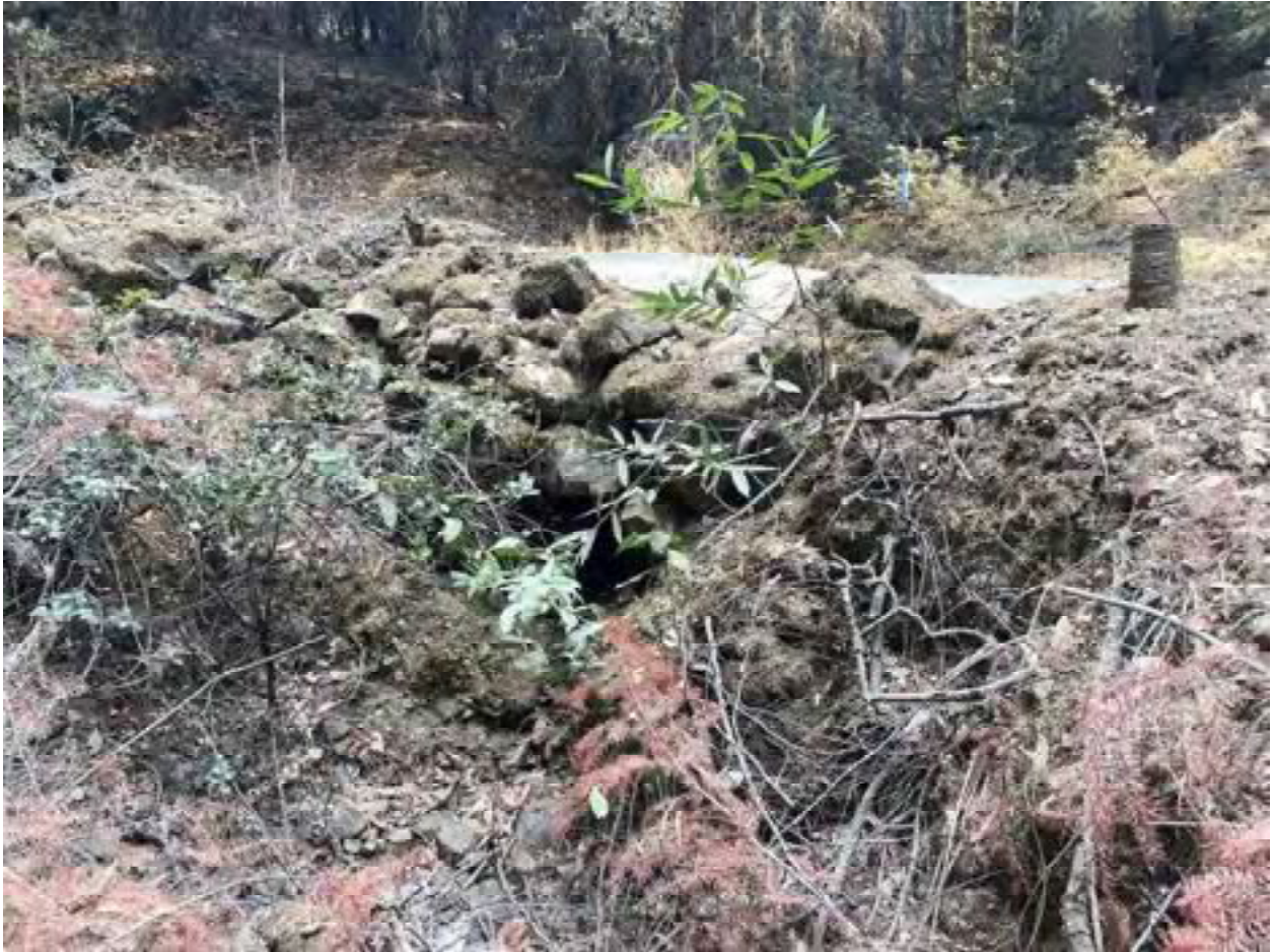
Photo 71: Stream Crossing 26. Looking upstream towards the outlet of the 18-inch diameter culvert at stream crossing 26. Photo date 9-1-2021.
