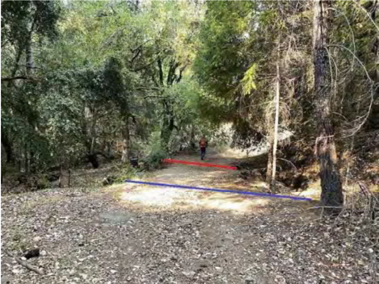
Photo 54: Stream Crossing 19. The roadside approach to stream crossing 19 facing West. The red line depicts where the current misaligned 18-inch culvert is located. The blue line depicts where the native channel used to flow and also where the channel will be realigned to after the stream crossing is decommissioned. Photo date 9-1-2021.
