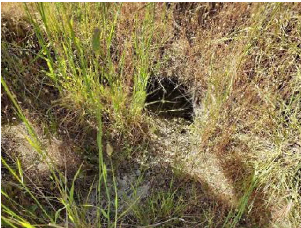
Site 04. Looking at the inlet of the channel.
