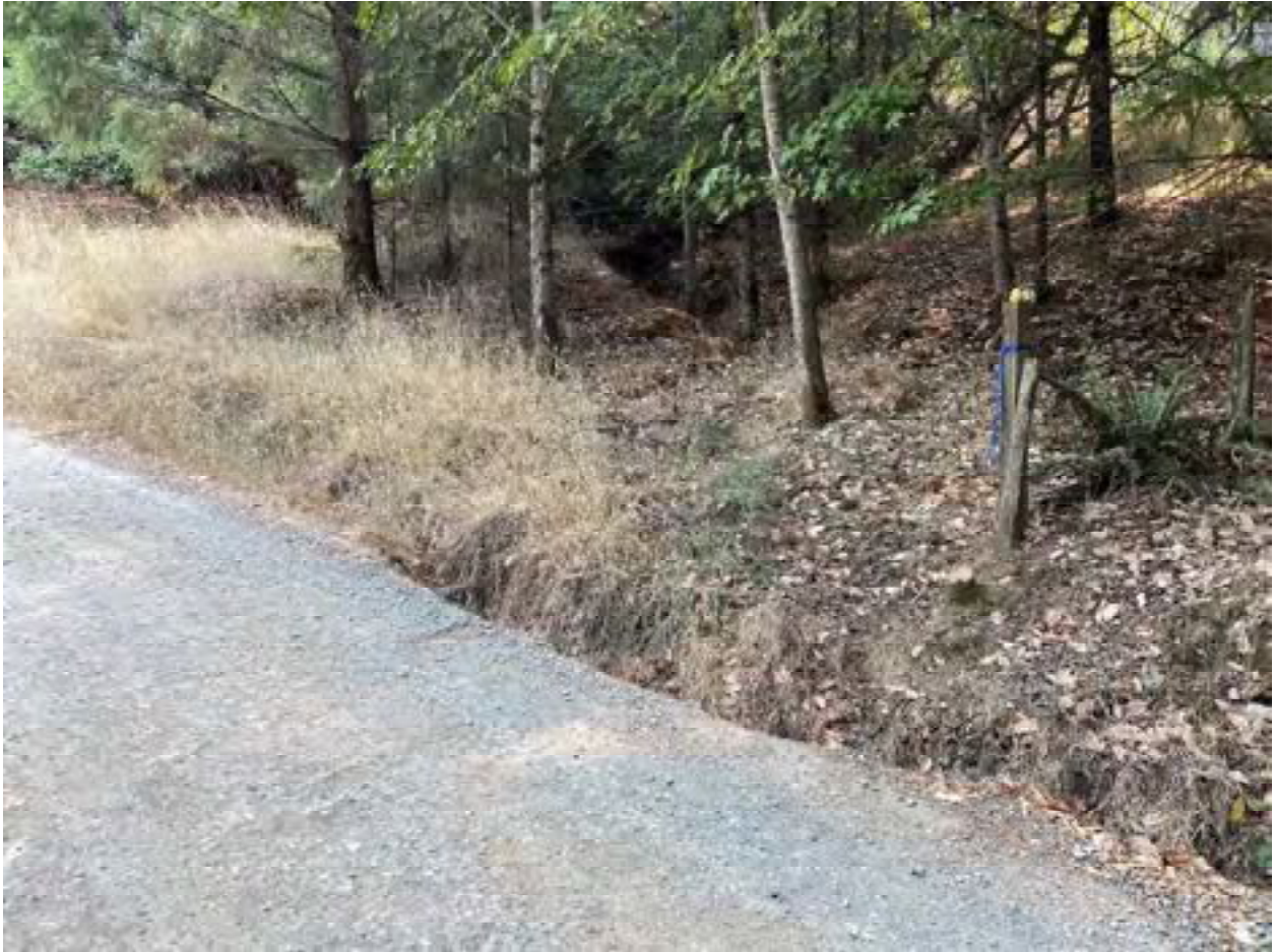
Photo 40: Stream Crossing 13. Looking upstream from the road where inlet of stream crossing 13 is proposed. Photo date 9-1-2021.
