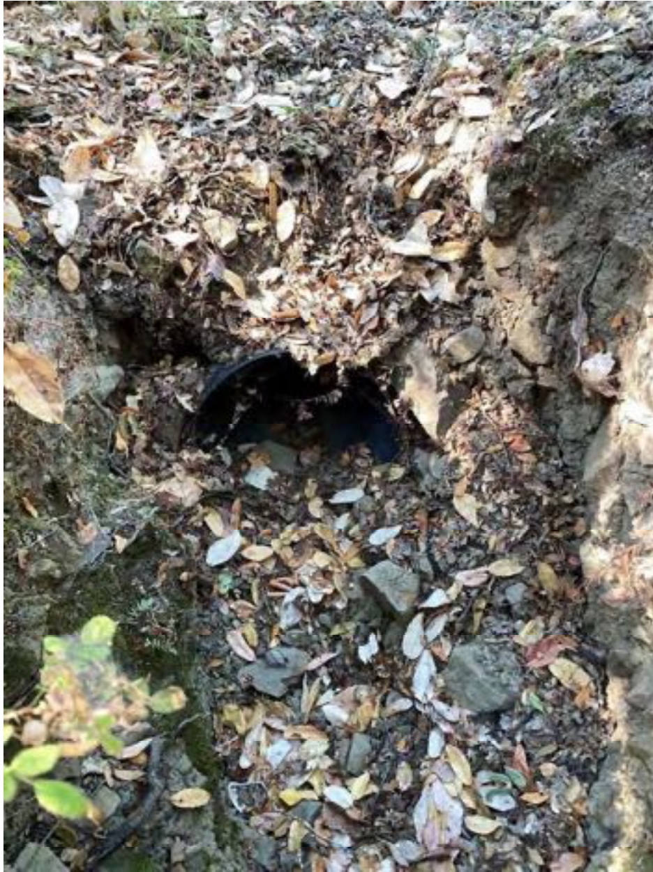
Photo 47: Stream Crossing 17. Looking downstream towards the inlet of the 18-inch diameter culvert at stream crossing 17 that is proposed for removal. Photo date 9-1-2021.
