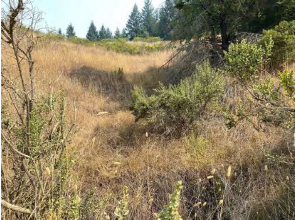
Photo 36: Stream Crossing 11. Looking upstream from the inlet of the 24-inch diameter culvert at stream crossing 11. Photo date 9-1-2021.
