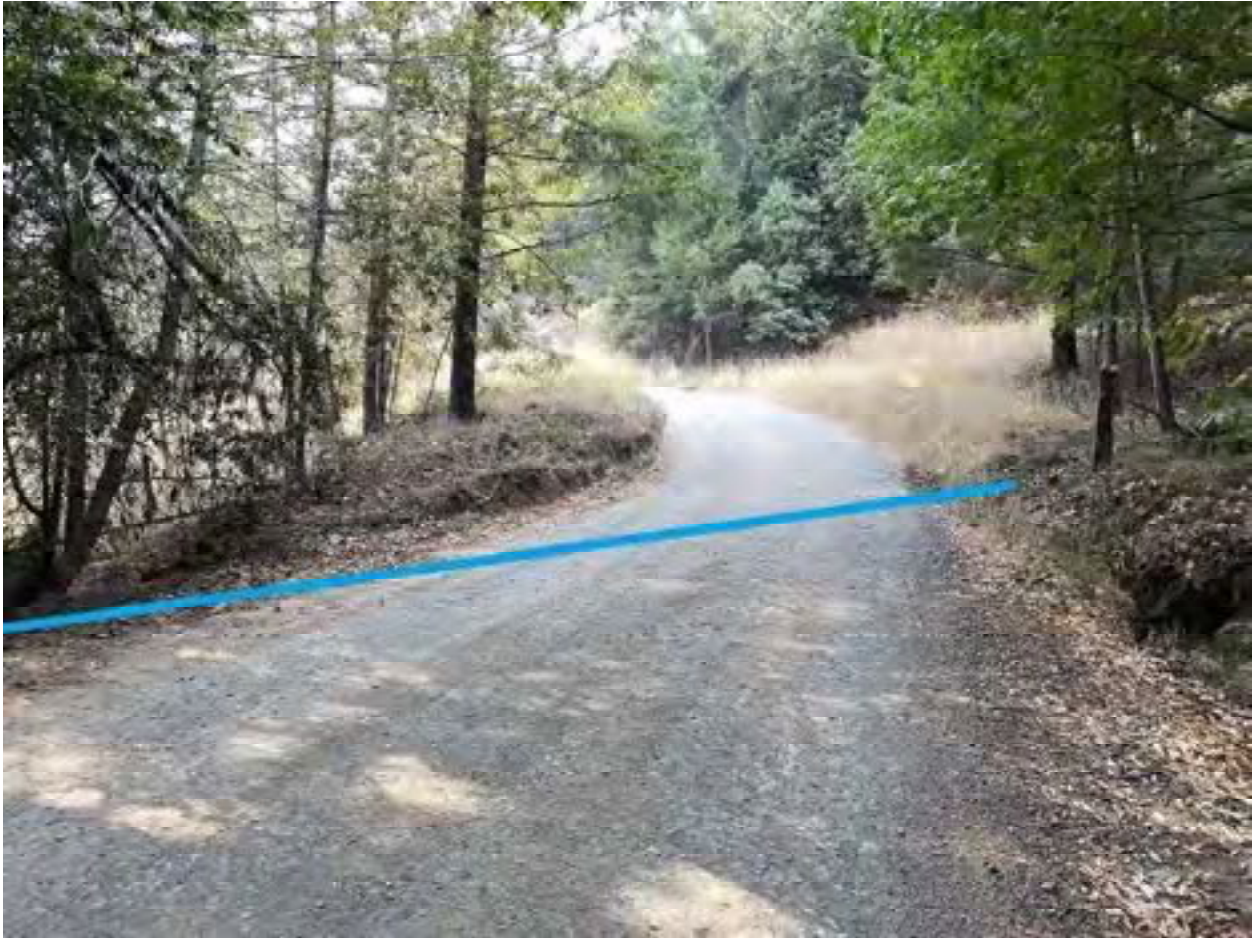
Photo 42: Stream Crossing 13. The roadside approach to stream crossing 13 facing North. The blue line indicates where the proposed culvert will be installed in-line with the native stream channel. Photo date 9-1-2021.
