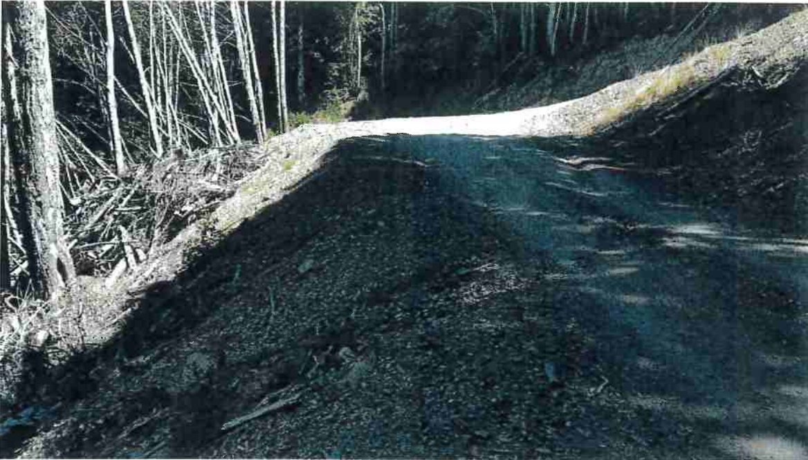
Picture 7: Road Point 5, the Discharger will apply road rock to the three-way intersection to secure the roads surface and slope.
