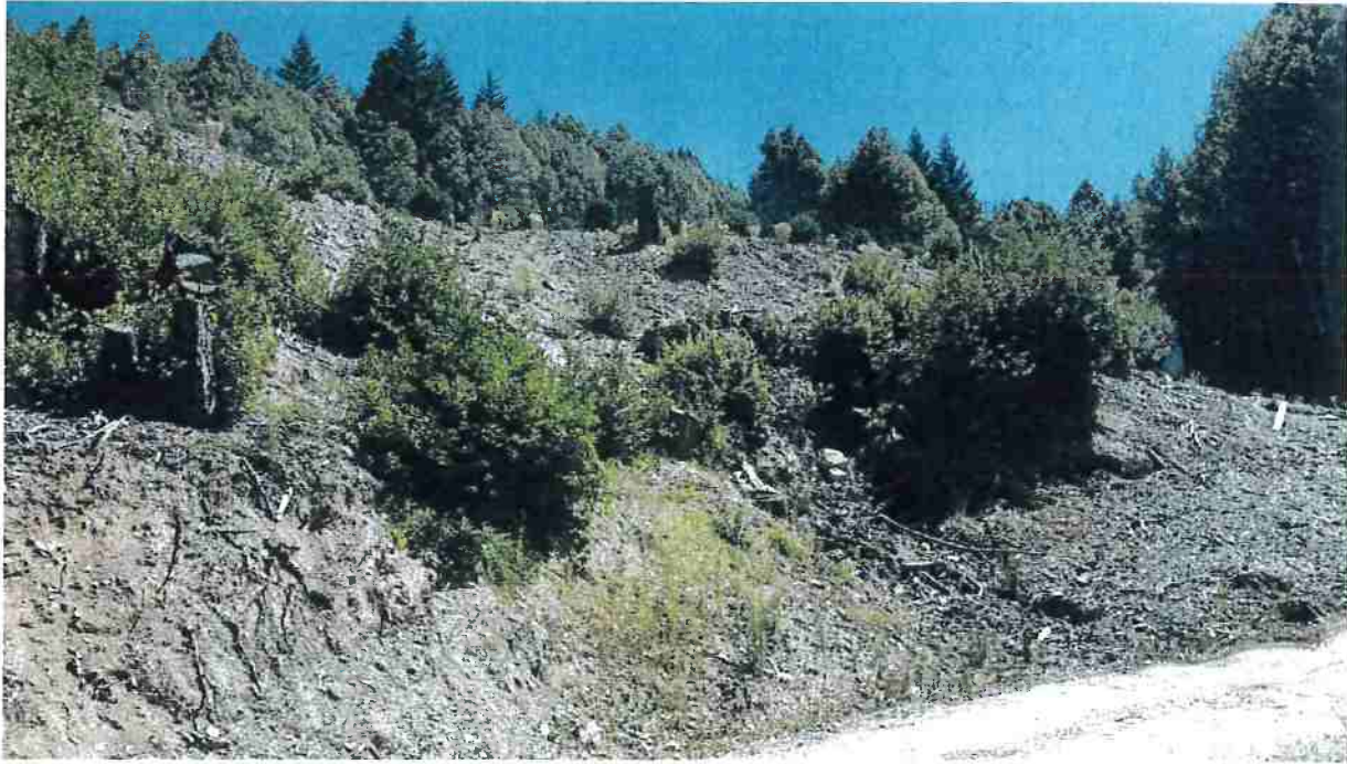
Picture 9: Looking up at Map Point 1 from Road Point 3.
