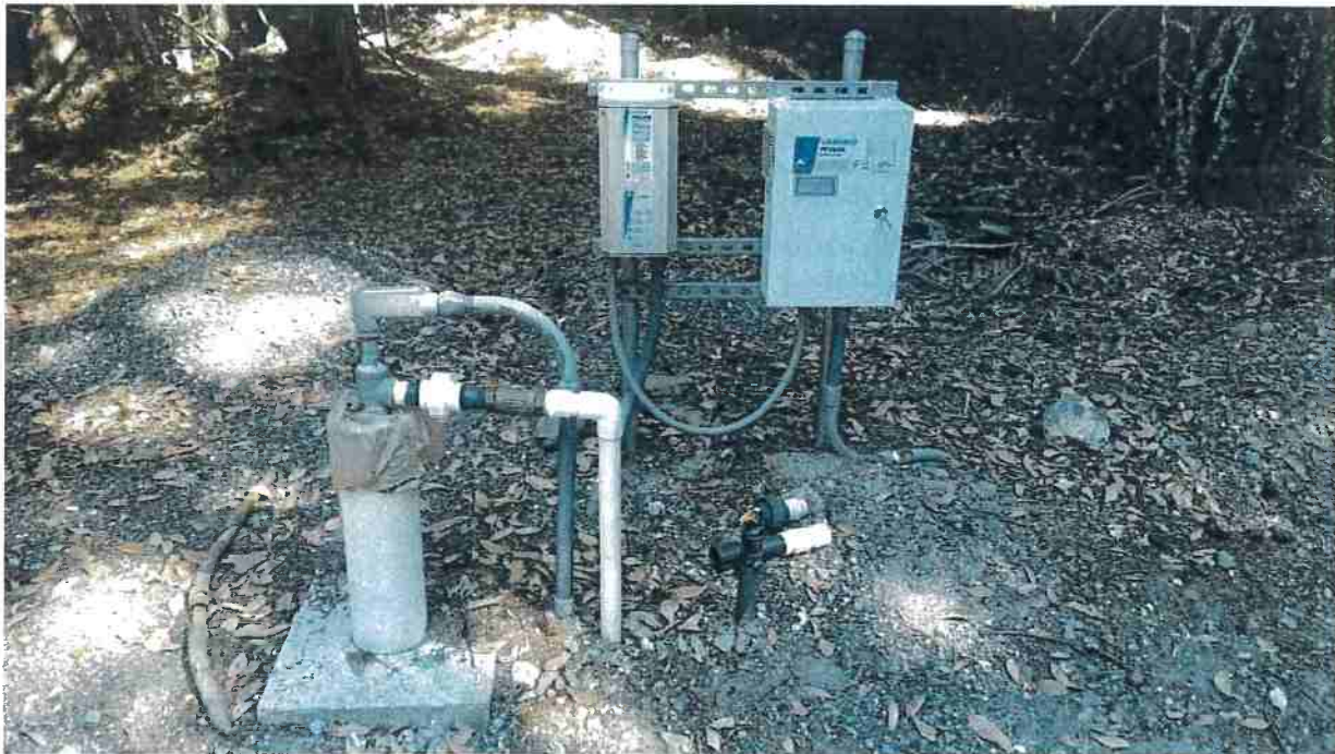
Picture 4: Source of water for the property, a 120 foot well drilled by Fisch Drilling.
