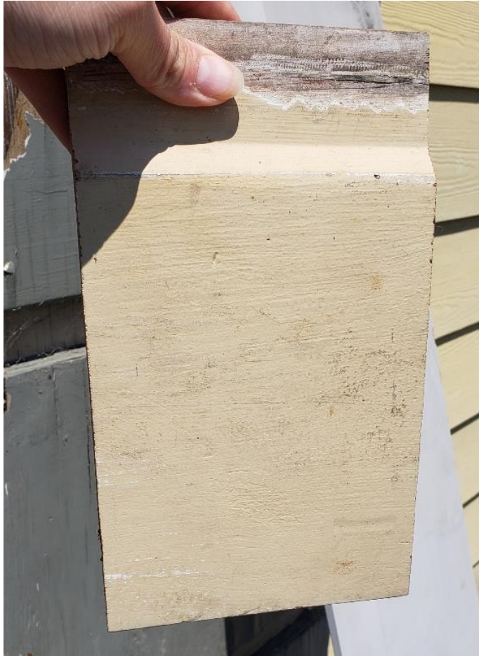
Figure 4: Piece of existing 5/16-inch by 10-inch Redwood siding
