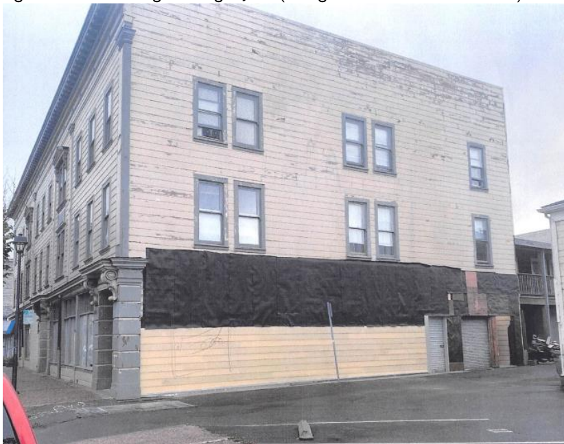
Figure 3: South-facing building façade (facing north east from D Street)
