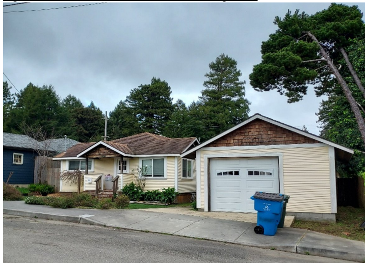
Figure 4: Street View from I Street (facing east)
