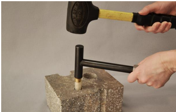
Figure 2. Installing the VAPOR PIN®
