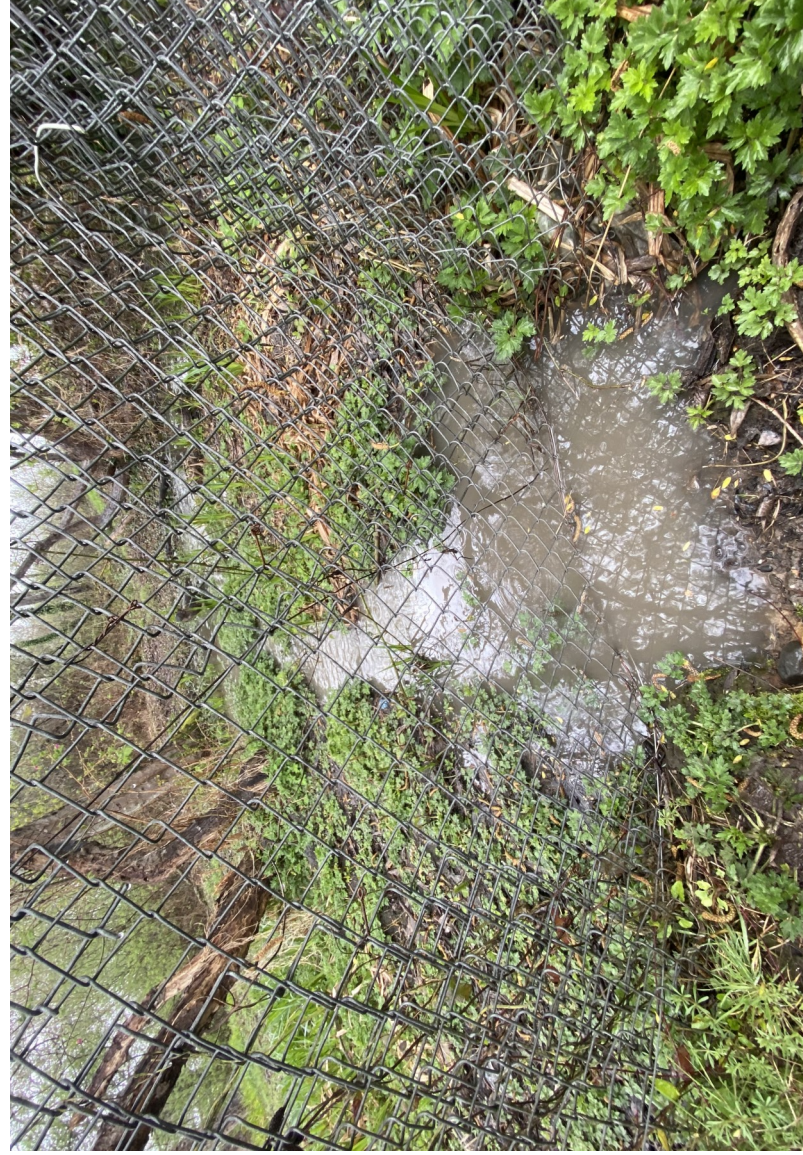
Northern discharge sampling location, D#2. Discharge received from subsurface corrugated pipe receiving runoff from concrete lined ditch and adjacent areas.
