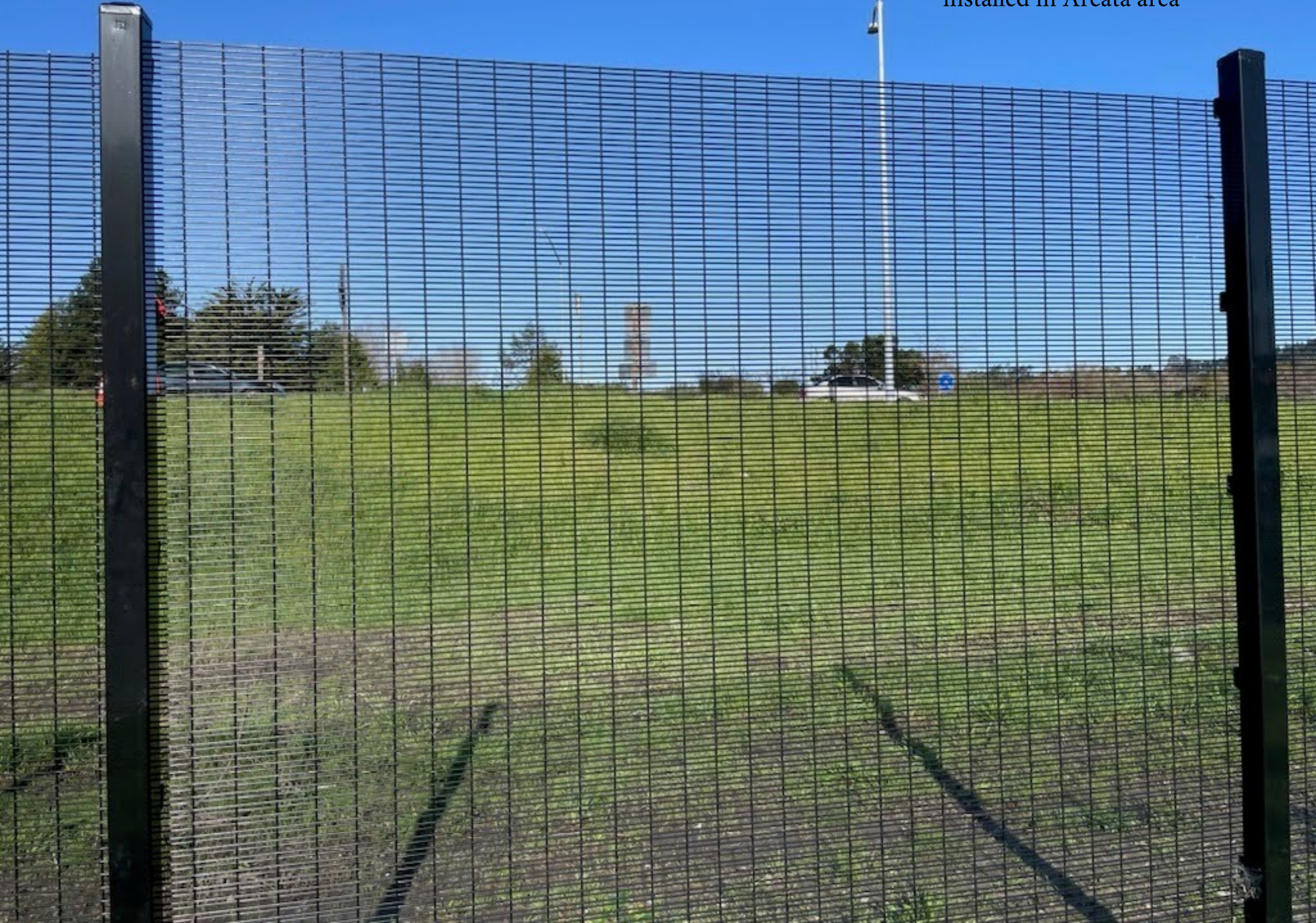
Example photo of Beta Fence installed in Arcata area
