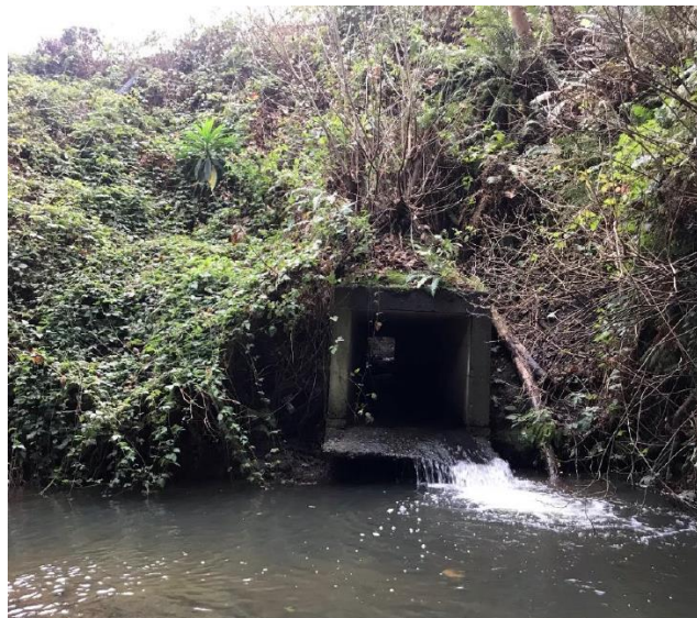
Figure 1. Mill Creek culvert outlet at Weber Street.
