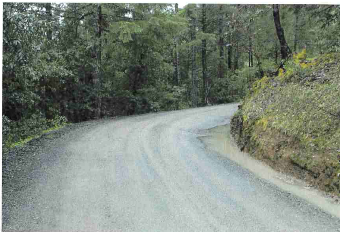
Photo 6. Mile 1.6: Pinch Point 3 (first pinch point on gravel segment), blind corner, 16-ft road surface + 1-ft shoulders.
