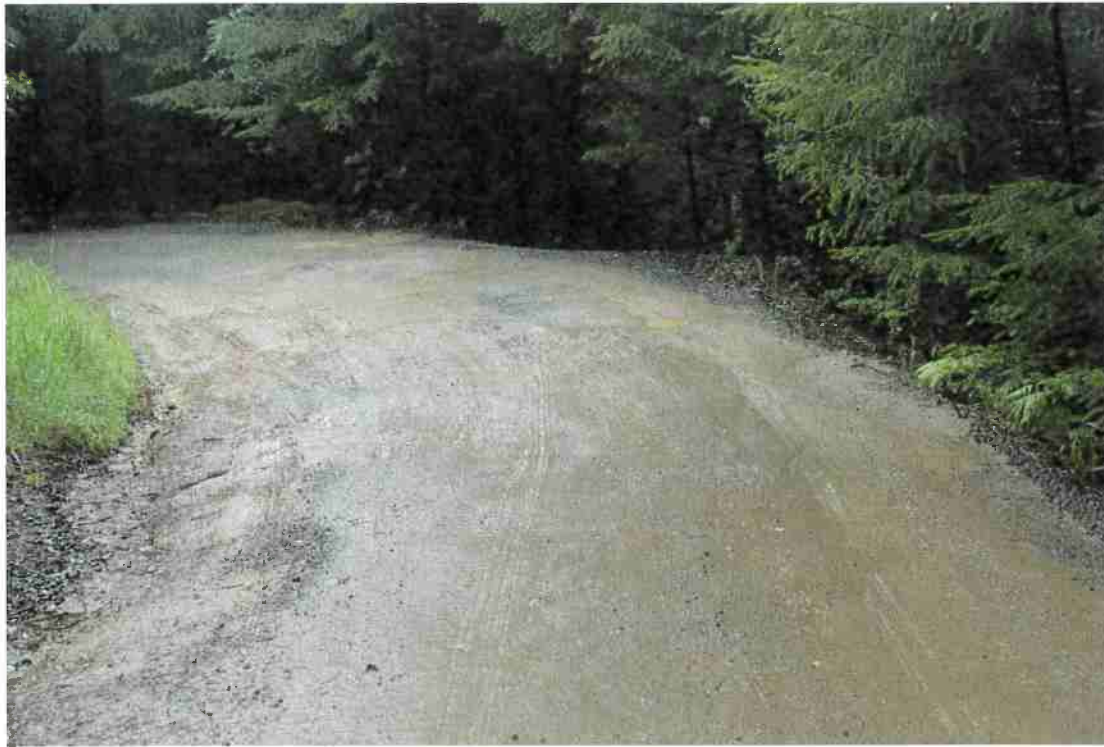
Photo 3. Mile 6.0: 18-ft road width with 1-ft shoulders.
