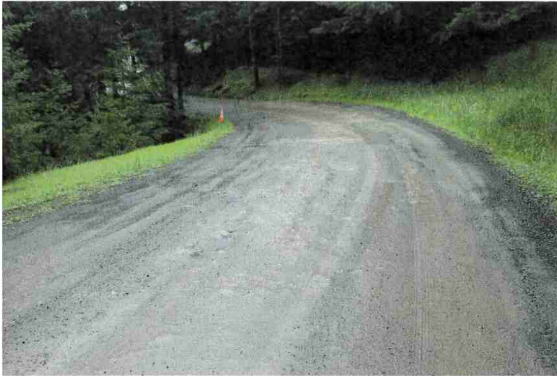
Photo 5. Mile 5.6: 20-ft road width with 2-ft shoulder.
