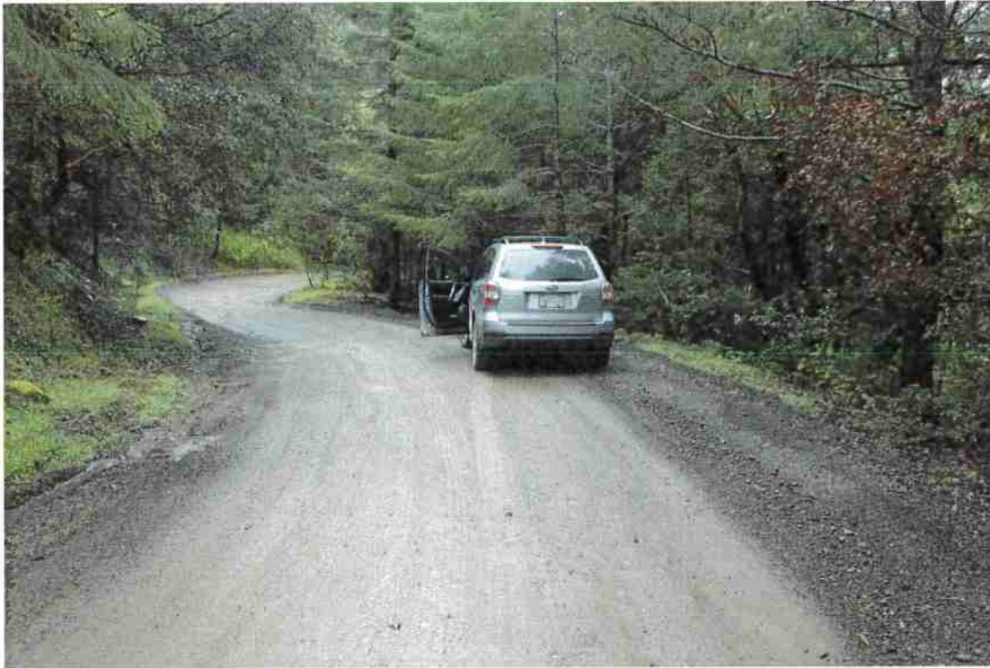
Photo 13. Mile 6.6: 18-ft road width with 2-ft shoulders.
