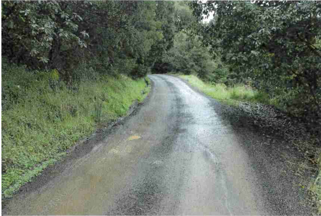
Photo 11. Mile 6.5: 12-ft road width with 1-ft shoulder.
