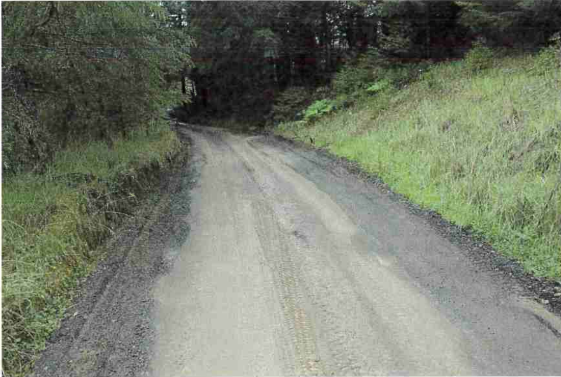
Photo 17. Mile 6.8: 12-ft road width with no shoulder.
