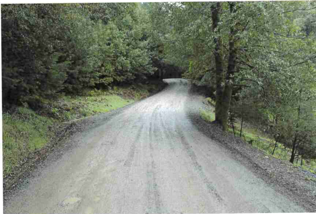
Photo 12. Mile 3.7: Typical 20-ft-wide road segment.
