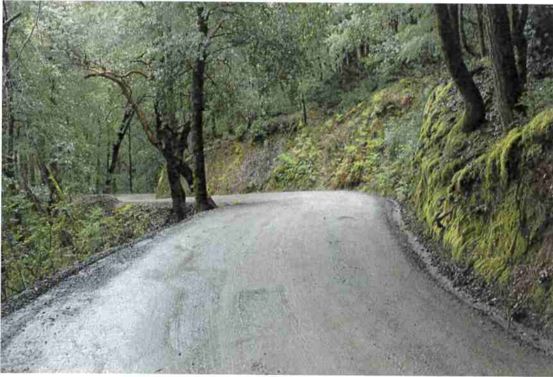
Photo 9. Mile 2.6: Typical 15-ft-wide road segment with good visibility, blind corner in background.
