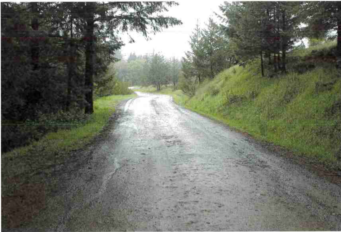
Photo 7. Mile 5.7: 20-ft road width with 2-ft shoulder.
