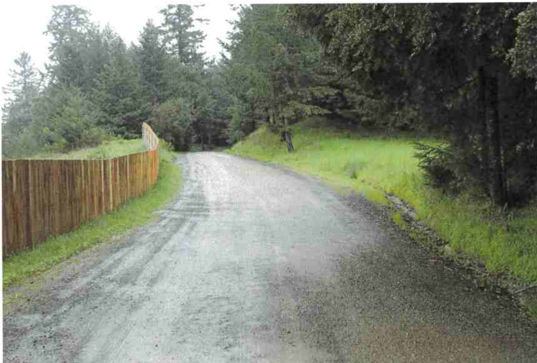
Photo 4. Mile 5.5: 20-ft road width with 2-ft shoulder.
