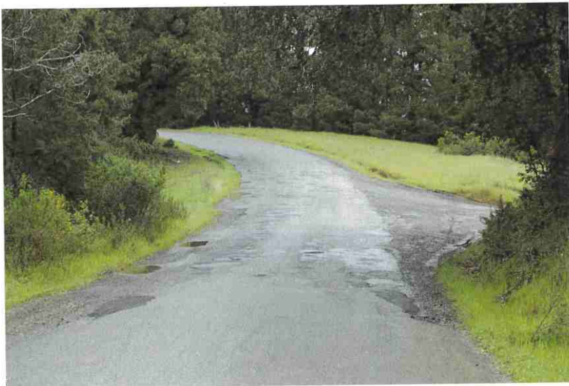
Photo 4. Mile 1.3: Typical lower gradient paved road segment.
