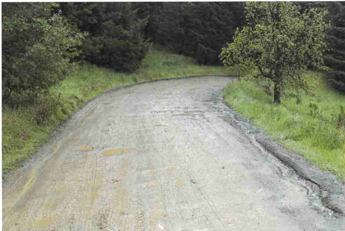
Photo 2. Mile 5.9: 18-ft road width with 1-ft shoulders.
