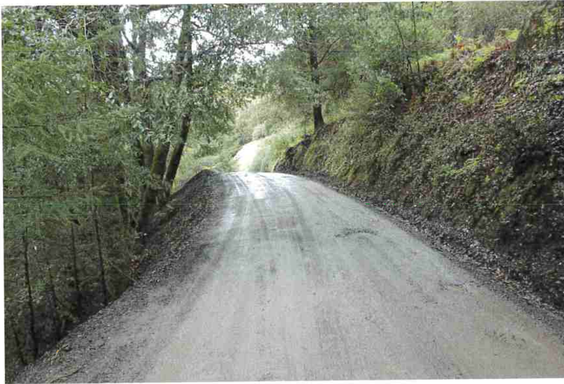
Photo 11. Mile 3.7: 12-ft-wide Pinch Point 5.
