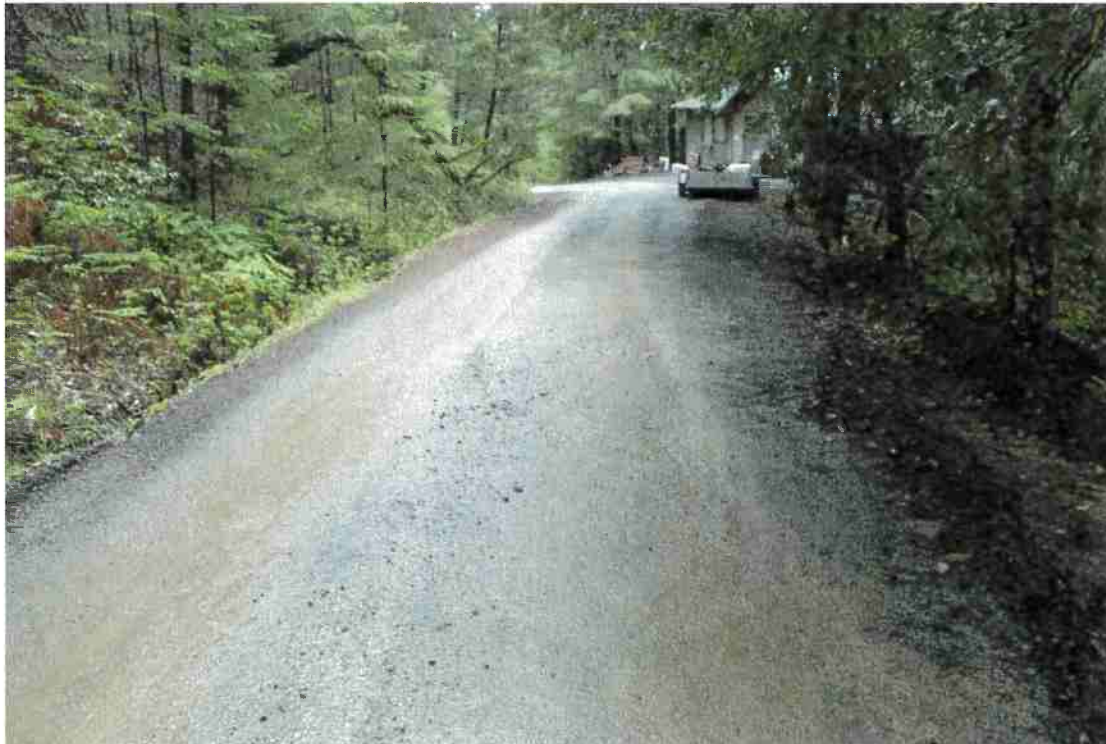
Photo 16. Mile 6.7: 16-ft road width with 1-ft shoulder.
