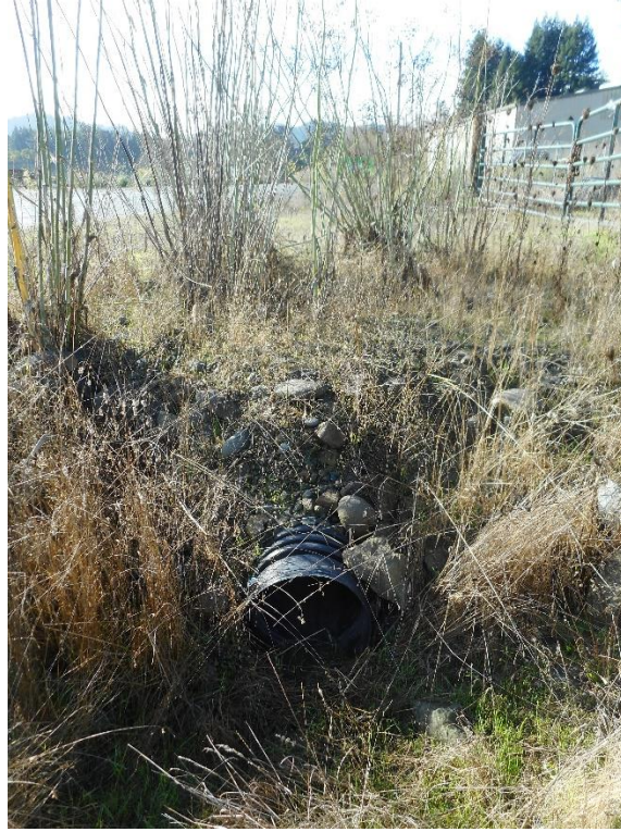
Figure 7: Culvert entrance from in-board ditch. Image taken facing south.
