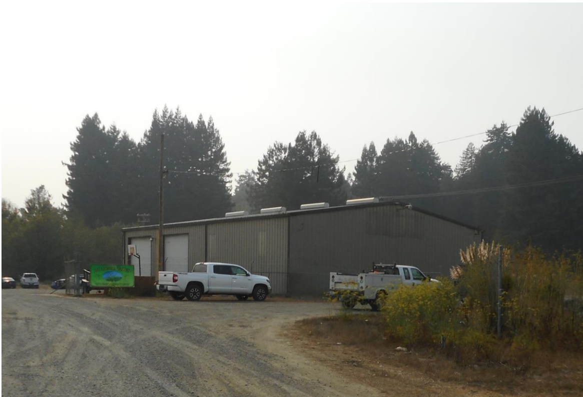
Figure 1: Existing 60' x 80' Onsite Metal Building
