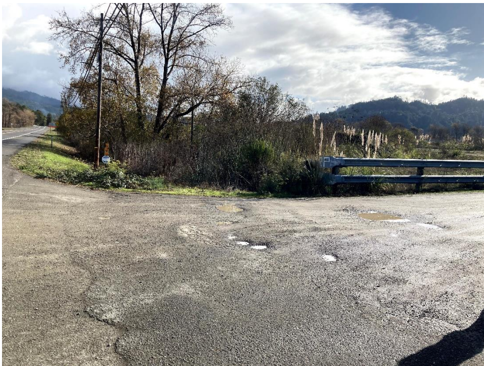
Figure 4: RP 1. Intersection of Private driveway and Highway 36. Image shown facing east toward Highway 36.
