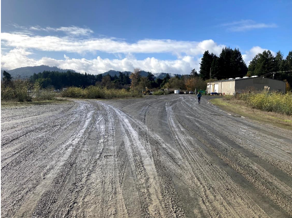
Figure 5: RP 2. 48' Graveled road width. Image shown facing southwest.
