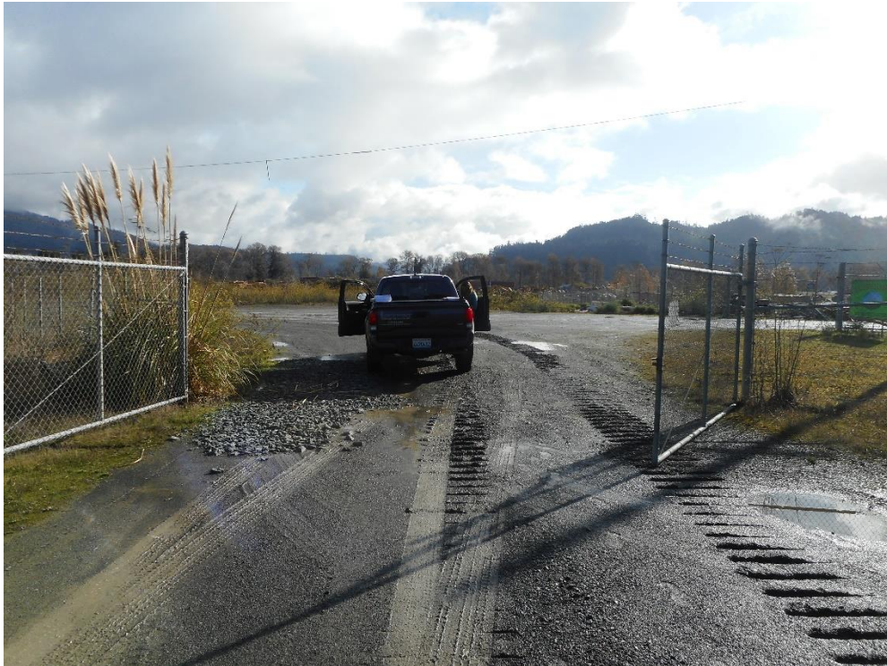
Figure 9: RP 3. Gate 23' in road width. Image facing east.
