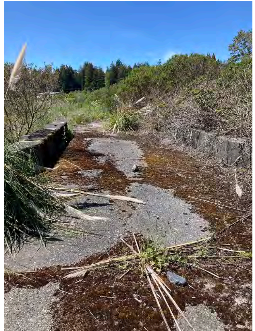
Photo 6. Truck reload. Image date: May 3, 2022.
