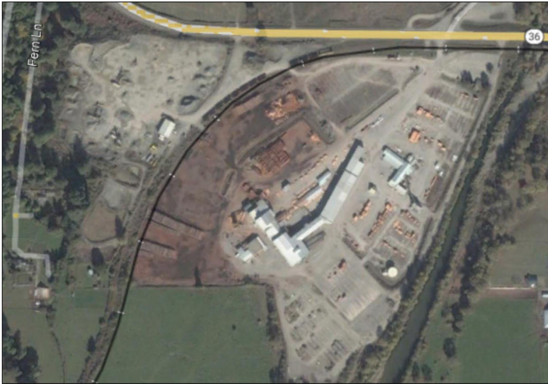
Photo 1. Ariel image from 2005 showing the Study Area utilized as a log deck. Photo taken from Google Earth Pro, 2022.
