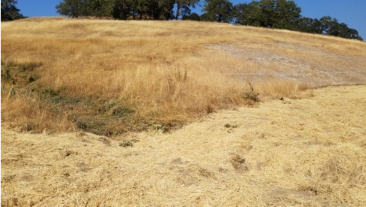
CA-3 debris and soil removed. Strawed and seeded
