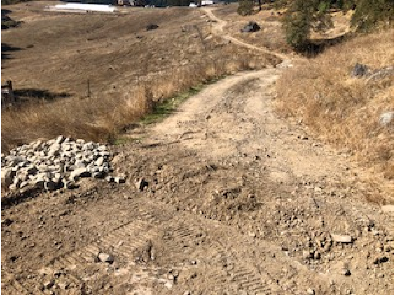
Figure 10: Installation of WB-7 in the foreground showing the waterbar and the riprap armoring at the outlet.
