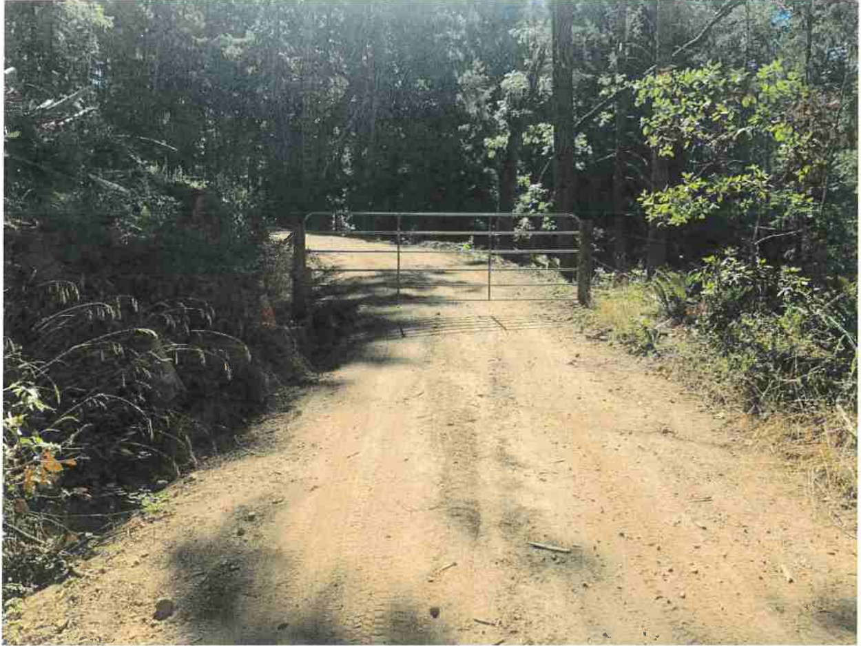
2.0 mm Photo 11 our gate and property line
