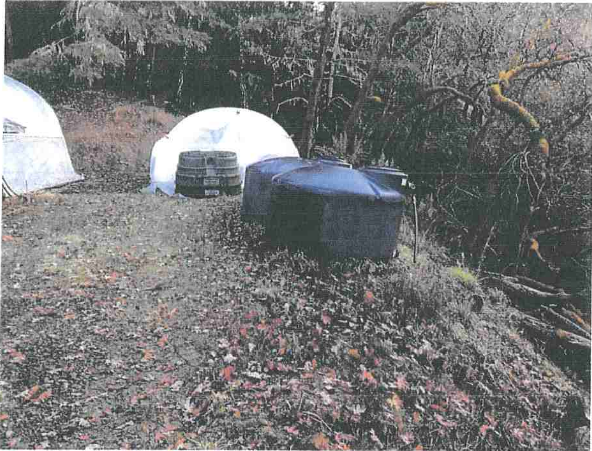
Photo #2: Water storage tanks that are inadequately installed within the riparian area of the adjacent Class II watercourse. These water storage tanks will be relocated to a location outside of all riparian buffer zones, and installed on flat stable ground. Photo Date: 11/27/2017.
