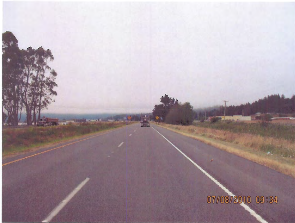
Photograph of Existing northbound Route 101 south of Indianola Cutoff
