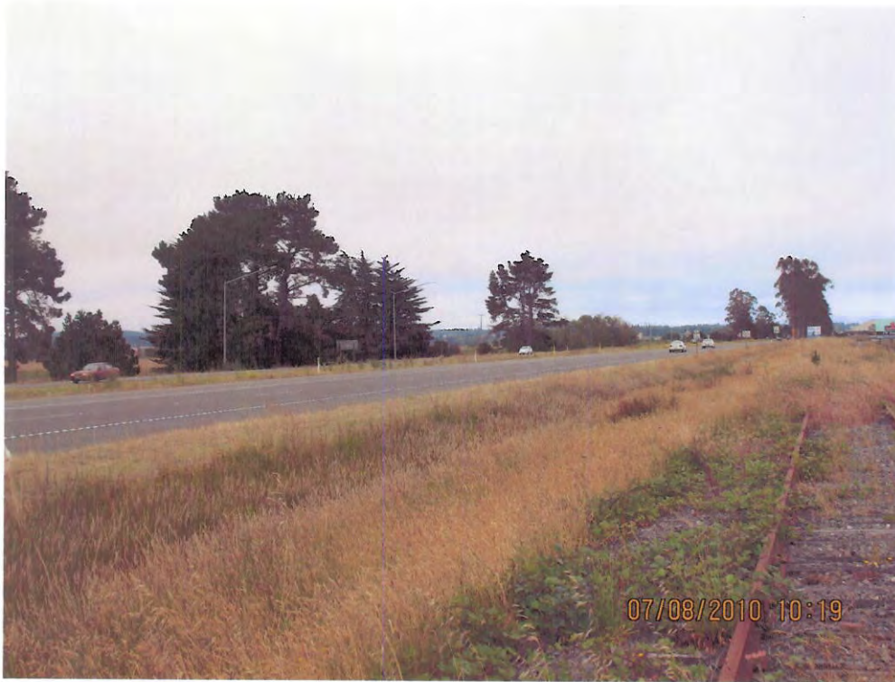
Photograph of existing southbound Route 101 South of Indianola Cutoff
