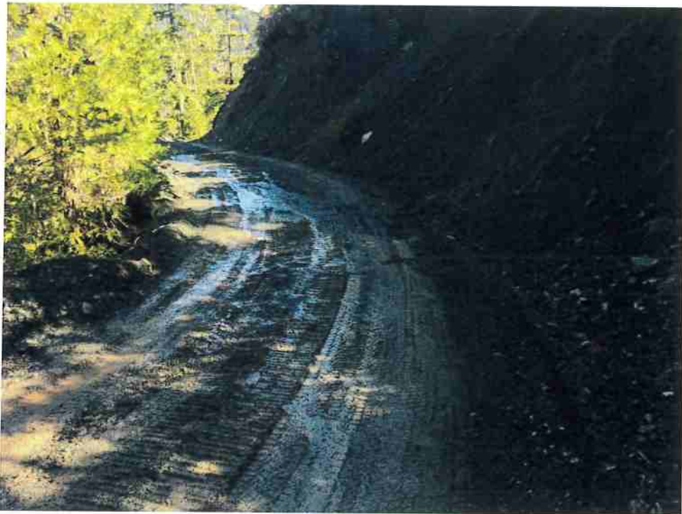
Photo 9. MP9 - Road surface at small fill crossing.
