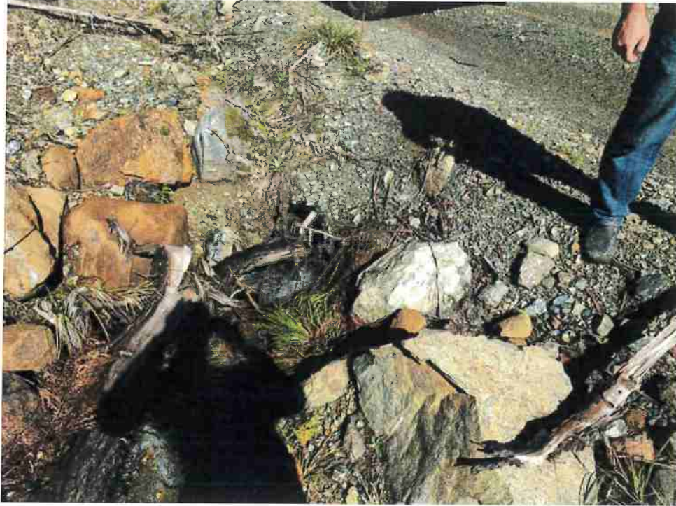
Photo 3. MP7 - Culvert inlet.
