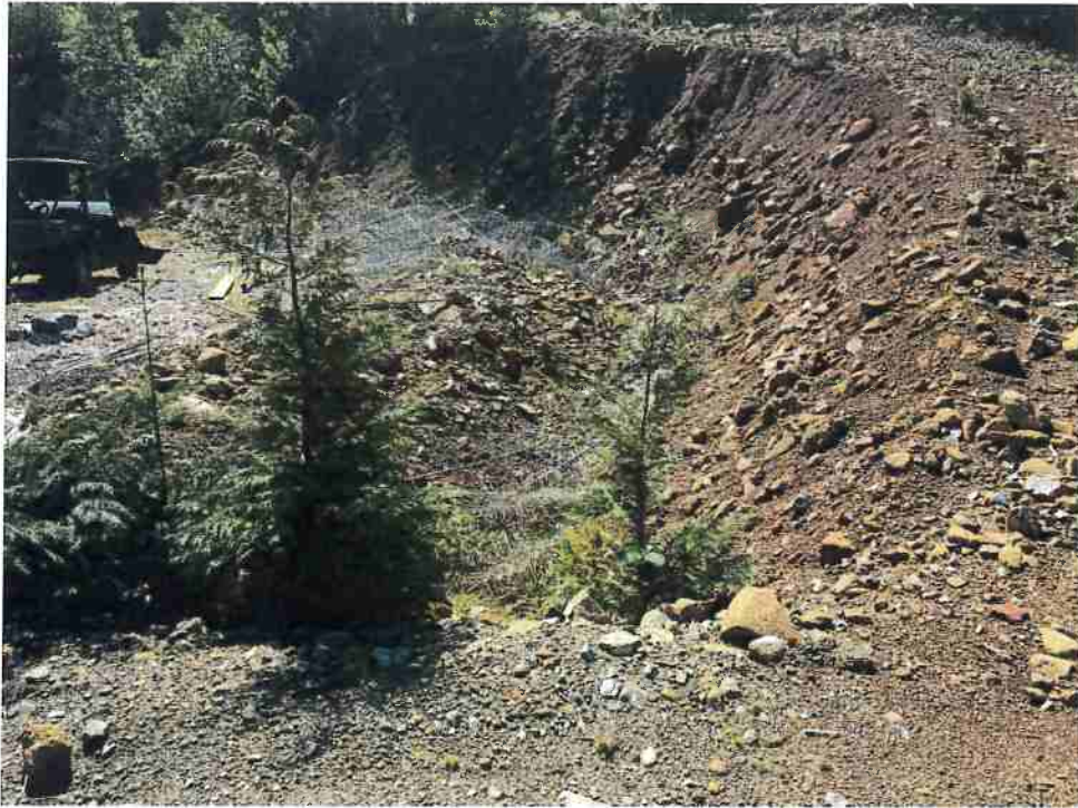
Photo 11. MP13 - Small channel and over-steepened slope.
