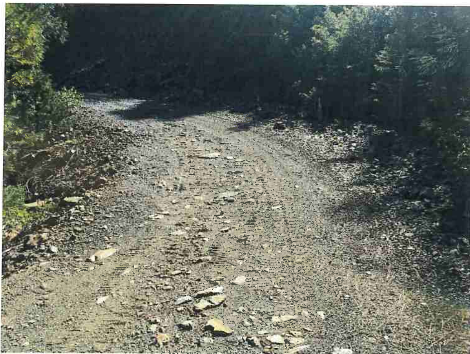
Photo 2. MP6 - Road surface at location of proposed culvert installation.
