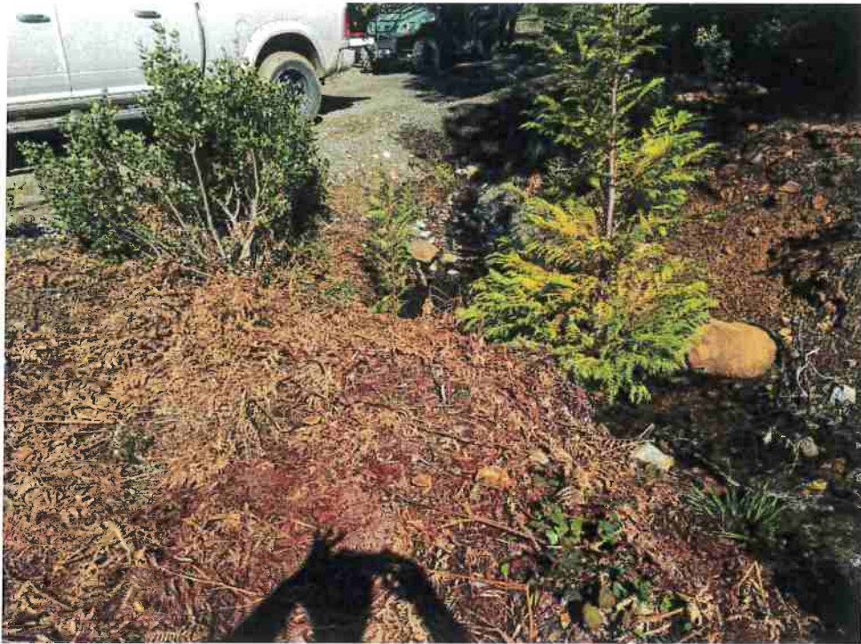
Photo 5. MP8 - Channel upstream from 18" culvert inlet.
