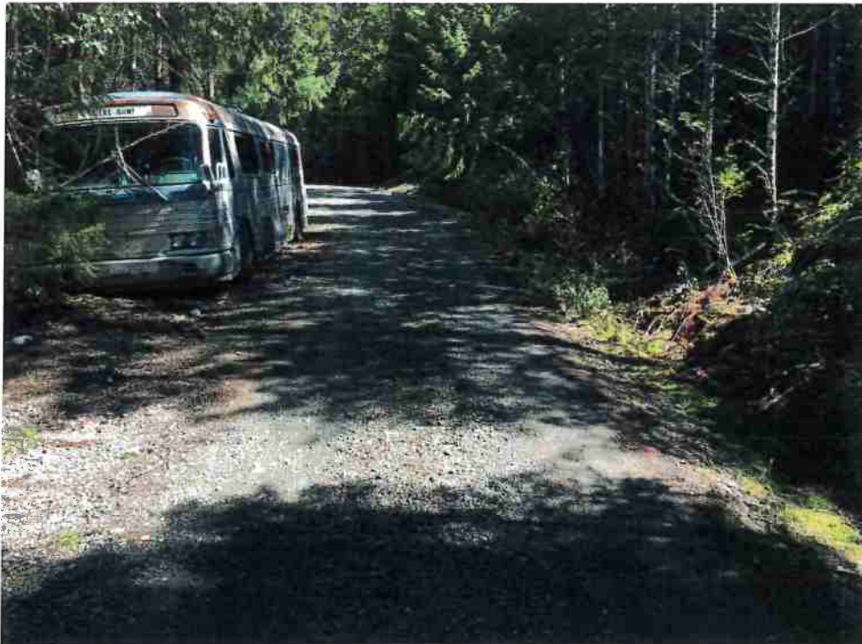
Photo 14. MP20 - Road surface at location of proposed culvert installation.
