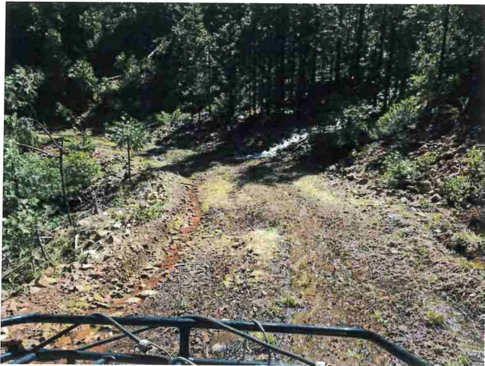
Photo 1. MP4 - Road surface at fill crossing.
