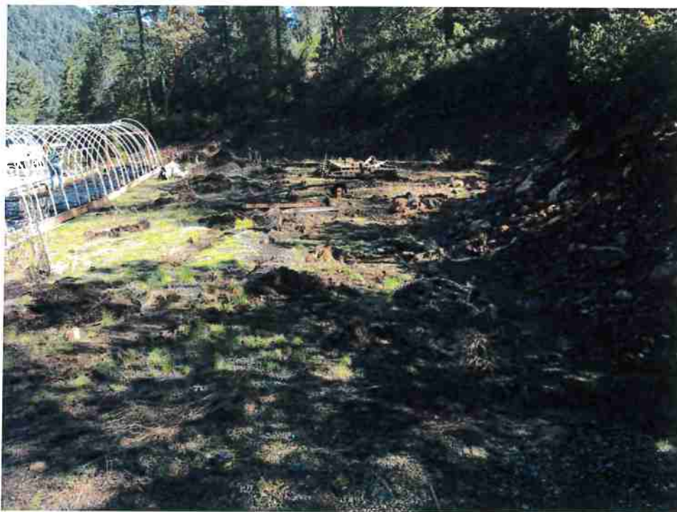
Photo 8. MP8 - Ditch excavated along eastern extent of cultivation flat.
