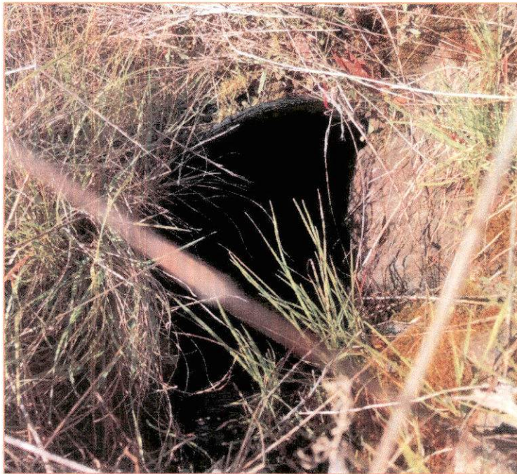
RP13) Clean and maintain DRC inlet.
