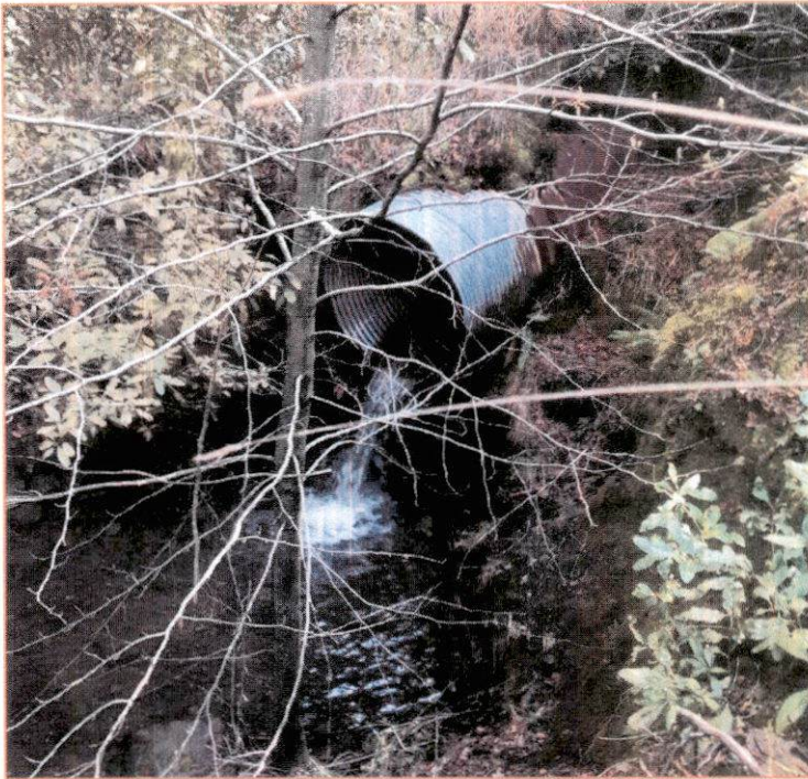
RP7) View of shotgunned outlet on a class II stream.
