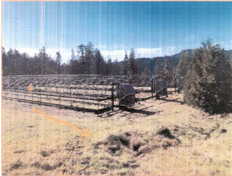
RP12) View of greenhouses from class III stream, note arrows display 50' riparian buffer setback.
