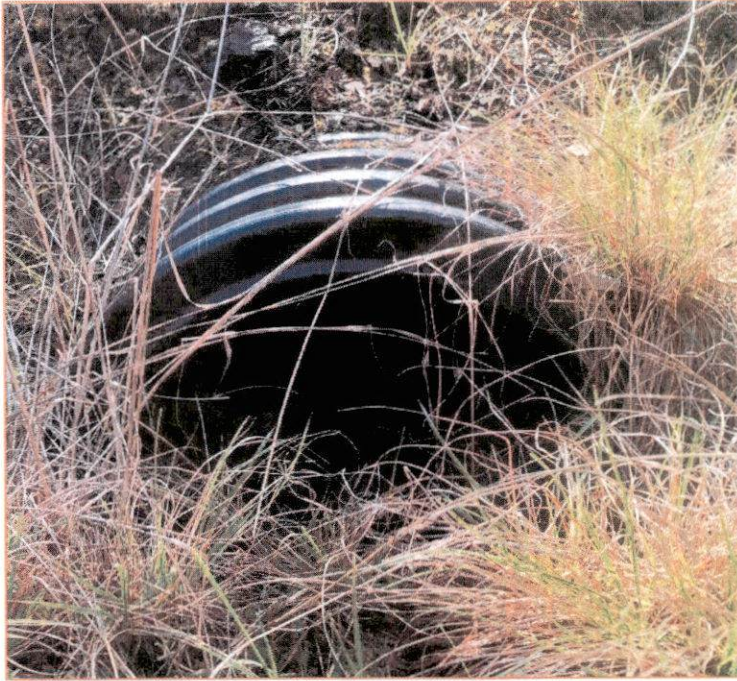
RP9) Clean and maintain DRC inlet.
