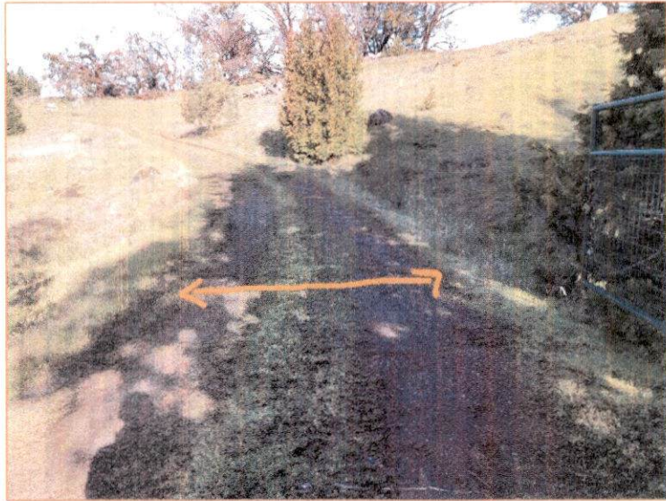
RP1) Install a critical dip.
