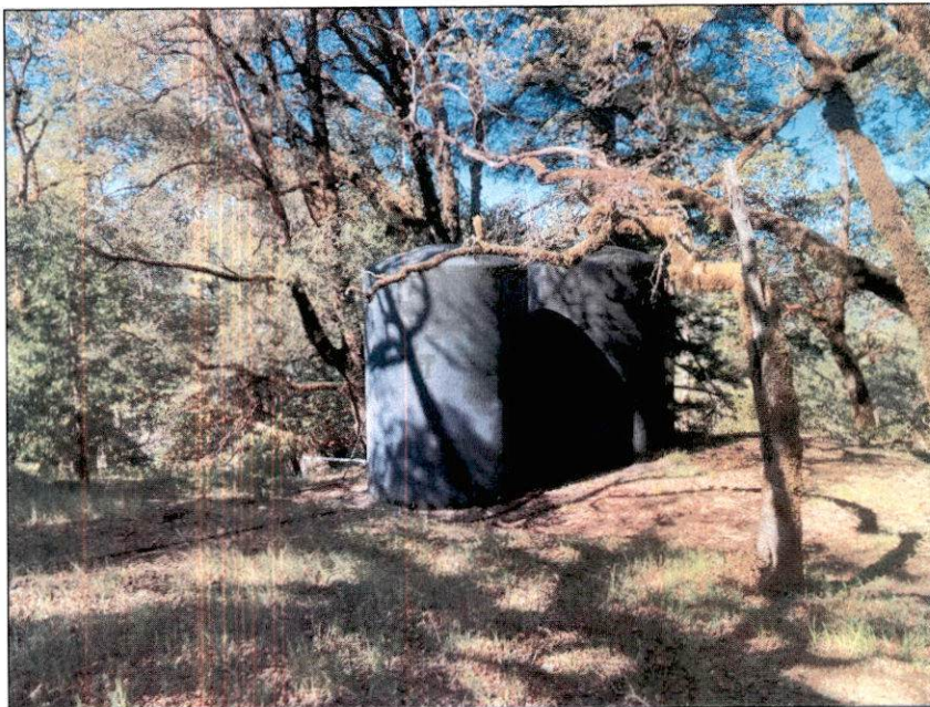
Photos 3 & 4: Existing water tanks for water storage to irrigate proposed cannabis cultivation. April 15, 2021.
