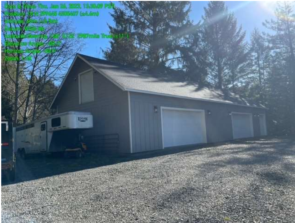
1. West Side of Garage Building at Hedding Property
