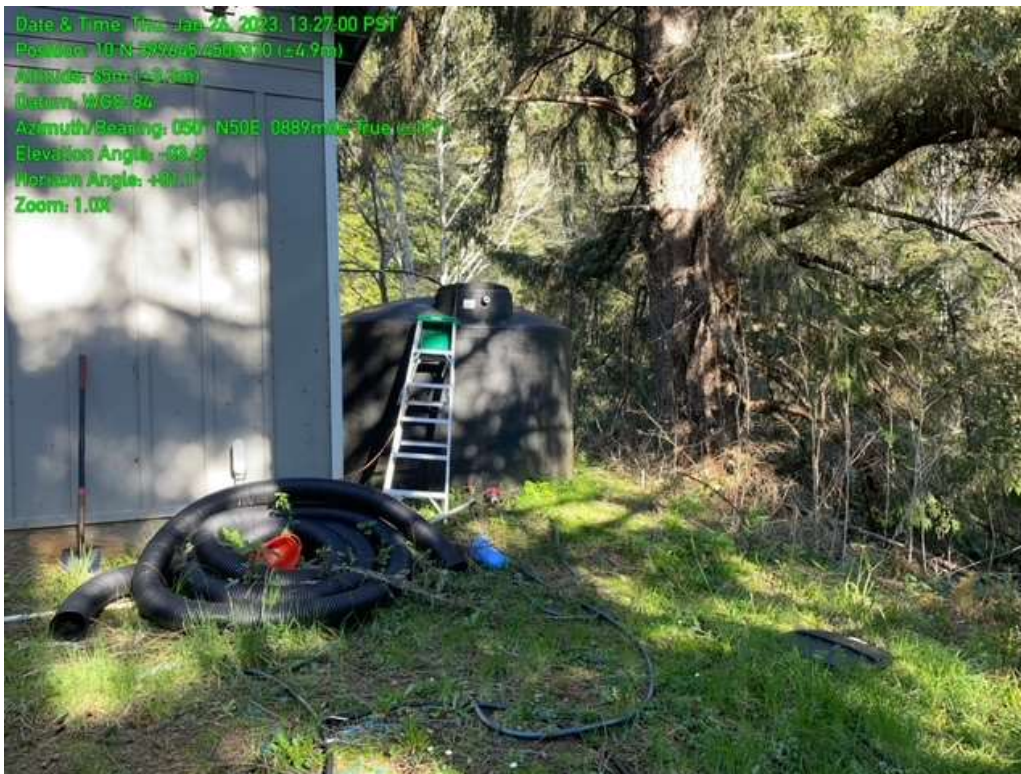
8. View of Southeast Corner of Hedding Garage Building
