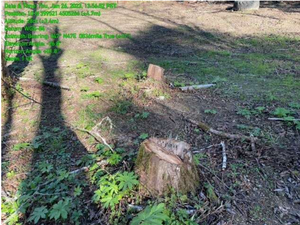
17. Stumps From Tree Removal at Willow Brook creek
