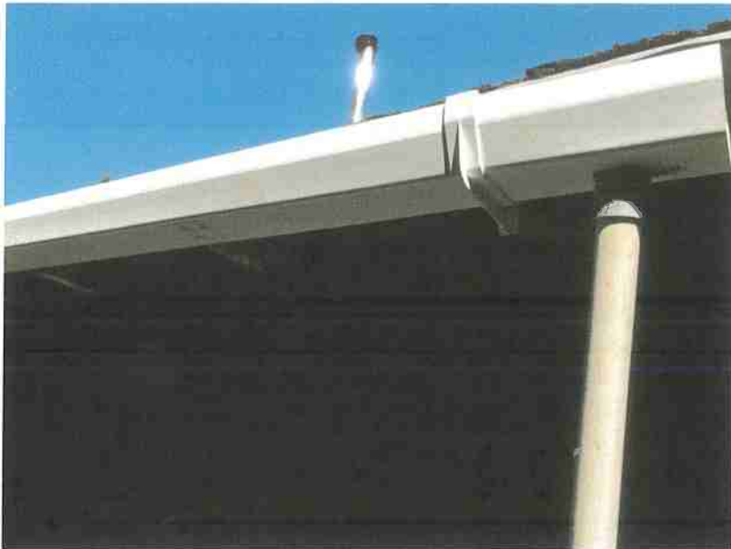
Rain gutter on east side of roof and drain pipe down to irrigation line
