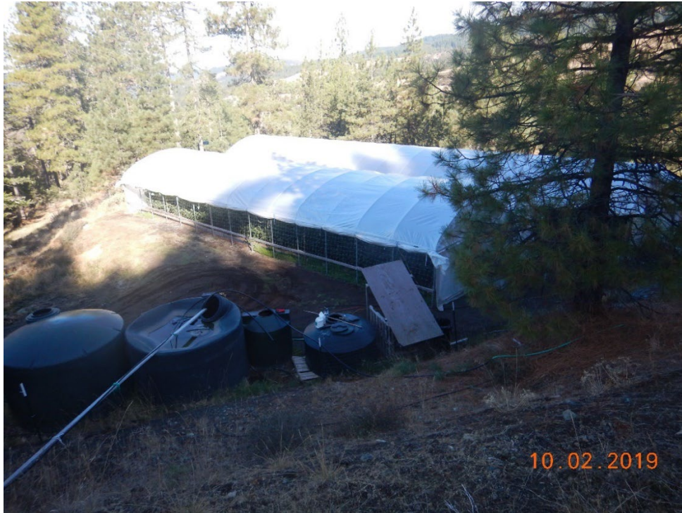
Photo 1. Western greenhouses on APN 210-144-011-000.
