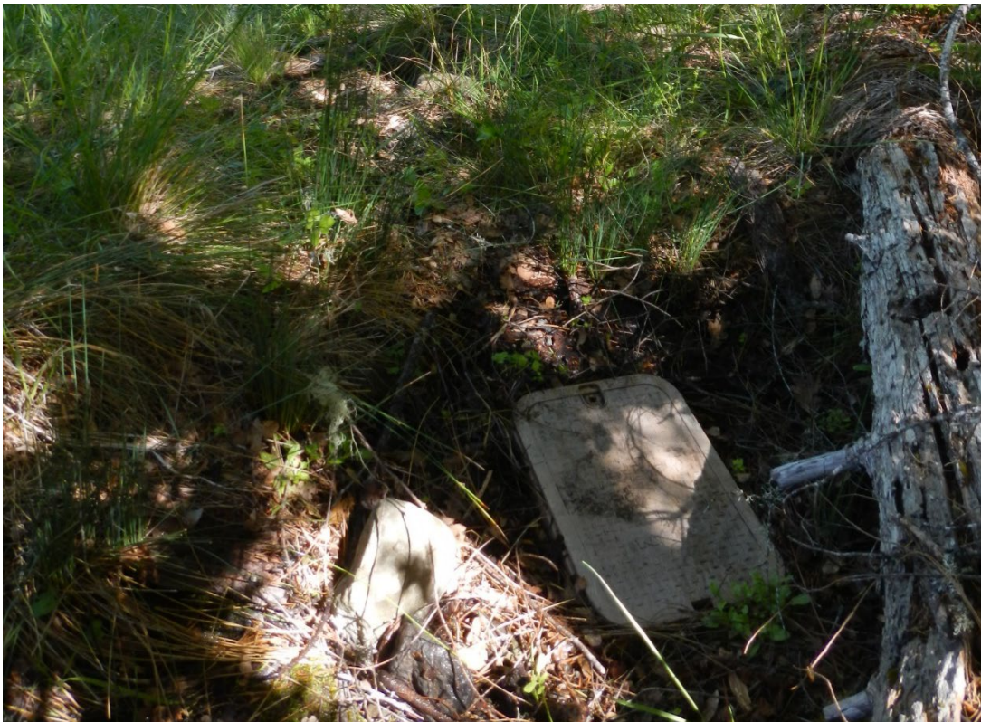
Photo 17. The spring box at POD4. The photo was taken on 6/15/2020.
