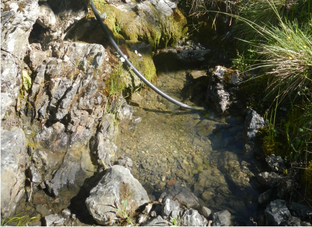
Photo 16. The intake at POD3. The photo was taken on 6/15/2020.
