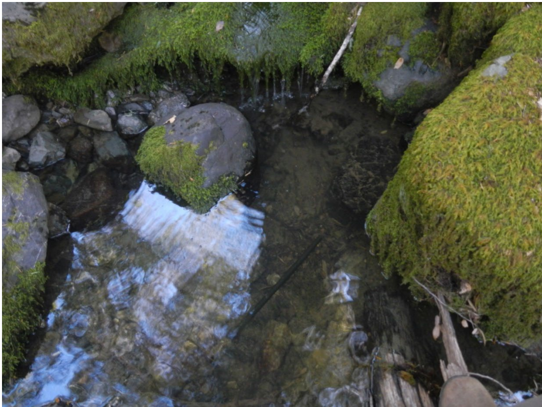
Photo 15. The intake at POD2. The photo was taken on 6/15/2020.
