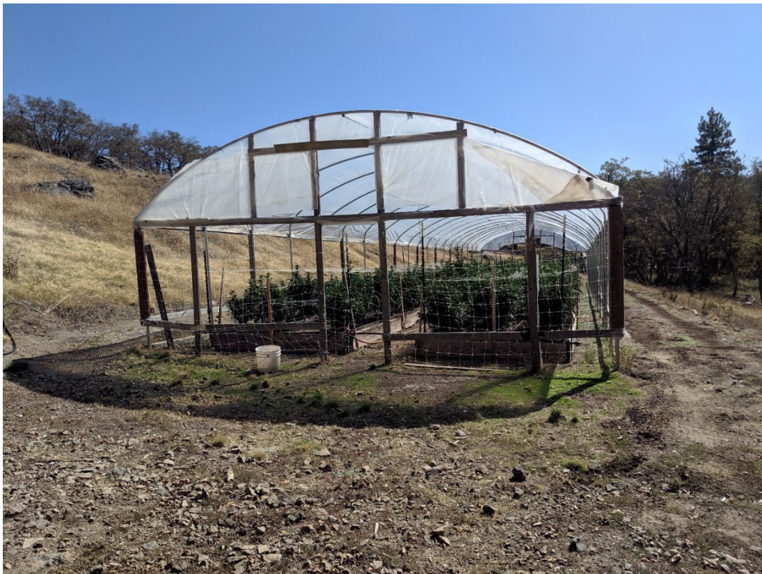
Photo 8. Southeastern greenhouse on APN 210-144-017-000.
