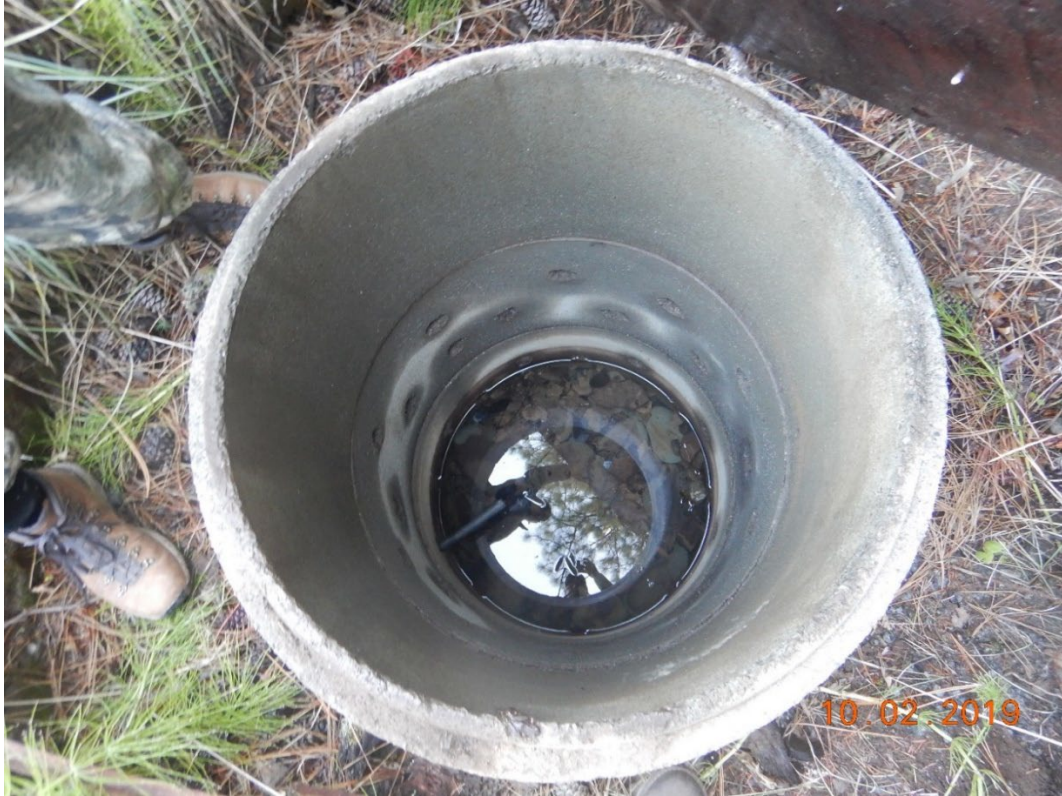
Photo 14. The spring box at POD1.
