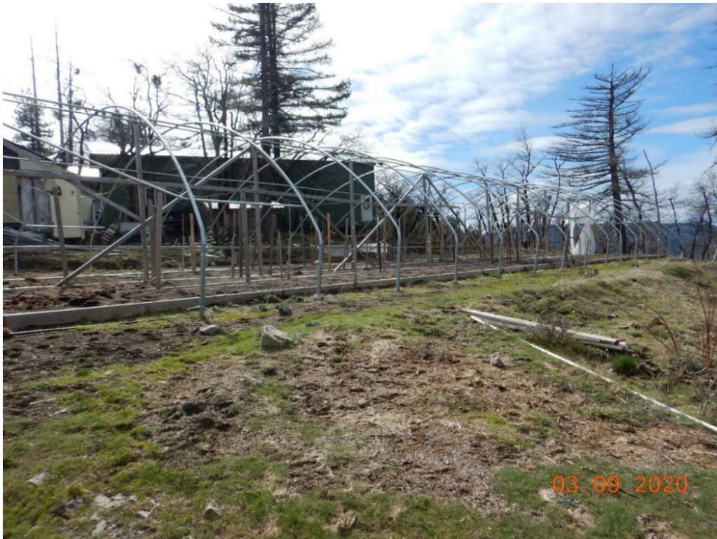
looking at the hoop house from within the riparian buffer.
