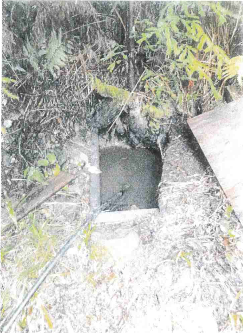
Picture 5: The point of diversion (POD) consists of a wooden box sunken into a seeping hill side. Water is gravity fed using \frac{3}{4} " polypipe to a 50 gallon pickle barrel used as a settling tank. Water is pumped from here to storage tanks throughout the property. Photo date: 03/09/2018
