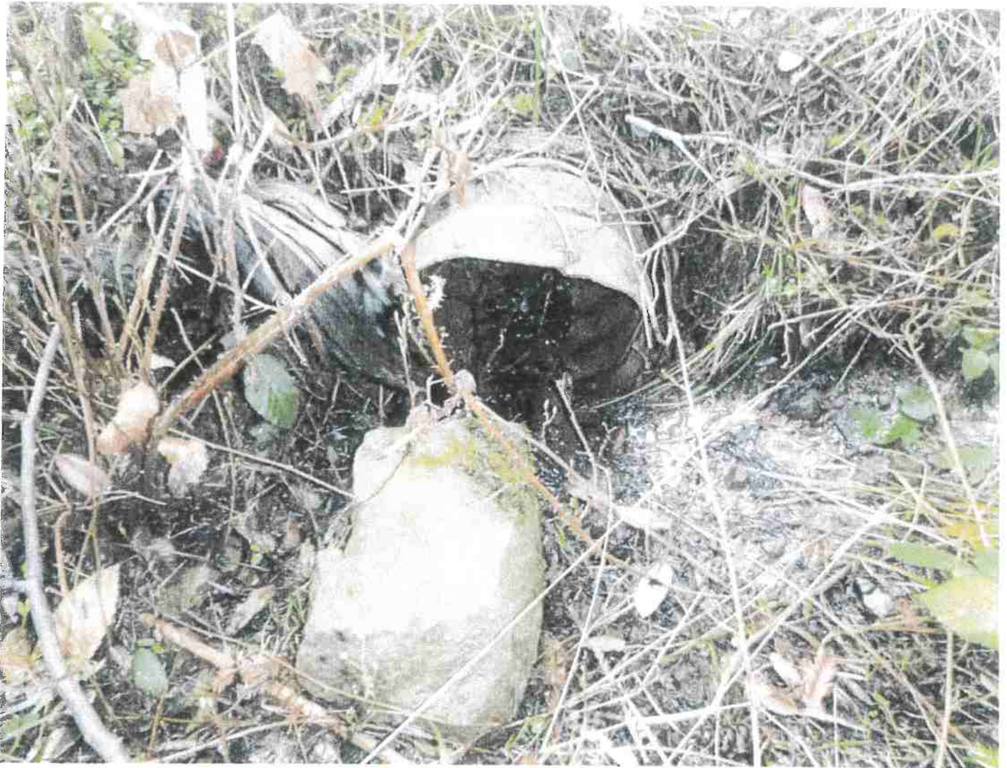
Picture 14: Inlet of 12" diameter relief culvert located at MP #5. Photo date: 03/09/2018
