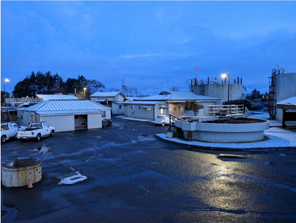
Arcata Wastewater Treatment Facility
