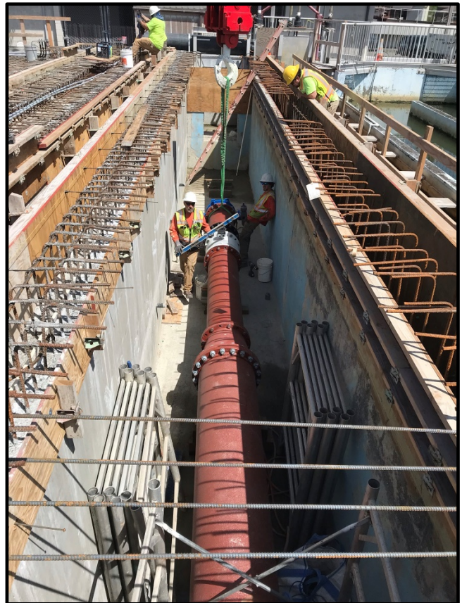
Wastewater Treatment Plant Construction: UV System Construction
