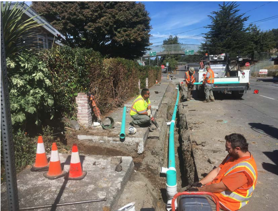
Crew installing new lines on G St
