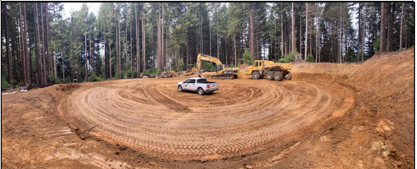
TANK 1 C CONSTRUCTION
