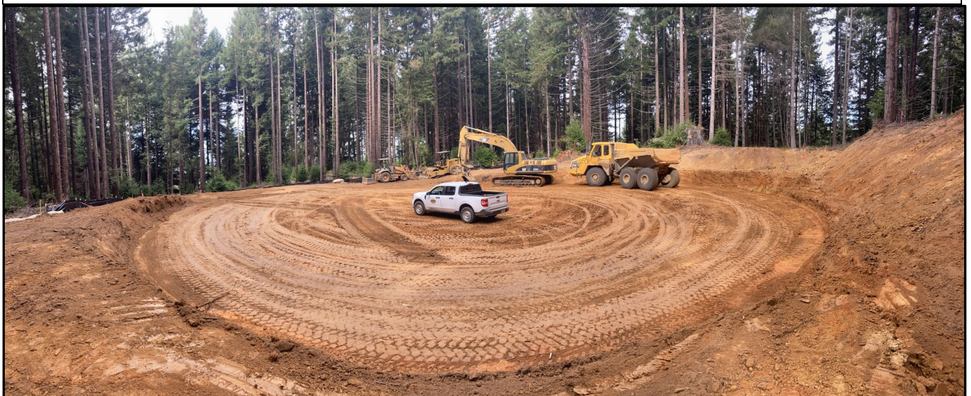
TANK 1 C CONSTRUCTION
