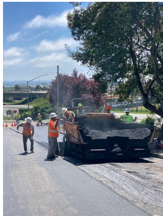
Streets Crew working on the D St. Repaving project.
