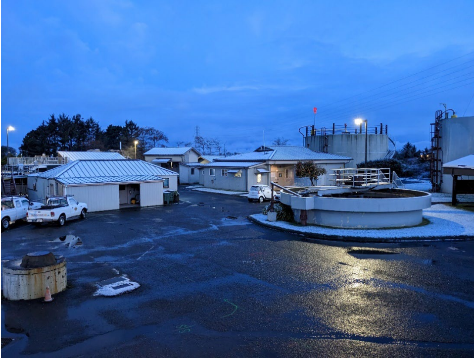
Arcata Wastewater Treatment Facility
