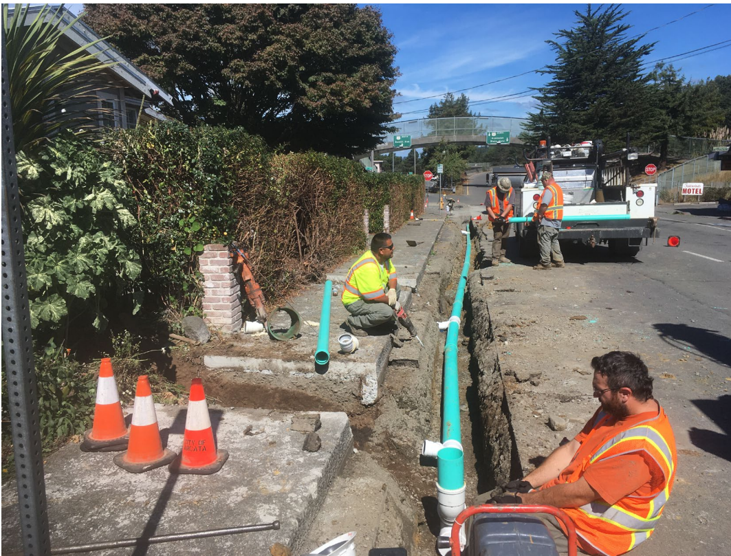
Crew installing new lines on G St
