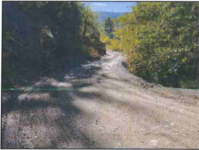
Photo #355 River Rd @ Turnout Location Looking SW @ Curve
