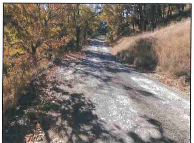
Photo #48 River Rd Looking West @ Turnout
