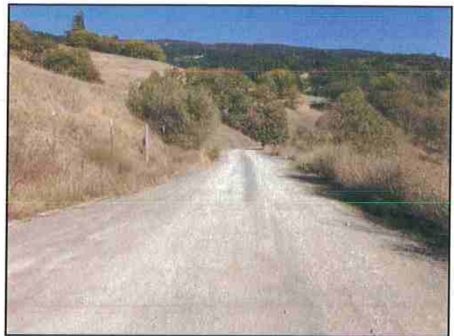
Photo #38 River Rd Looking East
