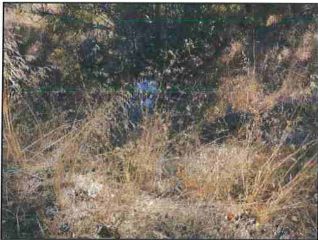
Photo #225 River Rd Looking @ 24" Culvert Out
