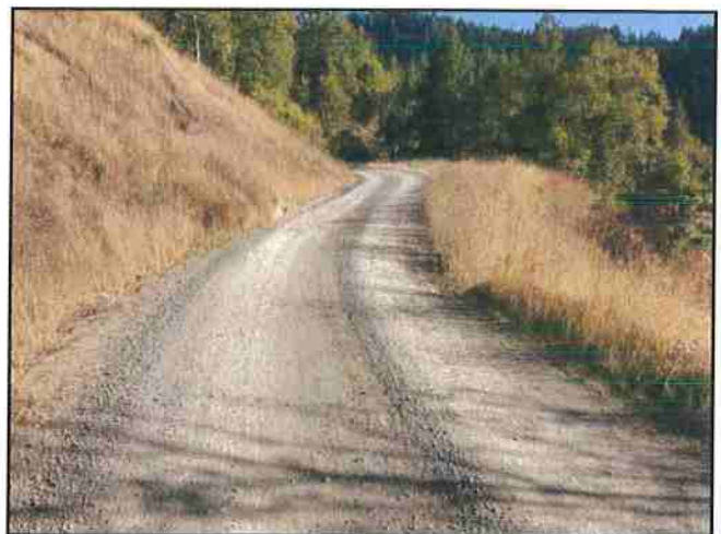
Photo #226 River Rd Looking SE @ Curve w/ Pullout
