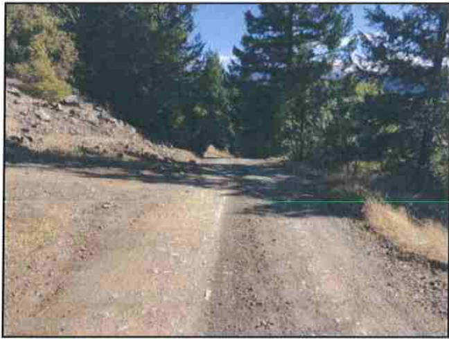
Photo #385 River Rd @ Turnout Location Looking SE
