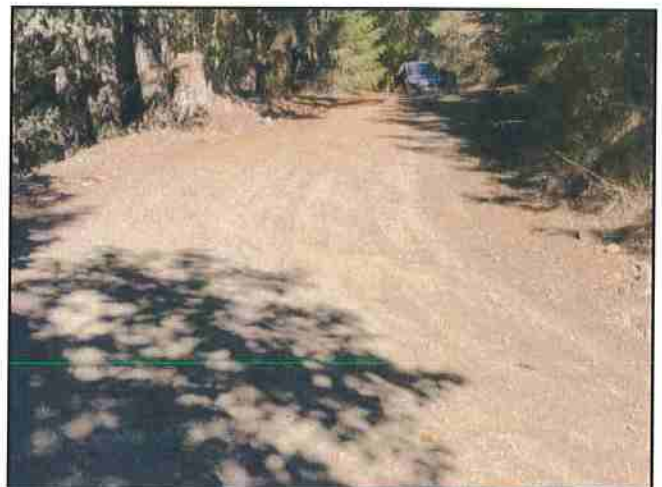
Photo #346 River Rd @ Turnout Location on-Curve Looking NE
