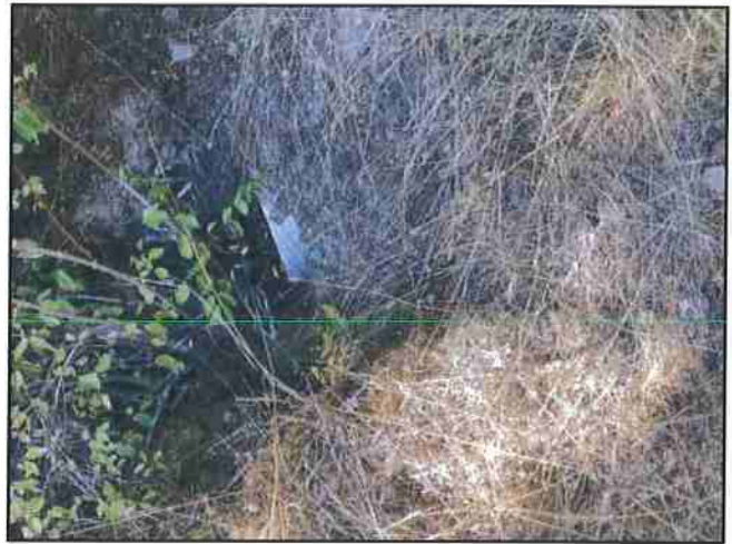
Photo #302 River Rd Looking @ 24" Culvert Out
