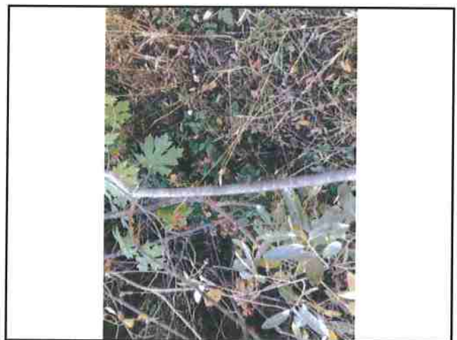
Photo #204 River Rd Looking @ 12" Culvert Out
