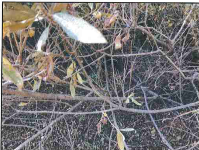
Photo #203 River Rd Looking @ 12" Culvert In
