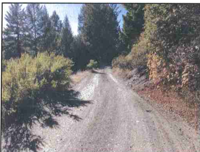
Photo #359 River Rd Looking SW
