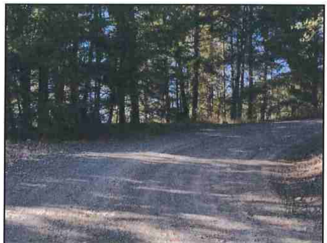
Photo #306 River Rd Looking NW @ Curve w/ Turnout
