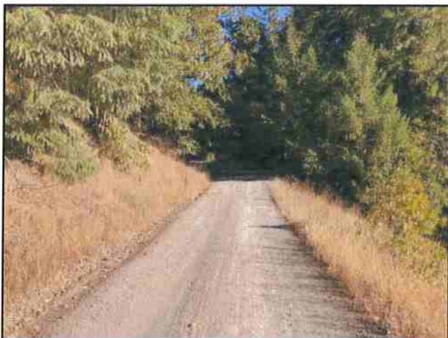
Photo #209 River Rd Looking SE @ Curve w/ Turnout
