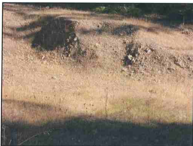
Photo #311 River Rd Looking @ Hillside Slip
