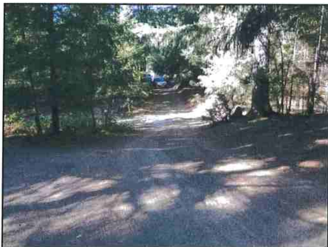
Photo #437 River Rd @ Curve w/ Turnout Looking NW
