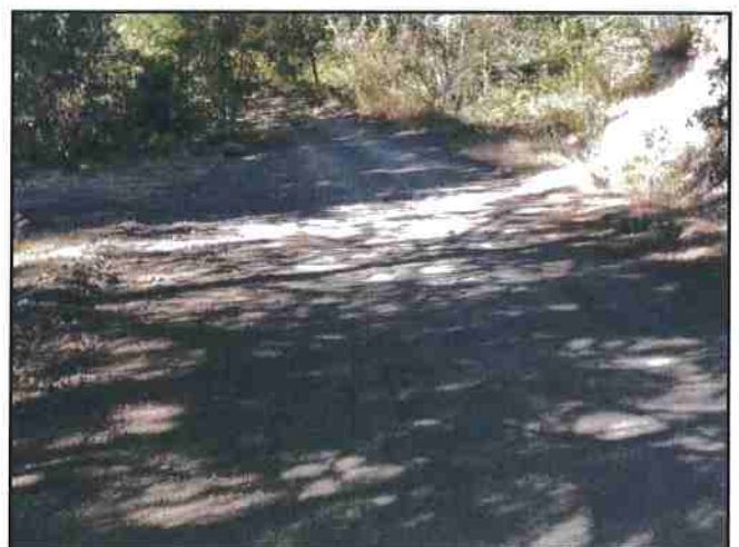
Photo #150 River Rd Looking NW @ Curve w/ Turnout
