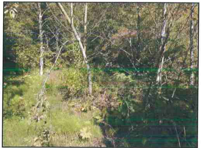
Photo #152 River Rd Looking @ 24" Culvert In
