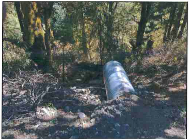
Photo #178 River Rd Looking @ 36" Culvert Out
