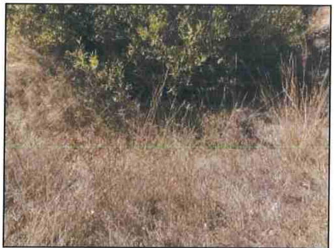
Photo #410 River Rd Looking @ 24" Culvert Out
