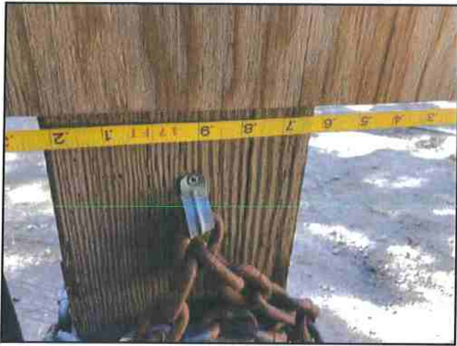
Photo #124 Private Access Rd APN 208-221-014 Gate Width 17'
