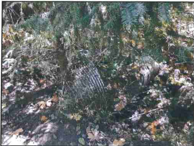
Photo #153 River Rd Looking @ 36" Culvert Out
