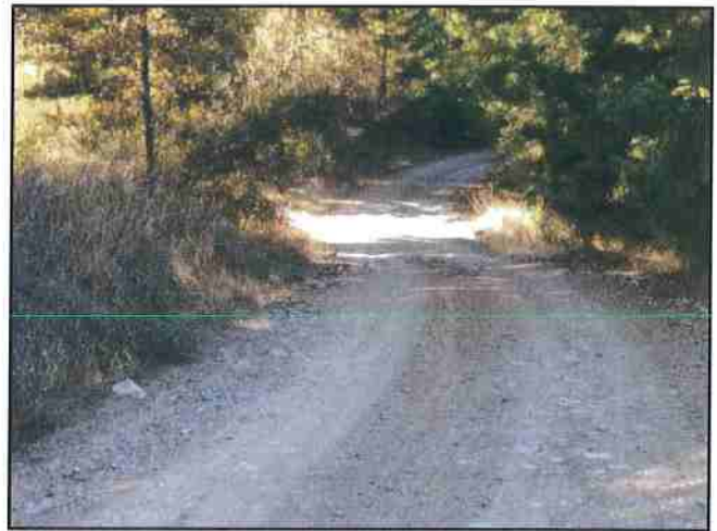
Photo #314 River Rd Looking South @ Curve w/ Turnout
