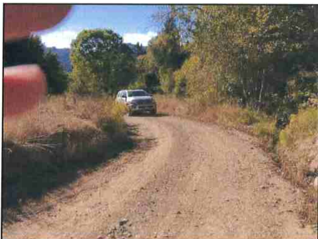
Photo #425 River Rd @ Curve w/ Turnout Looking SW
