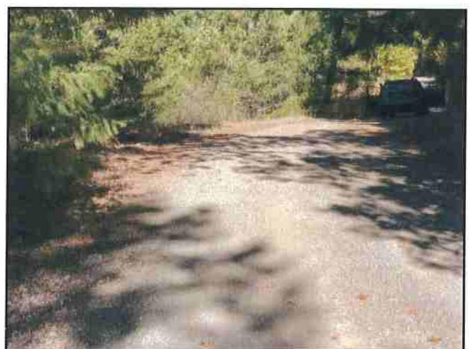
Photo #264 River Rd Looking NW @ Curve w/ Turnout
