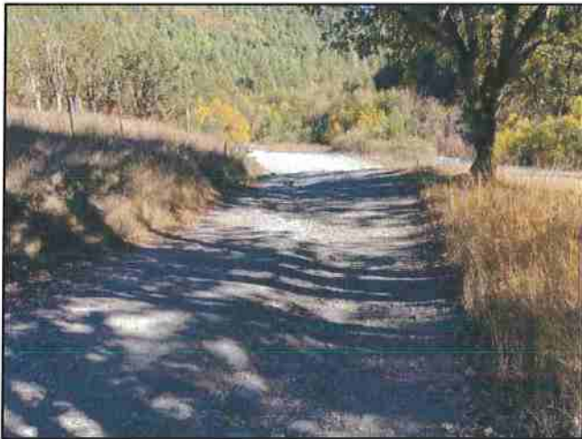
Photo #9 River Rd Looking SE @ Curve w/ Turn-out
