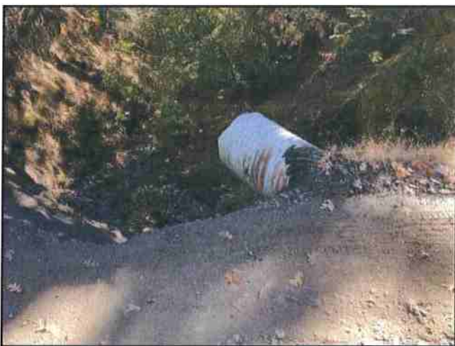
Photo #89 River Rd Looking @ 24" Culvert Out
