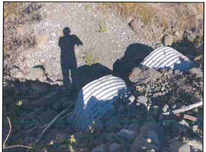
Photo #16 River Rd Looking @ Dual 36" Culverts Out
