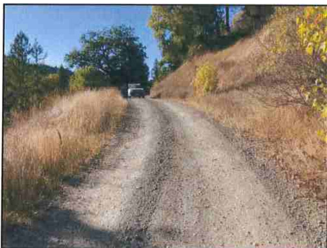
Photo #227 River Rd Looking NW @ Curve w/ Pullout
