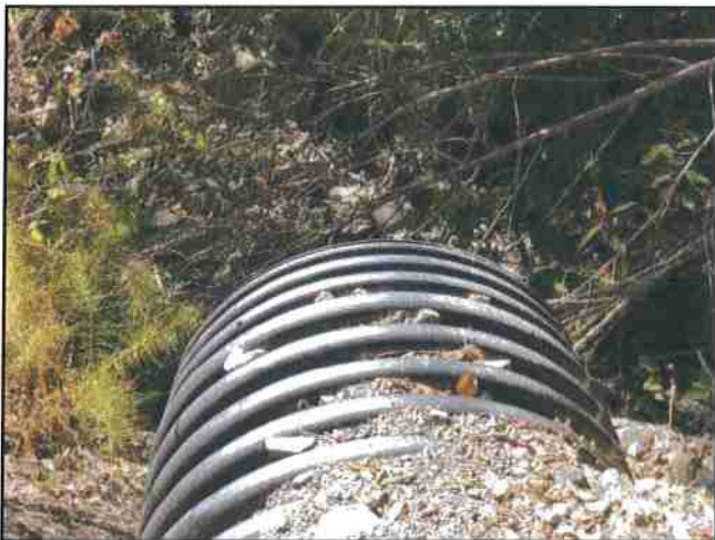
Photo #279 River Rd Looking @ 24" Culvert Out
