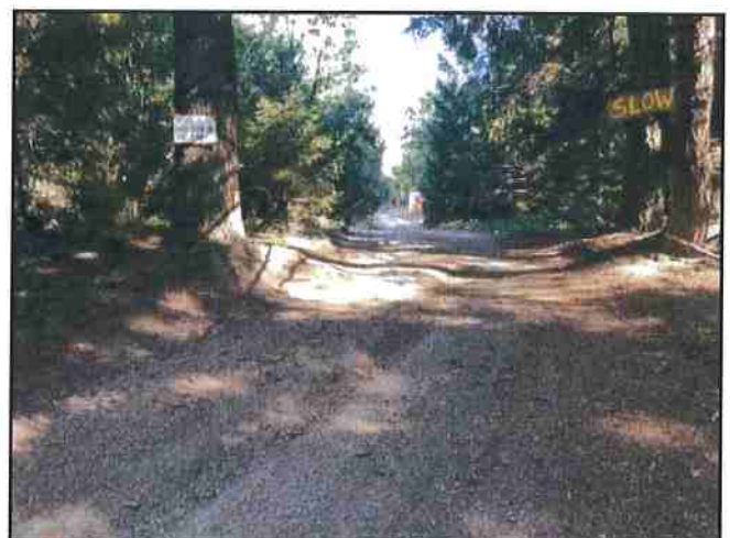
Photo #438 River Rd @ Curve w/ Turnout Looking SE
