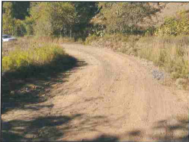
Photo #423 River Rd @ Curve w/ Turnout Looking SW
