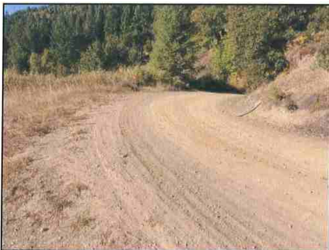
Photo #419 River Rd @ Curve w/ Turnout Looking NW
