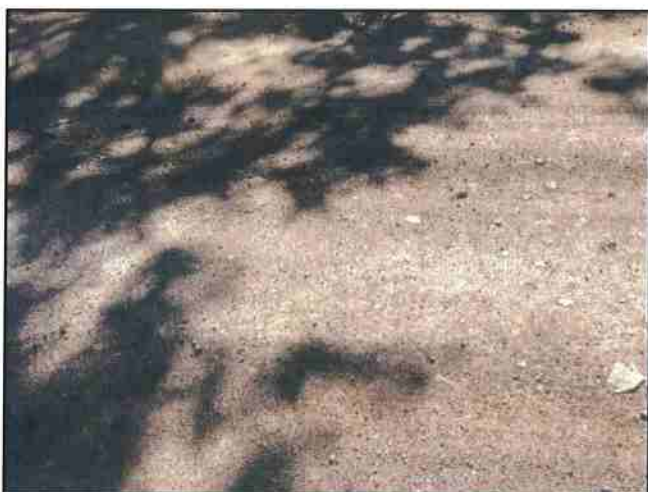
Photo #143 River Rd Looking @ Drainage Path Over Road
