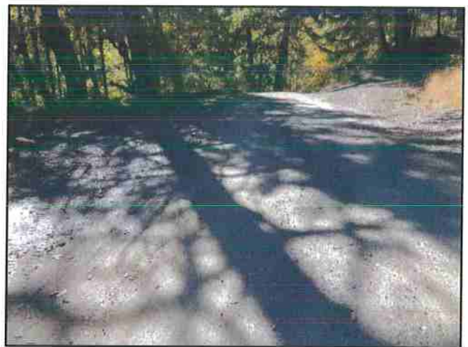
Photo #92 River Rd Looking SW @ Turnout, Approach, & Curve
