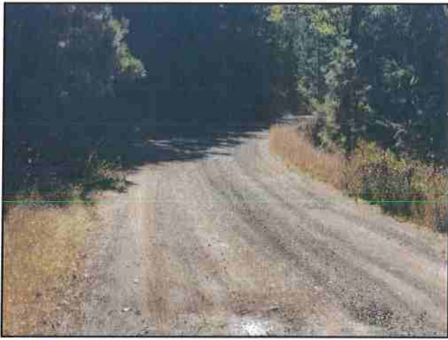
Photo #271 River Rd Looking South @ Curve w/ Turnout
