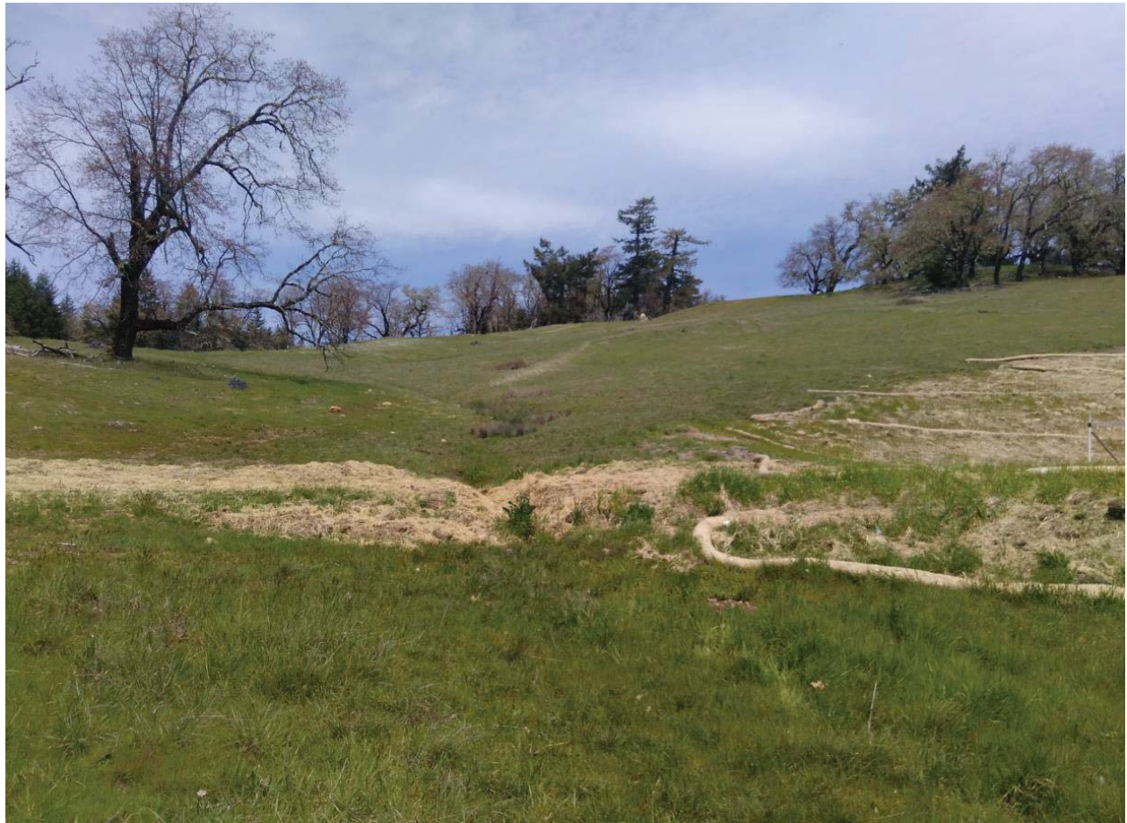
View of Class III water course. Also in view are the decommissioned access road to CA-3 and the site of the removed culvert. Retake of OP-6
