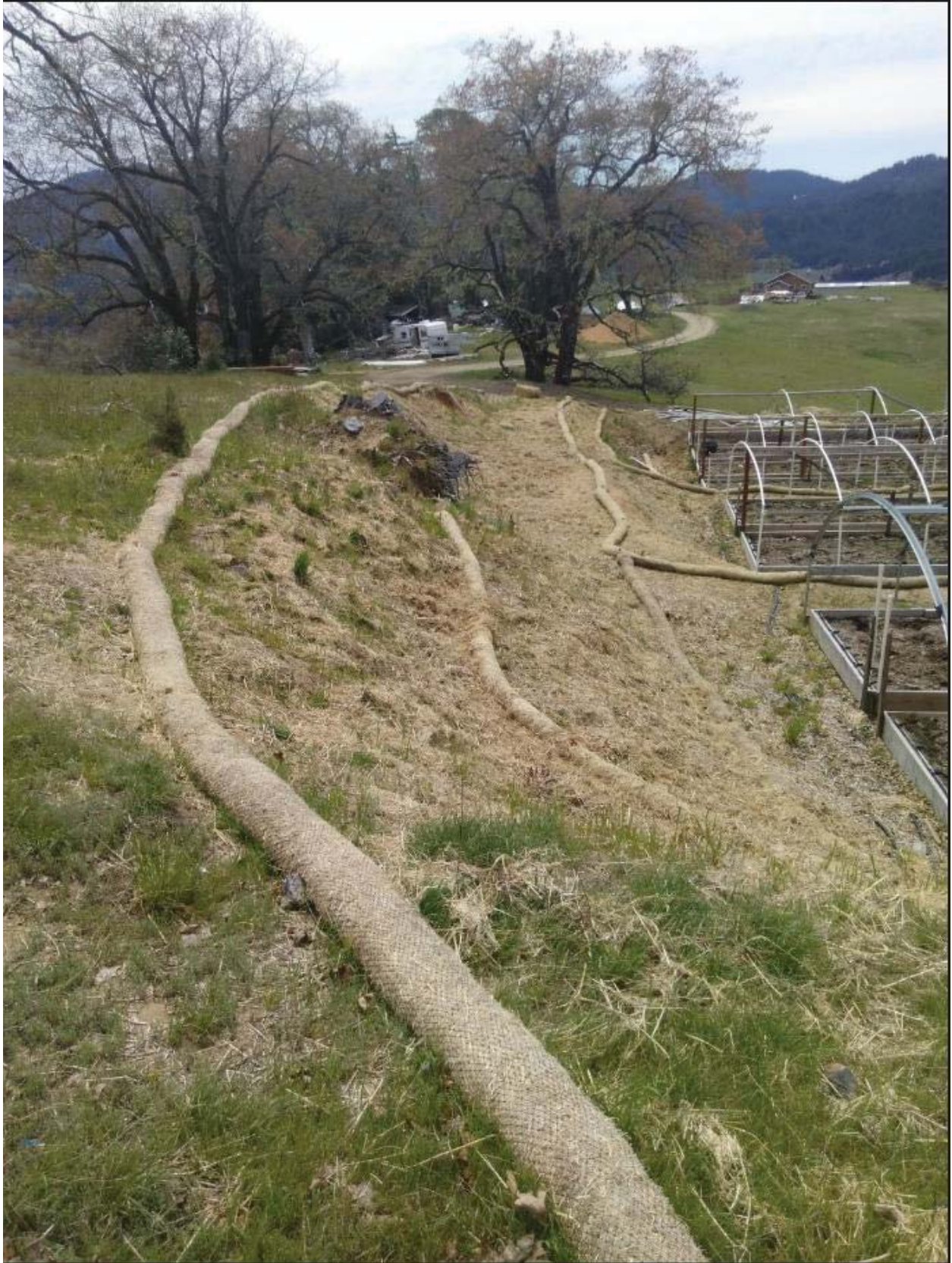
NE corner of CA-2 showing adequate installation of straw and waddles.
