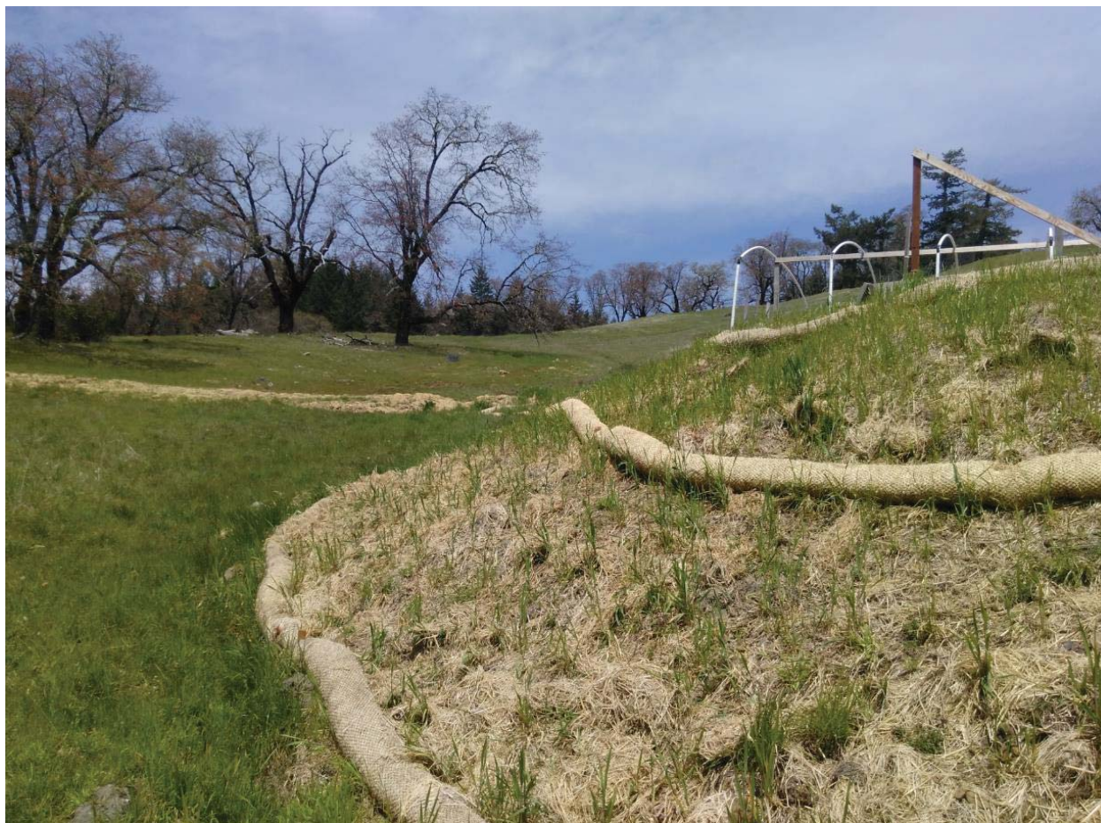
SW corner of CA-3 showing strawing and waddles installed. Drainage for Class III is in lower left corner of photo, not a very defined channel, very vegetated, waddle installed in channel. Retake of OP-4
