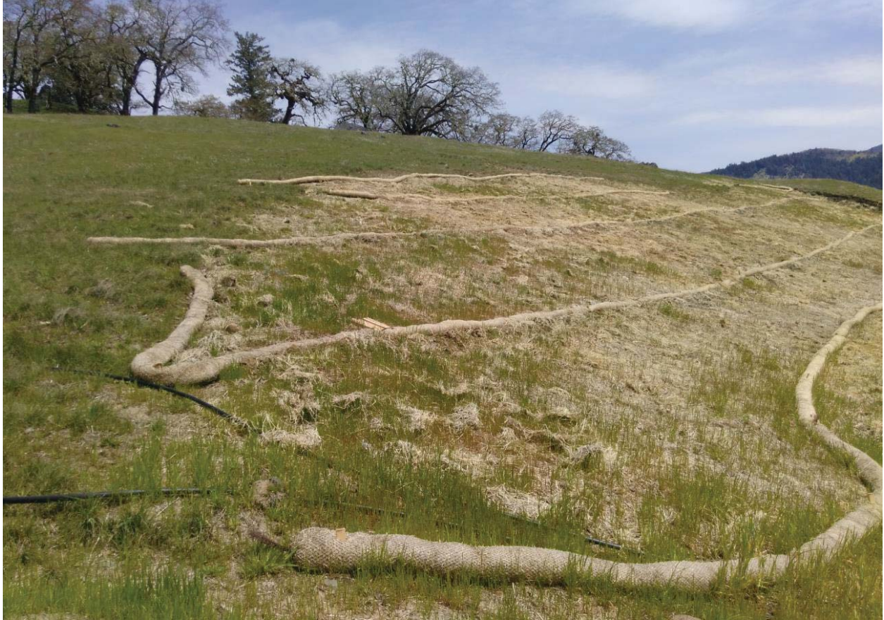
Waddles and straw installed on disturbed earth above CA-3
