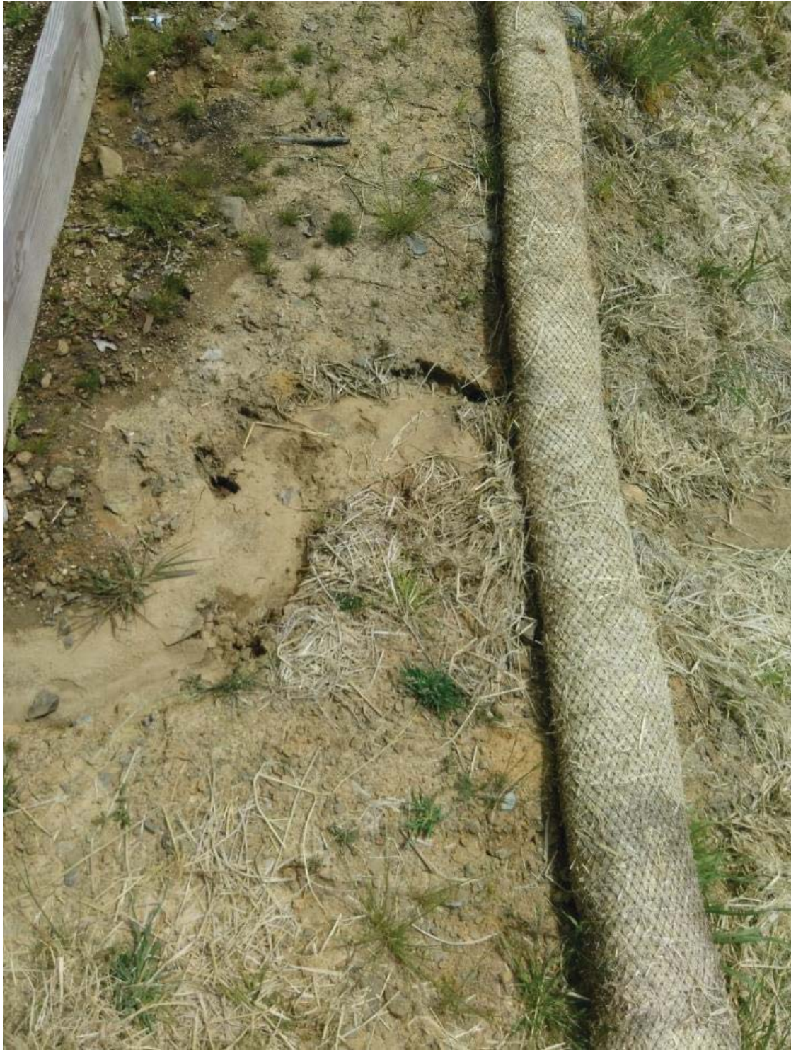
Close up of wattle installed in CA-2
