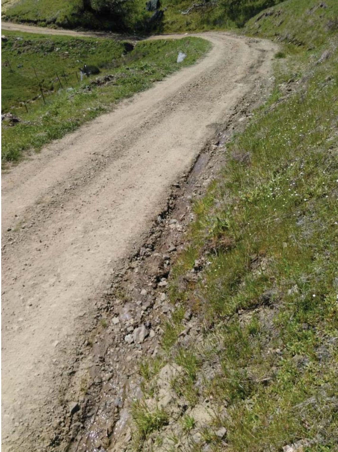
Road segment to be improved and hydrologically disconnected. CV-2 is visible in the background at the bend in the road.
