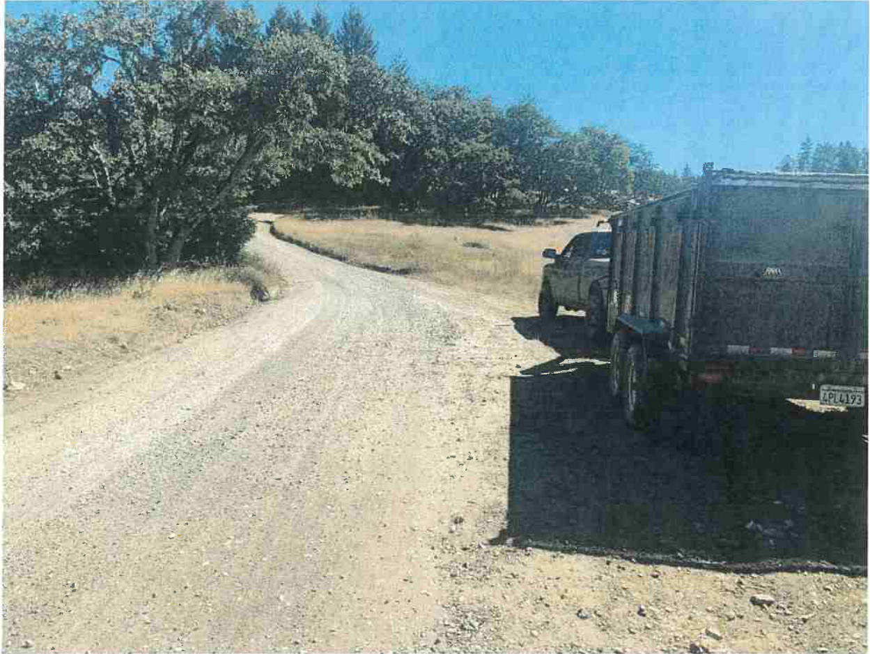
Mm —.25. Photos 2/3 large pull out and recently graded road with new ditches for proper water drainage
