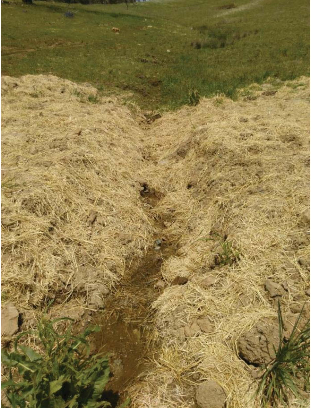
Site of removed 4" culvert at CA-3
