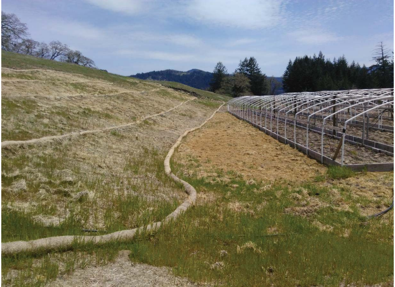
Another view of the revegetation progress on the cut slope above CA-3
