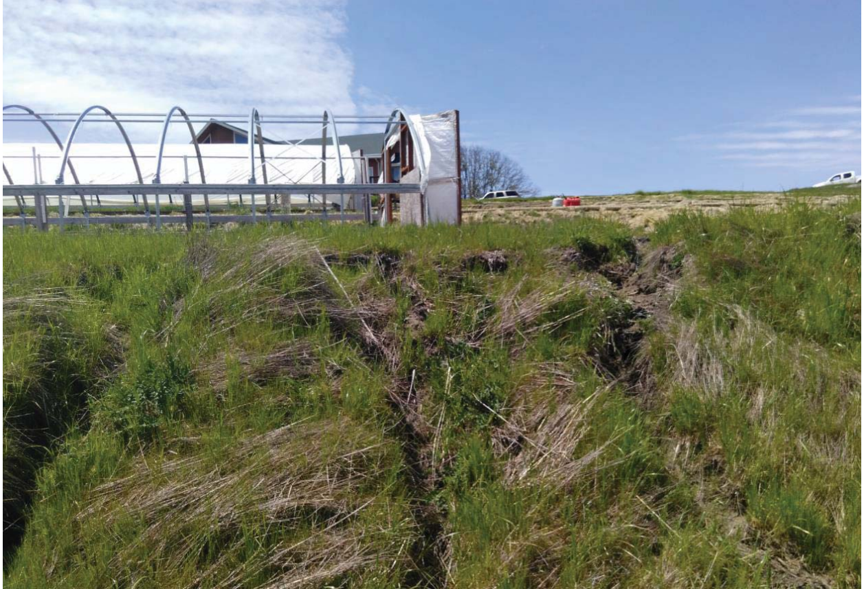
Ruts and revegetation at the lowest slope of the terrace at CA-5
