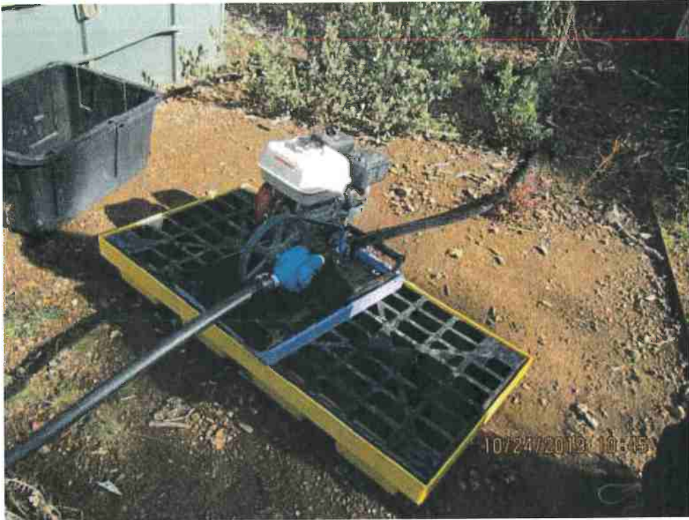
Photo 3. Pump needing secondary containment
