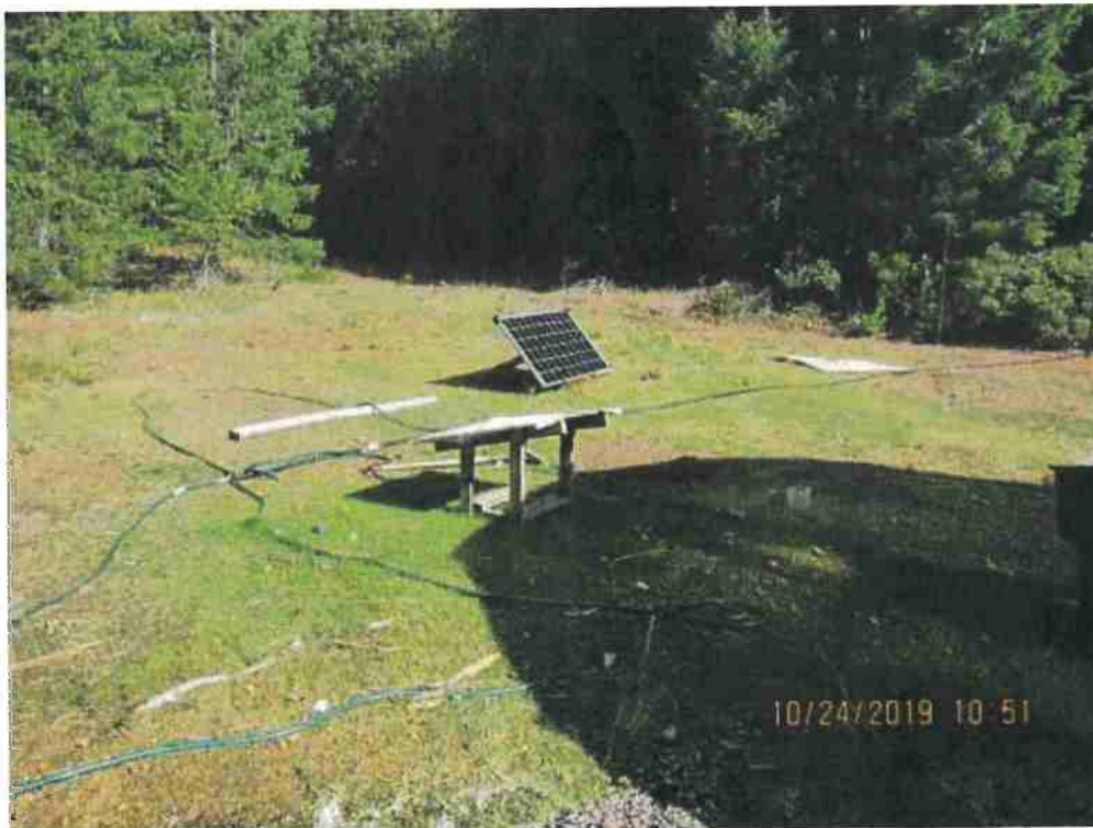
Photo 4. Solar panel near bladder
