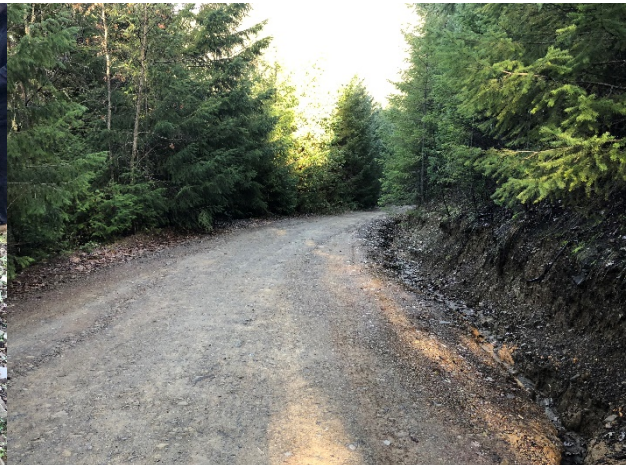
Picture #4 Cobb Rd @ curve looking NW
