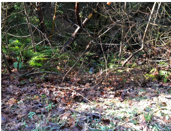
Picture #47 Cobb Rd outlet of 12" culvert in Picture 46
