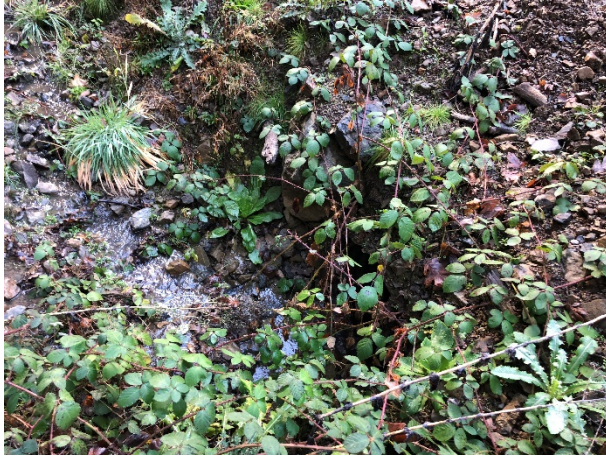
Picture #7 Cobb Rd @ 12" CMP inlet at curve
