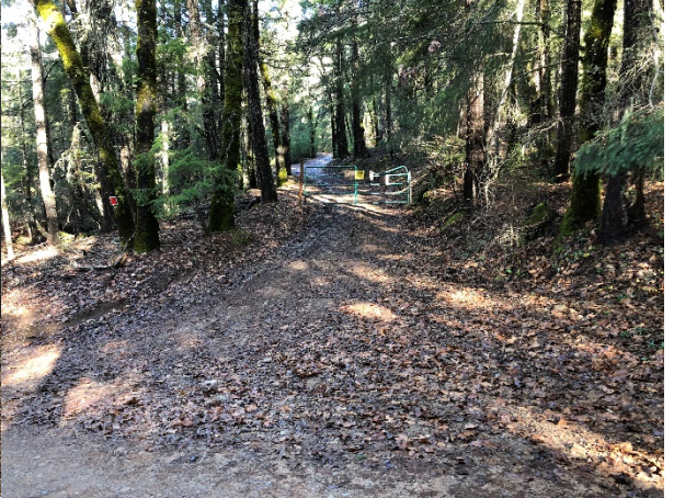
Picture #34 Cobb Rd looking N. @ driveway w/ erosion
