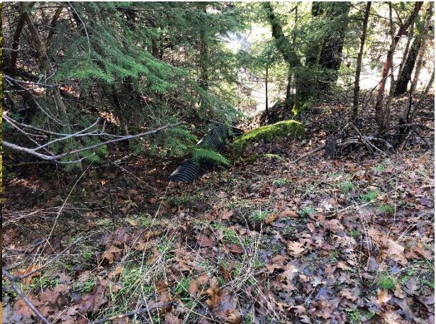
Picture #18 Cobb Rd @ 18" culvert outlet looking W @ esmt.
