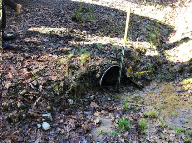
Picture #26 Cobb Rd inlet of 12" culvert in Picture 27.
