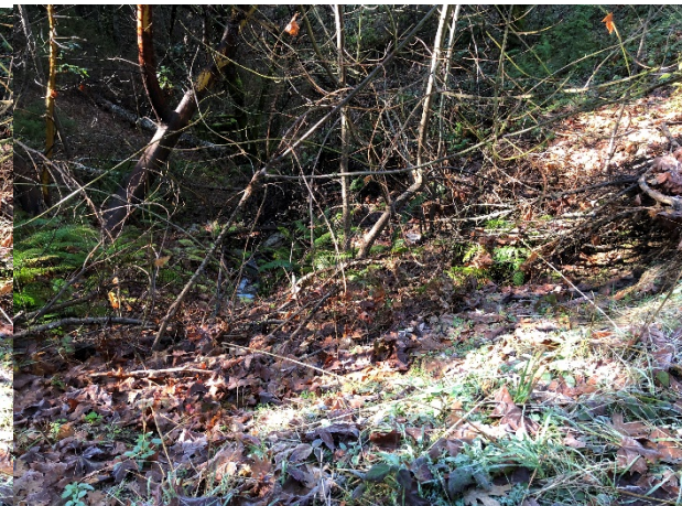
Picture #48 Cobb Rd outlet of 12" culvert in Picture 46
