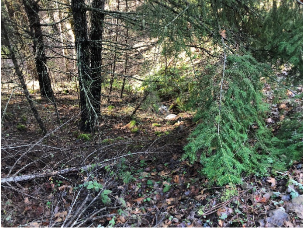
Picture #31 Cobb Rd 12" culvert outlet
