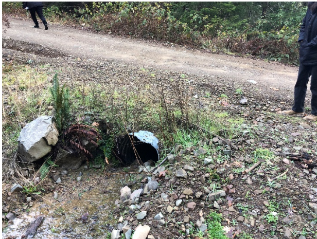
Picture #3 Cobb Rd at Curve in Picture #2 looking @ 12" CMP
