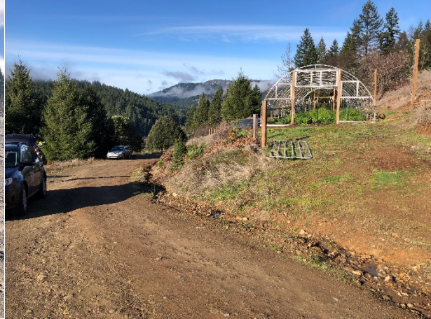
Picture #14 Cobb Rd looking SW towards curve.
