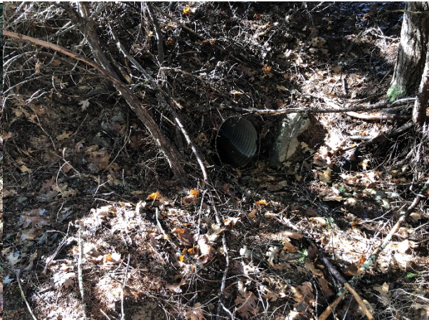
Picture #42 Cobb Rd looking @ inlet of 12" culvert
