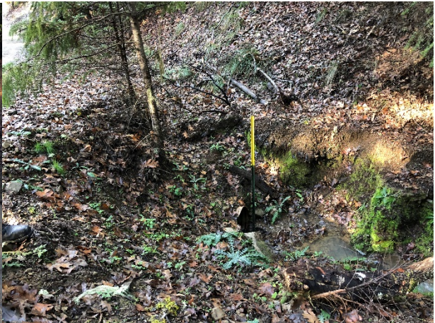
Picture #30 Cobb Rd 12" culvert inlet
