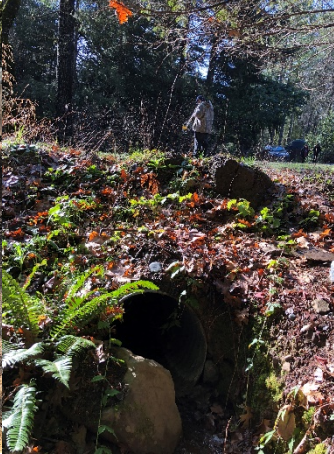
Picture #40 Cobb Rd looking @ 12" culvert inlet
