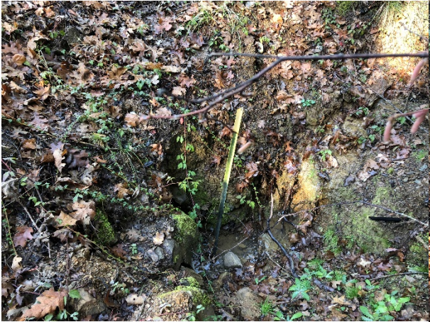
Picture #21 On PG&E esmt looking NE @ outlet from Cobb Rd
