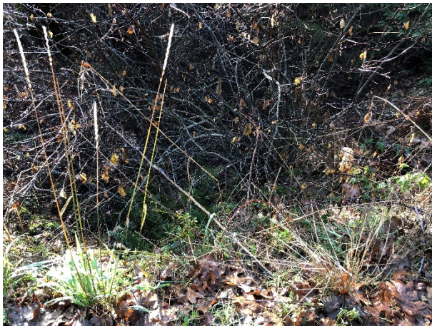
Picture #41 Cobb Rd looking @ outlet of 12" culvert in Picture 40
