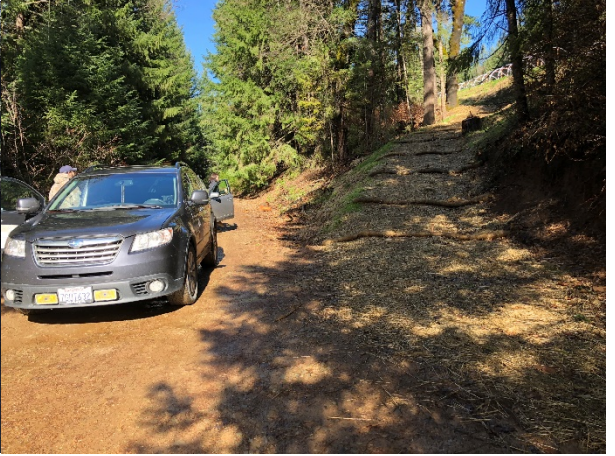
Picture #52 Cobb Rd looking NW towards properly stabilized slope
