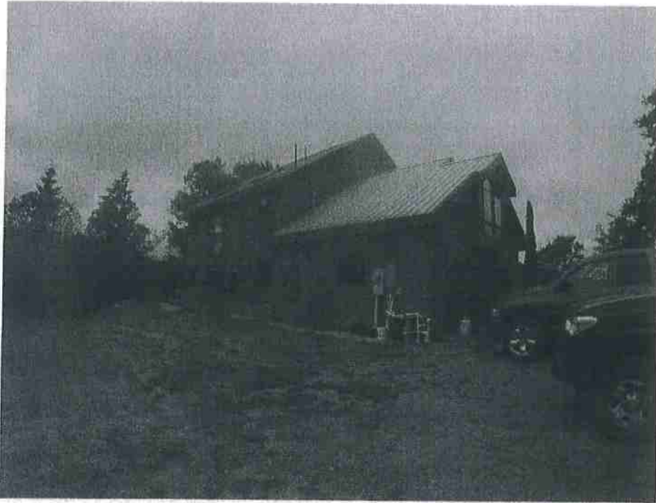
Primary residence: This residence has a permitted septic system.
