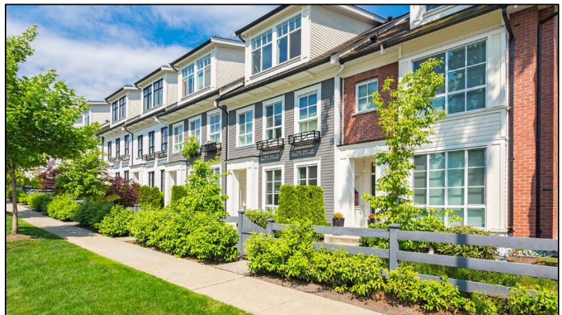
Entrances to individual units facing the street
