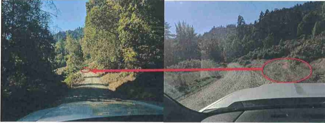
Figure 10: Pinch point and turnout area along RS #5
