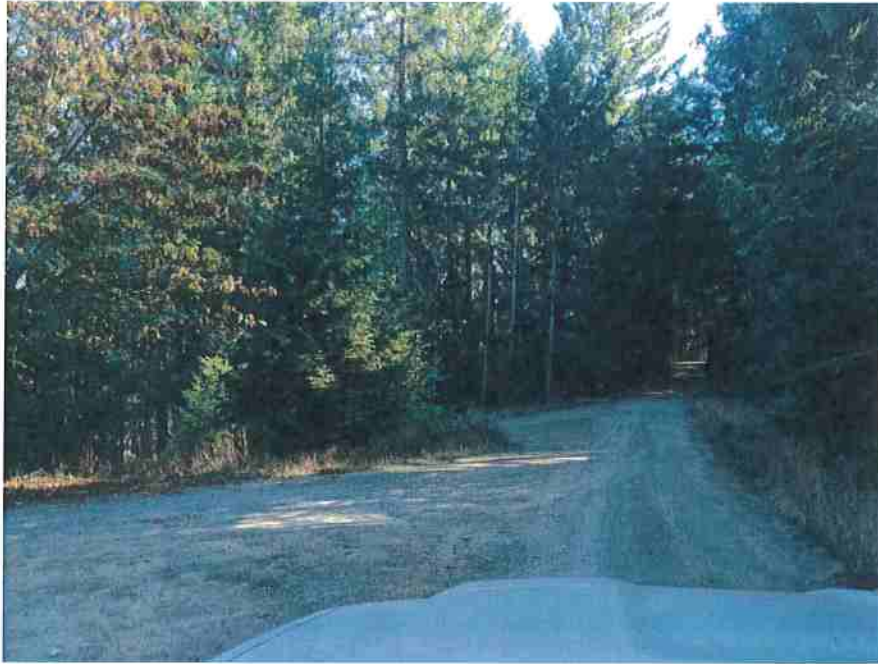
Figure 21: Road segment #10 ground view heading South with turnout to the left.
