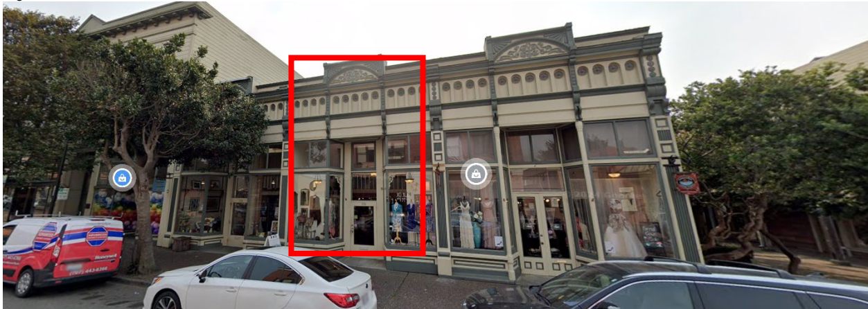
Figure 3: Second Street Façade - 326 Second Street (APN 001-093-004)
