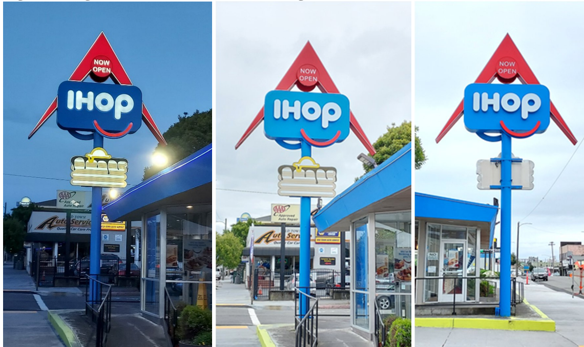
Figure 4: Sign Installed Without a Building Permit (4/12/2024)
