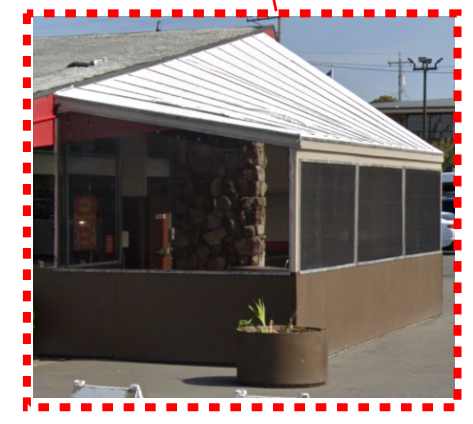
Existing Patio to be demo'd
