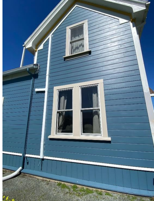
Figure 5: View of the renovated southern-facing façade using cedar for the siding, trim, skirting, and roof eave and new double-hung fiberglass exterior and wooden interior windows, photo taken January 2024
