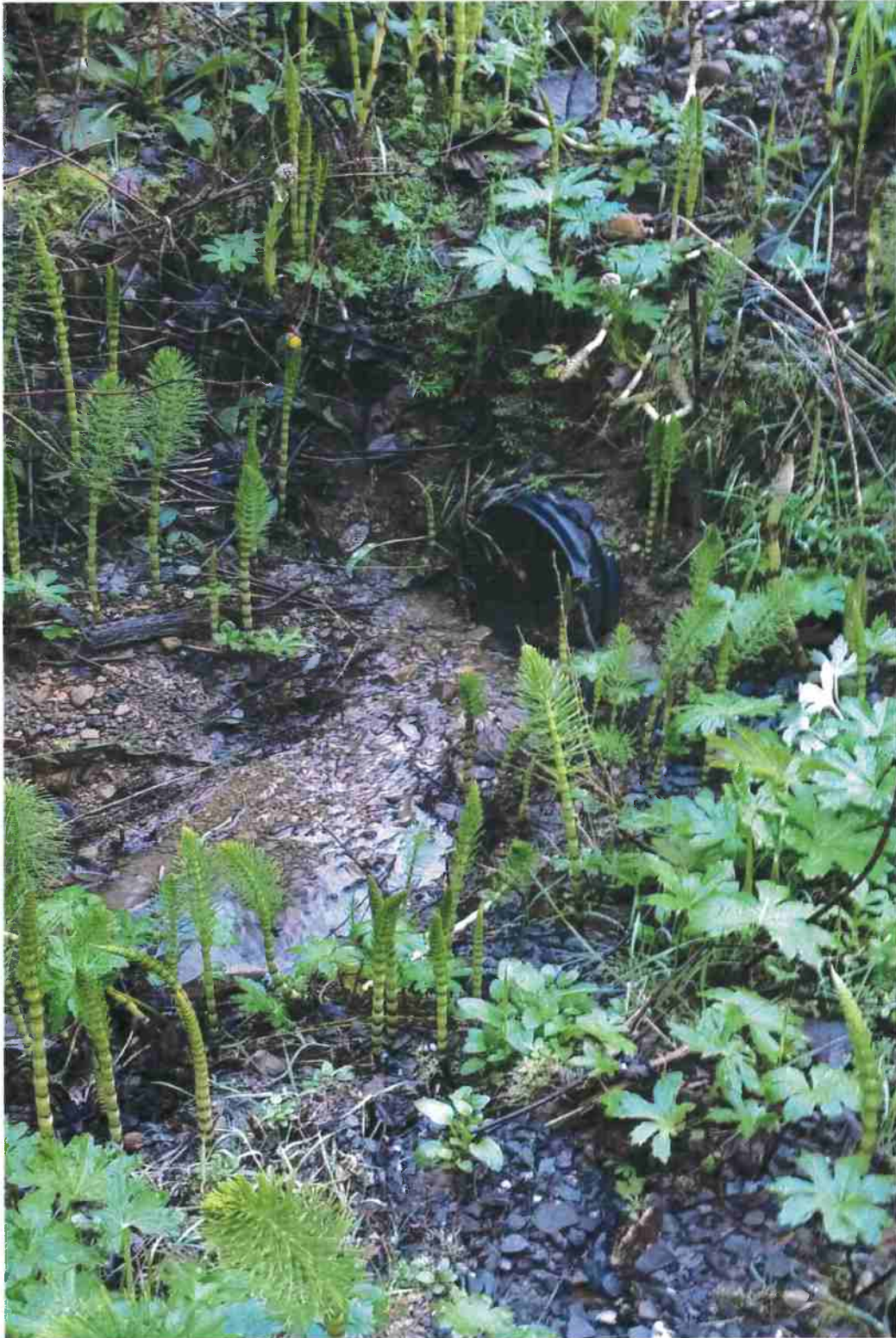
Figure 9. Outlet at 12" pipe at STX-1. Culvert will be replaced with a 24" diameter pipe.
