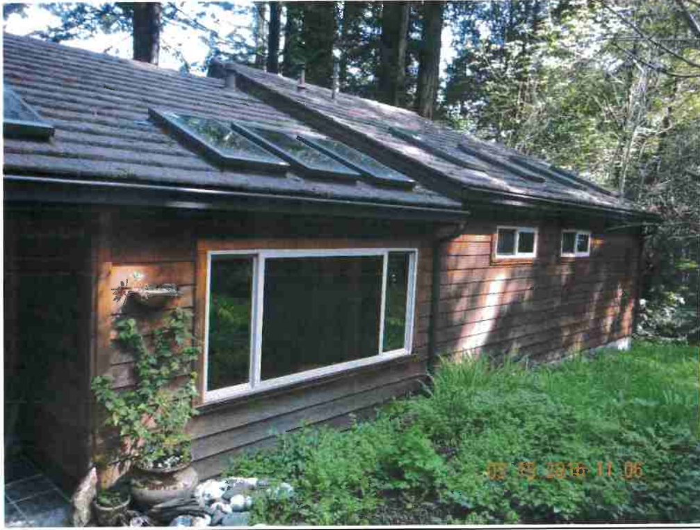
Figure 6. Single family residence
