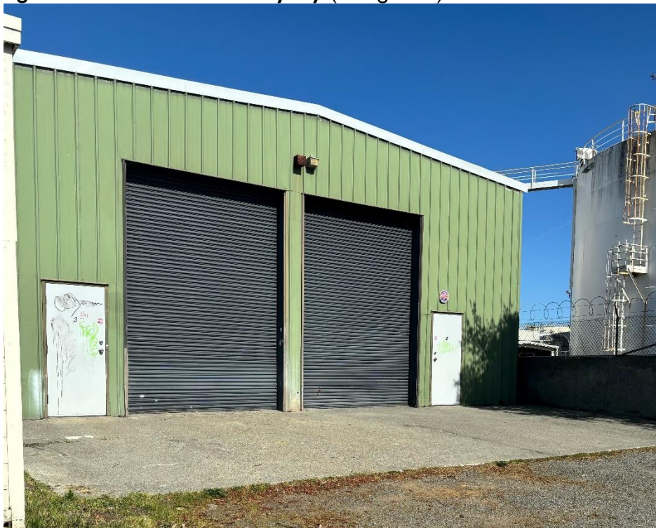
Figure 6: Street view from alleyway (facing west)
