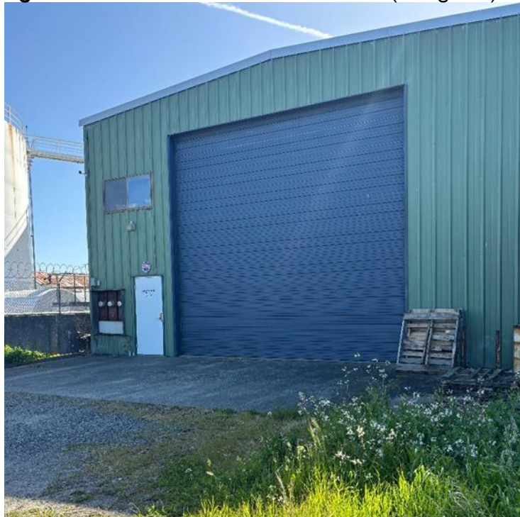
Figure 5: Street view from Christie Street (facing east)
