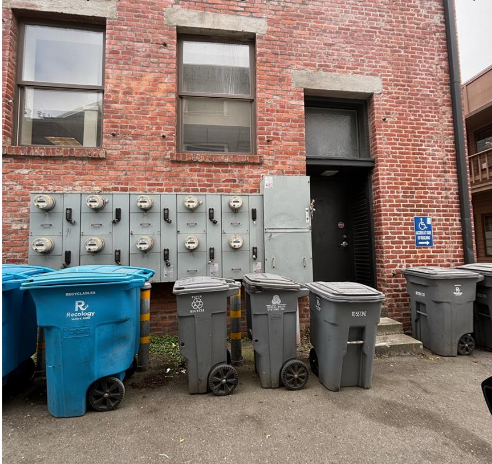
Photo 5: Alley-Adjacent North-Facing Windows and Door to Suite 103 (Summit Funding)
