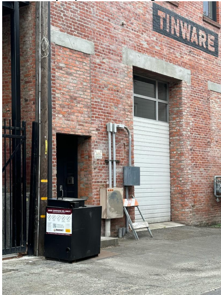
Photo 7: Alley-Adjacent North-Facing Doors to Suite 104 (Radiant Living storage)
