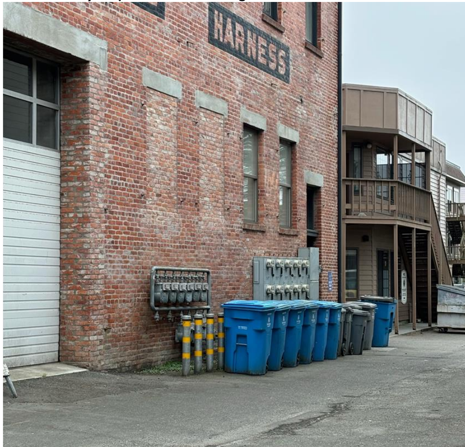
Photo 6: Alley-Adjacent North-Facing Windows and Doors
