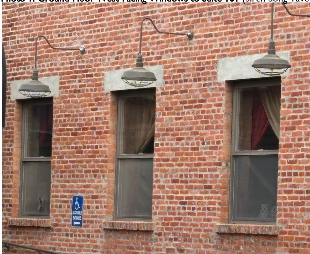
Photo 1: Ground-Floor West-Facing Windows to Suite 101 (Siren Song Tavern)
