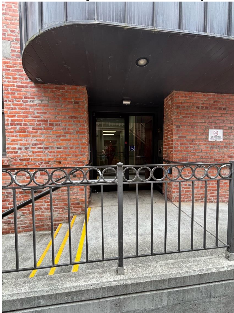
Photo 4: West-Facing Entrance to Shared Hallway
