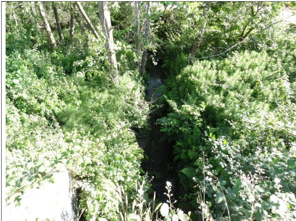
June 18, 2023. Wolverton Gulch at concrete box culvert and Hwy 36, looking south. (40.546012, - 124.115143).
