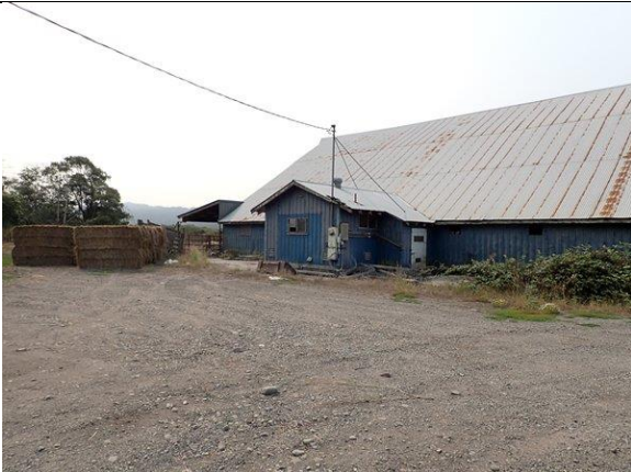
View of the north side of the barn on the Property
