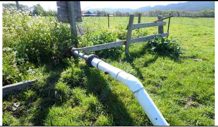
Additional view of water line connections
