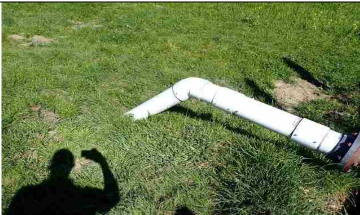
Additional view of water line connections
