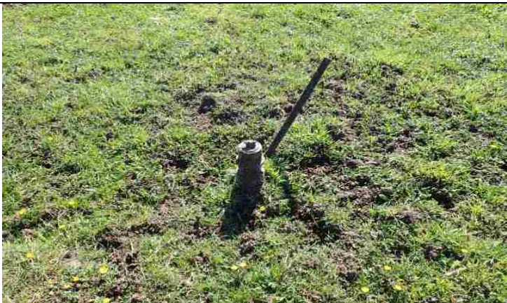
View of a sprinkler hookup on the Property
