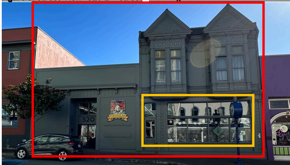
Figure 3: Street View- 520 2 nd Street – building outline red and storefront window area orange
