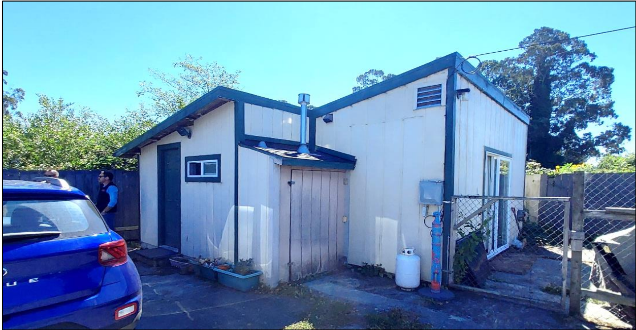
Figure 3: Current Photo of Unpermitted ADU (Looking towards the southeast)
