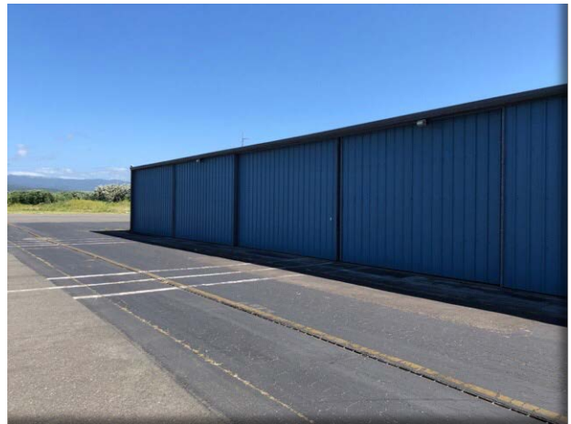
Small T-Hangar Nunno
